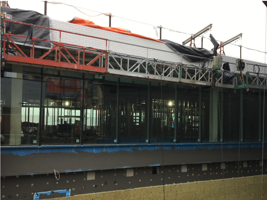
Brick installation on Bar 1
