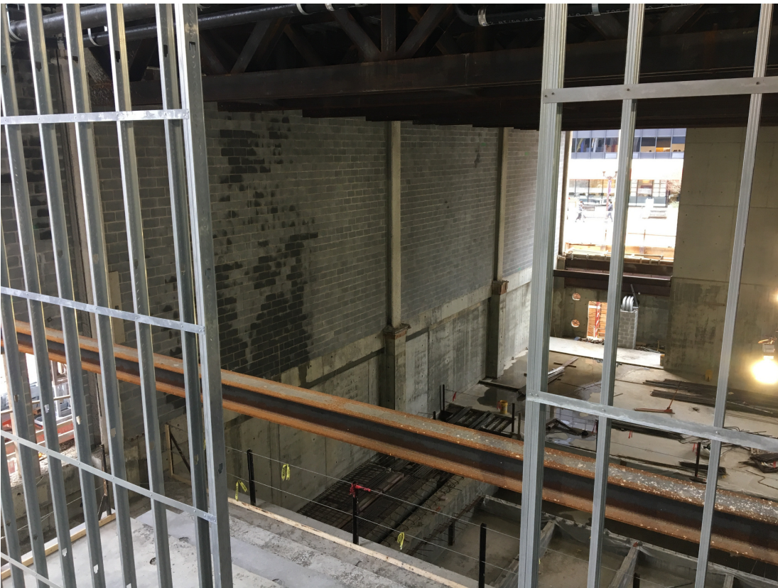
CMU wall completed on auditorium east wall
