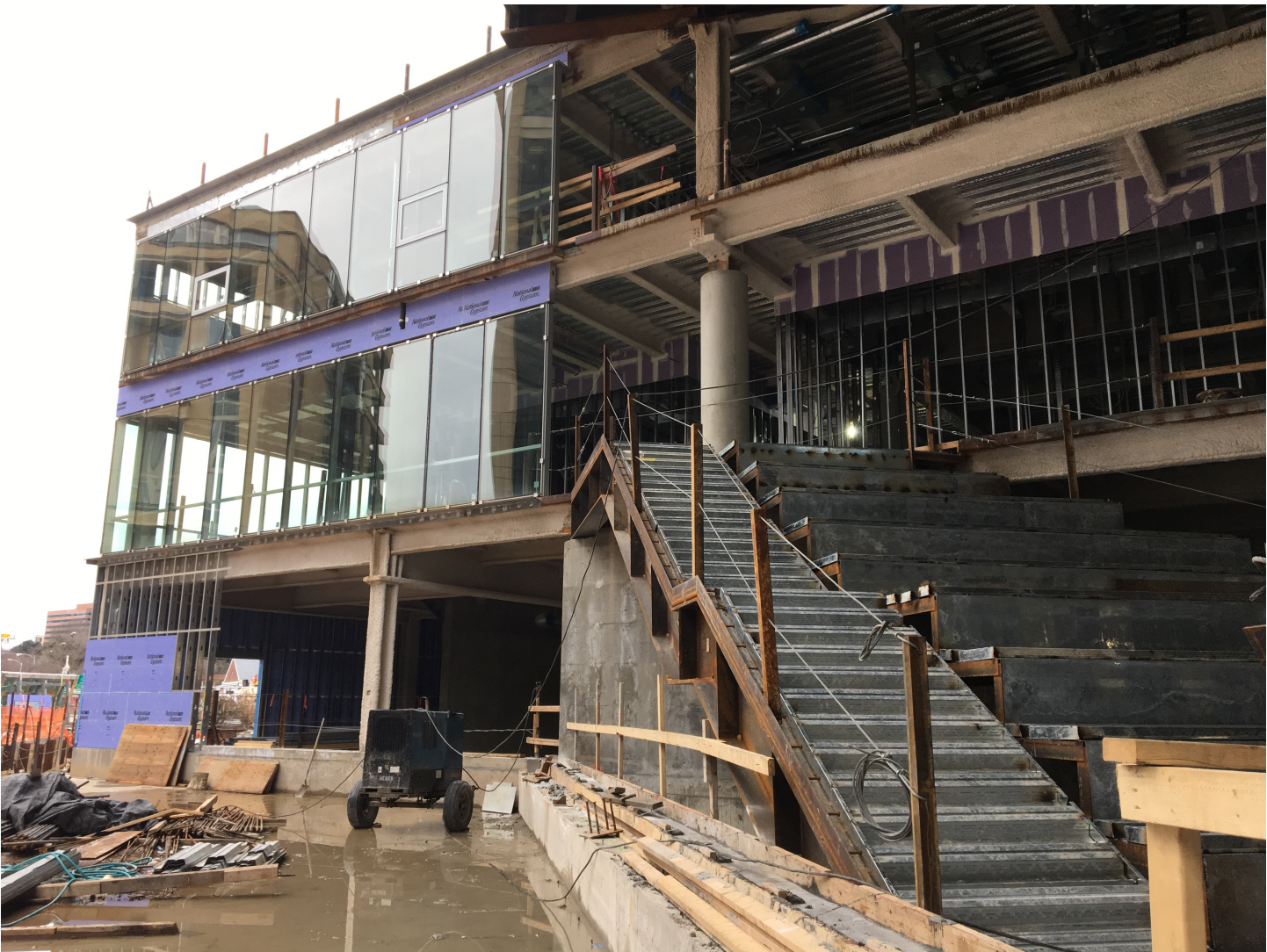
Curtainwall installation along Wilson Blvd
