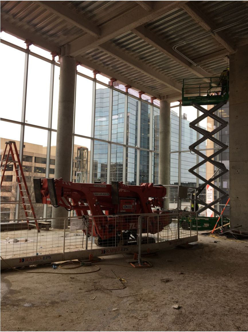
Curtain wall completed at music rooms
