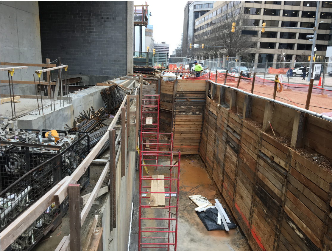
Electrical transformer vault wall and mat pad installation
