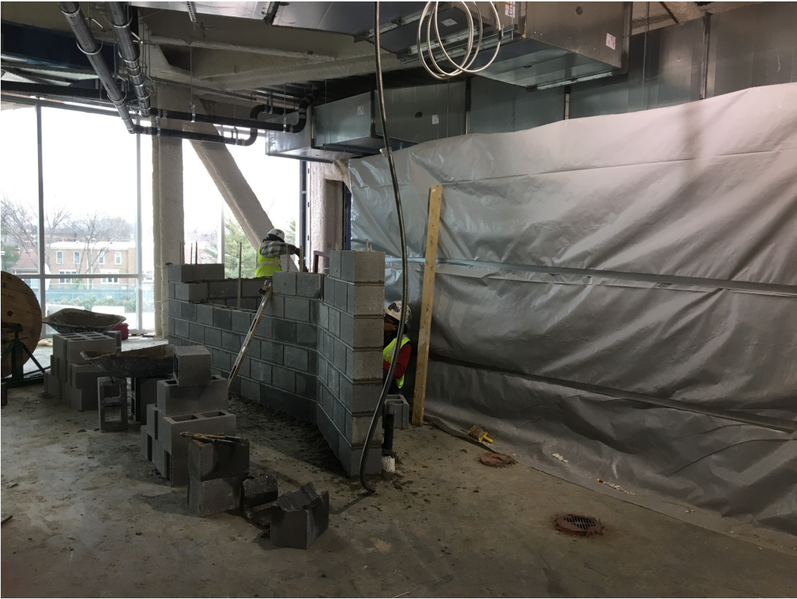
Air handling unit set and CMU wall installation
