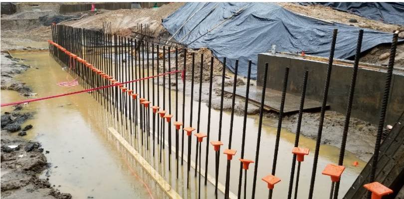
Foundations – 1 st floor
