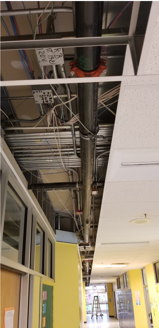
New Fire Suppression Main line
