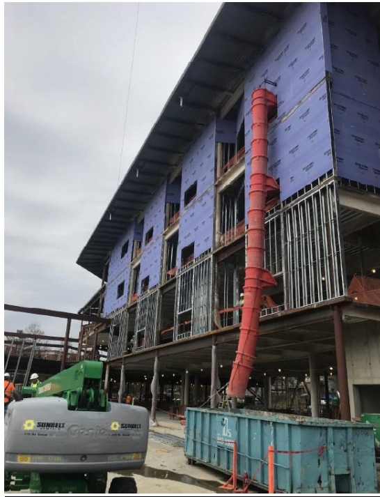
SHEATHING OF EXTERIOR WALLS
