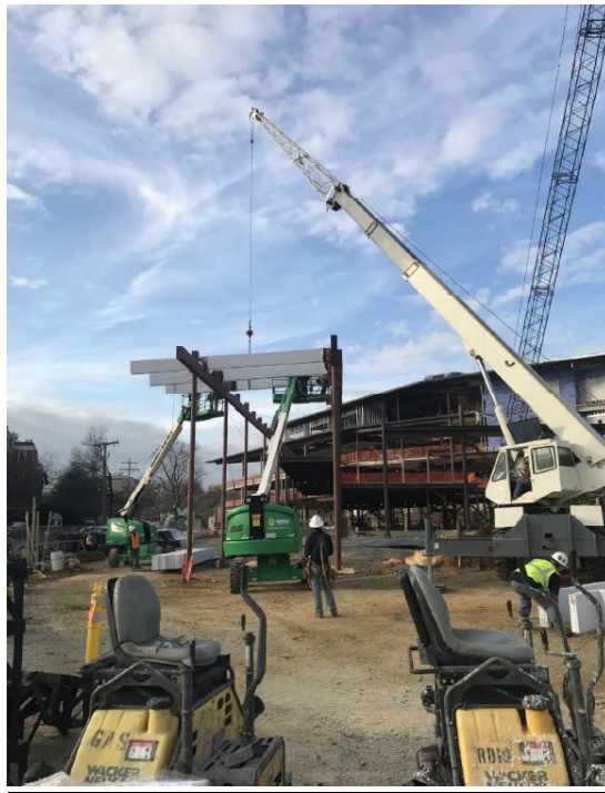
START OF STRUCTURAL WOOD ROOF INSTALLATION AT GYM
