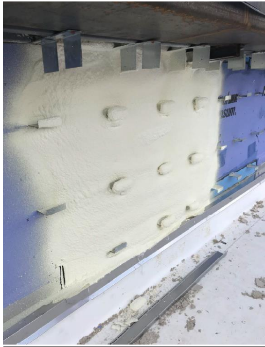
INSTALLATION OF SPRAY FOAM INSULATION/AIR & VAPOR BARRIER ON EXTERIOR SHEATHING
