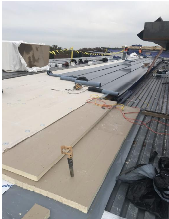
ROOFING UNDERLAYMENT INSTALLATION
