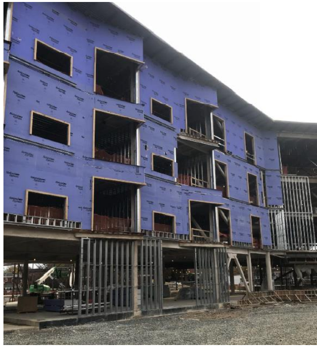
SHEATHING OF EXTERIOR WALLS
