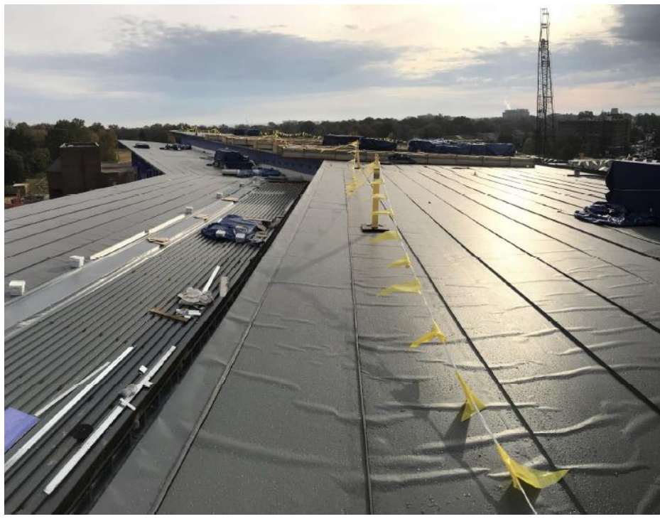
ROOFING UNDERLAYMENT INSTALLATION
