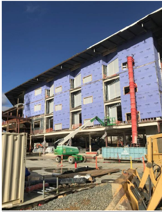
TEMPORARY CLOSE-IN OF WINDOWS
