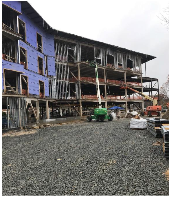
EXTERIOR WALL FRAMING
