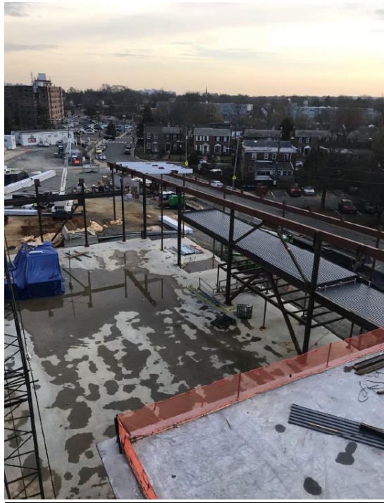
STRUCTURAL STEEL AT GYM READY FOR STRUCTURAL WOOD ROOF INSTALLATION
