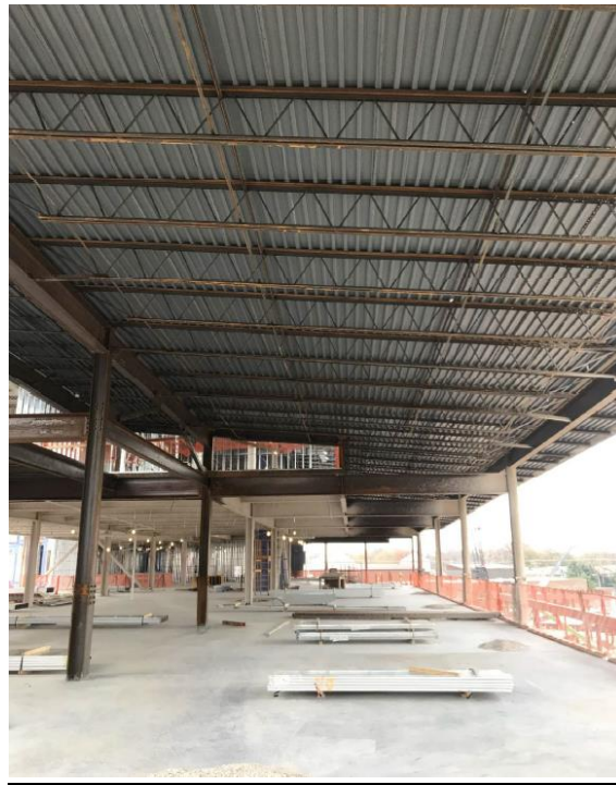
STRUCTURAL STEEL ERECTION COMPLETED AT 4-STORY SECTION OF BUILDING
