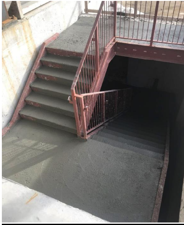
GARAGE STAIRS POURED
