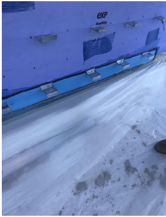
INSTALLATION OF CLIPS FOR ATTACHMENT OF EXTERIOR FAÇADE CLADDING
