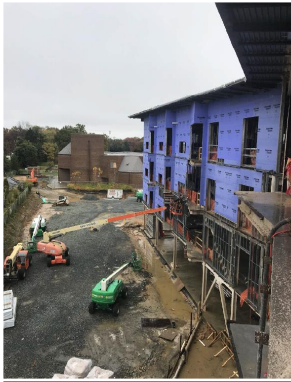
SHEATHING OF EXTERIOR WALLS
