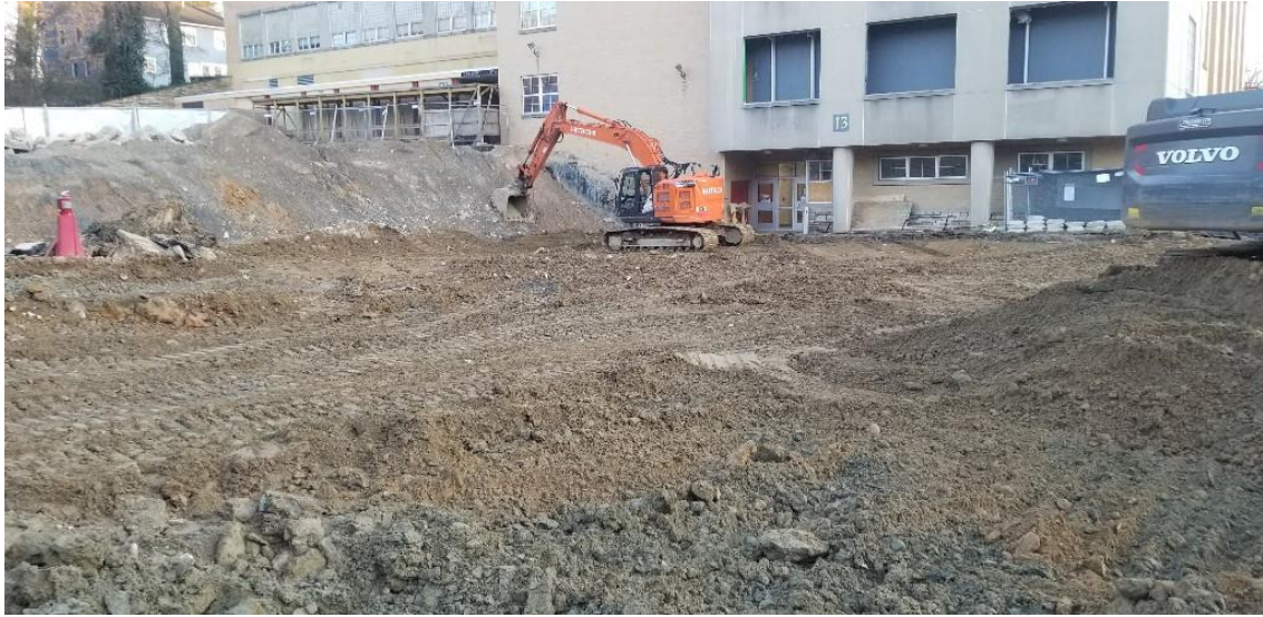
Building Pad preparation
