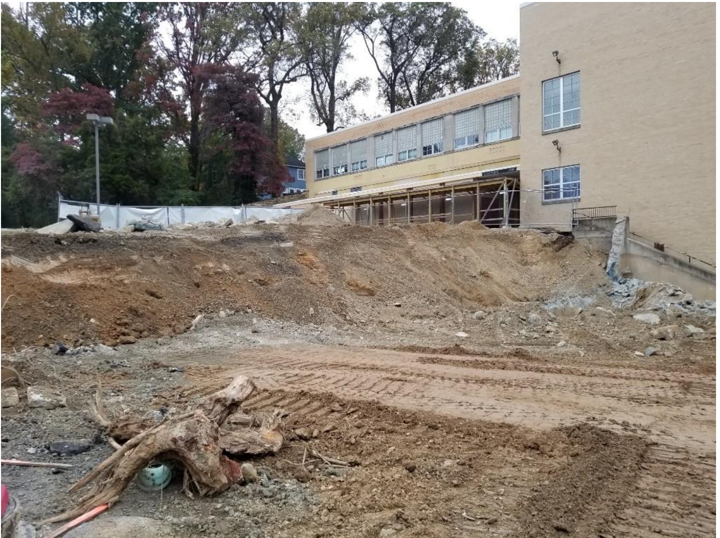
Demolition of existing retaining wall / parking lot
