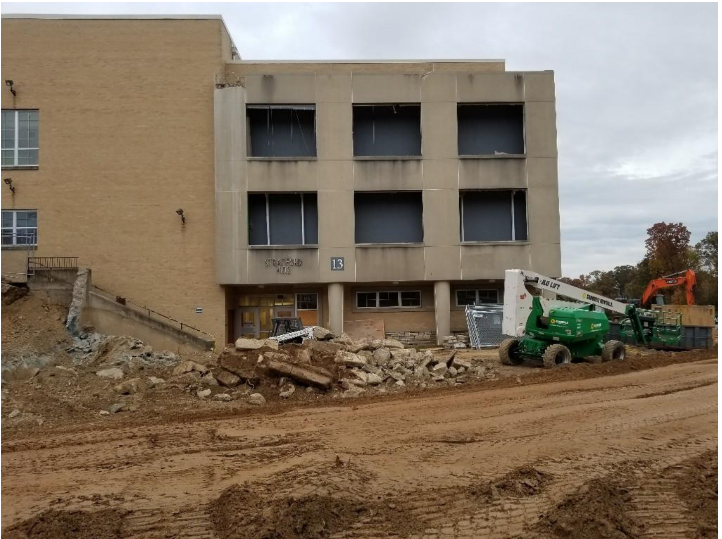
Stratford Entrance Pre-Cast and window demolition
