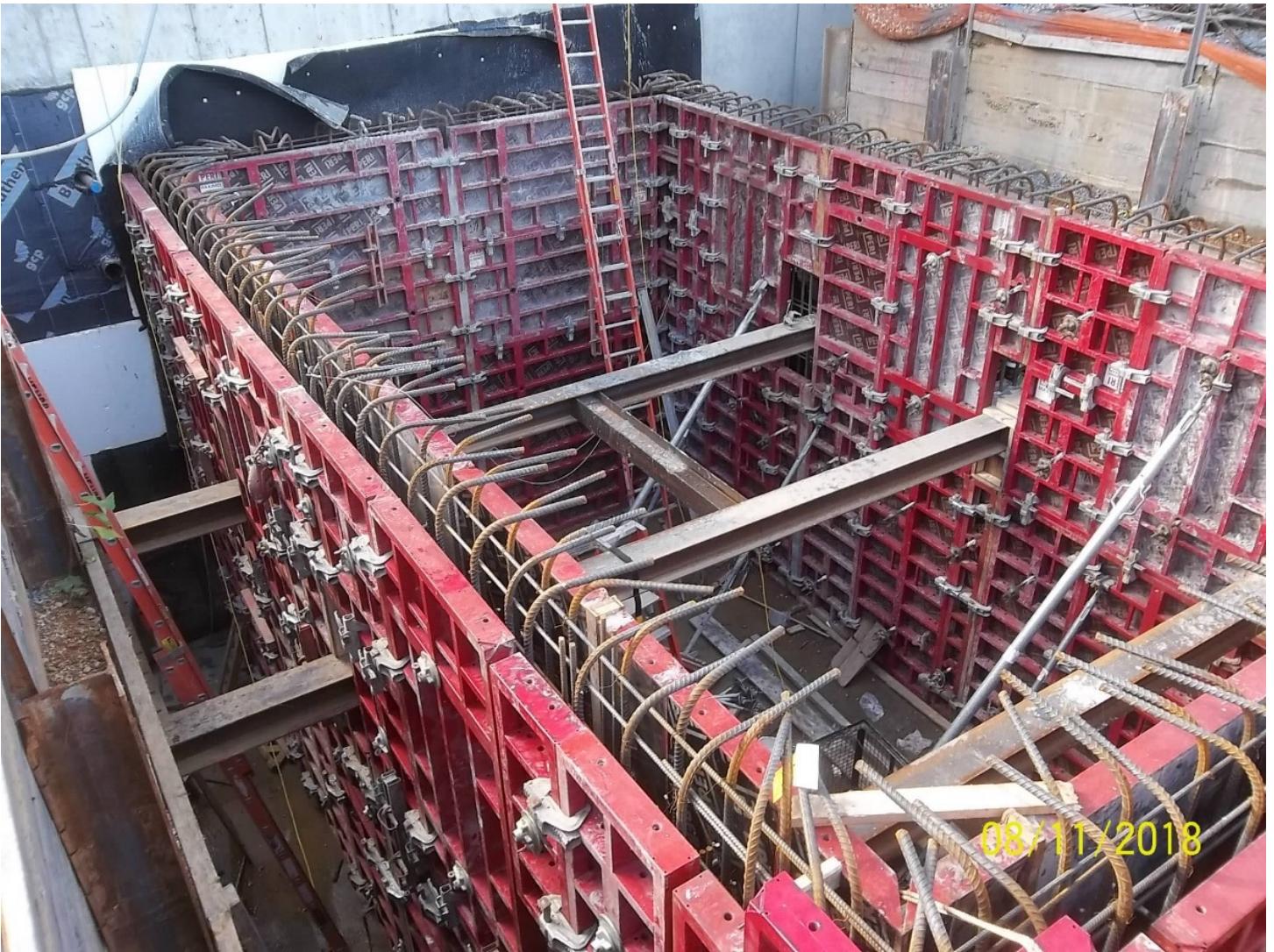
Wall forms for the cistern
