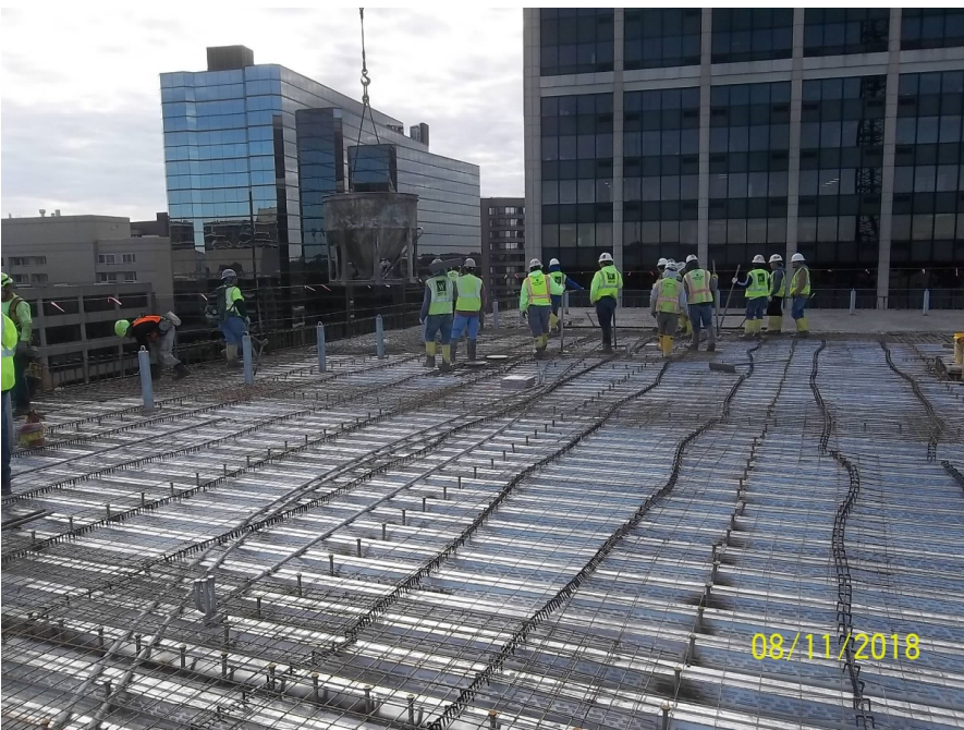
Pouring concrete deck at the roof level
