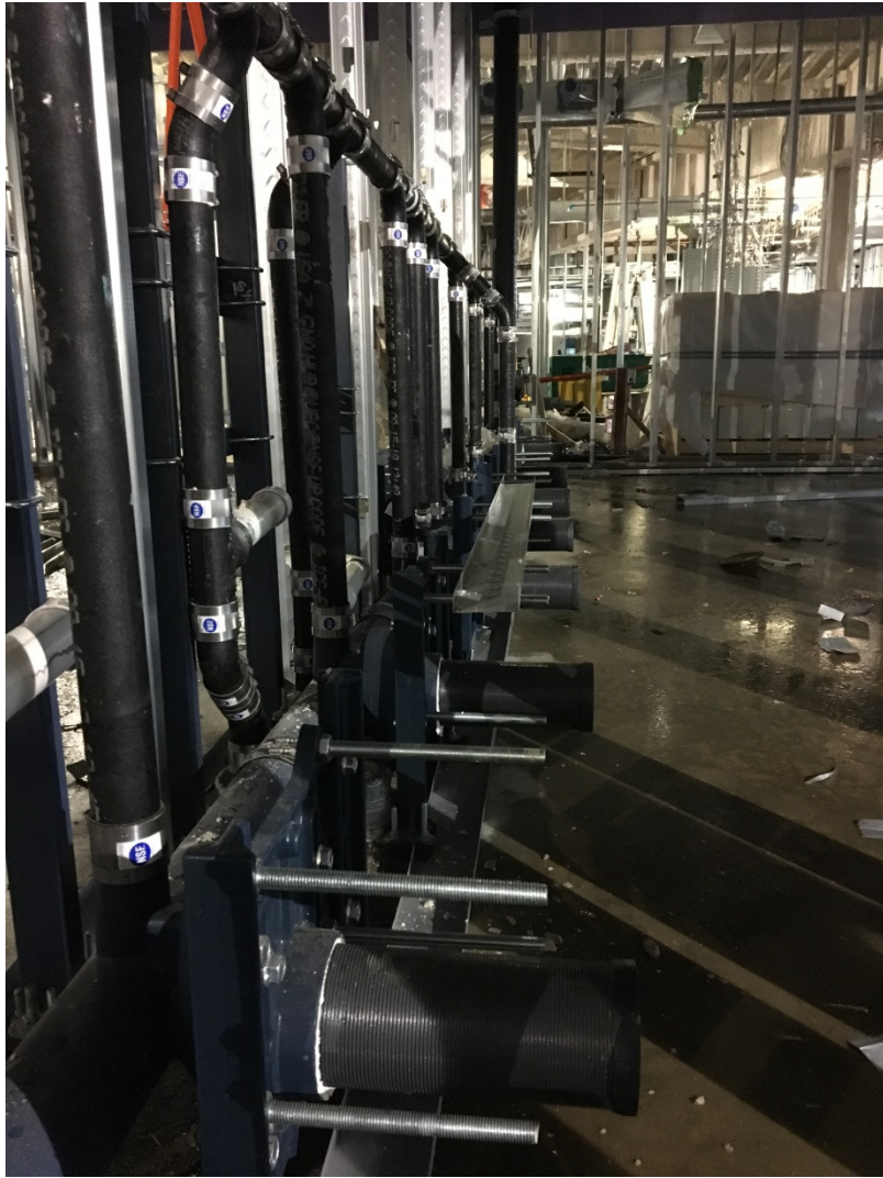
Plumbing pipe work at L1 level
