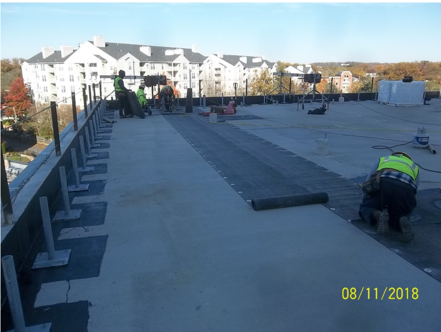
Roof installation at Bar 3 Terrace
