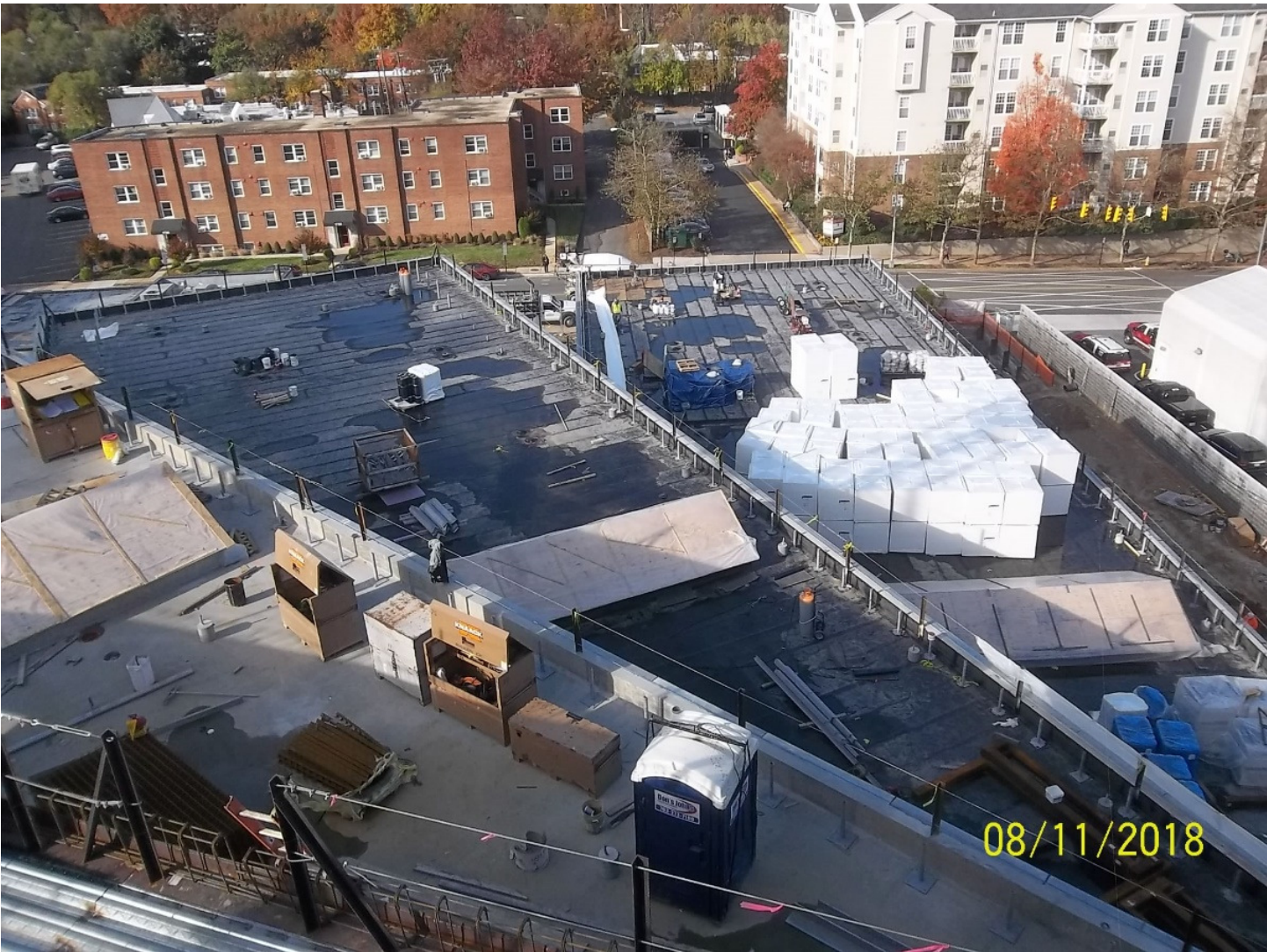
Roofing at Bar 1 & Bar 2 Terraces
