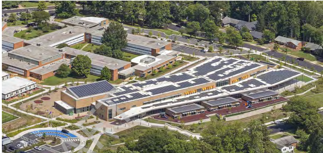
Discovery's environmental and sustainability design features make it the first Net Zero energy school in the Mid-Atlantic Region, and only the third in the United States. The rooftop solar lab, as illustrated, is accessible to students, who can utilize it to conduct real-time and on-going experiences. Data and information from these experiences are tracked and graphed using the building's dashboard system.
