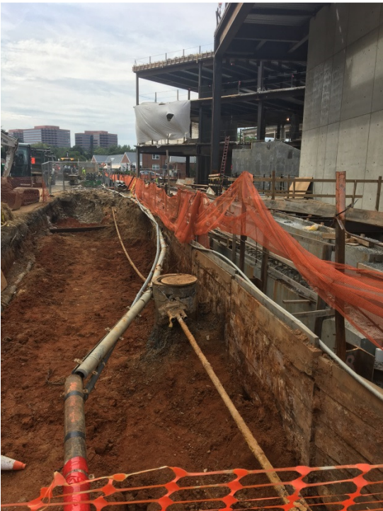
Excavation for DVP vault
