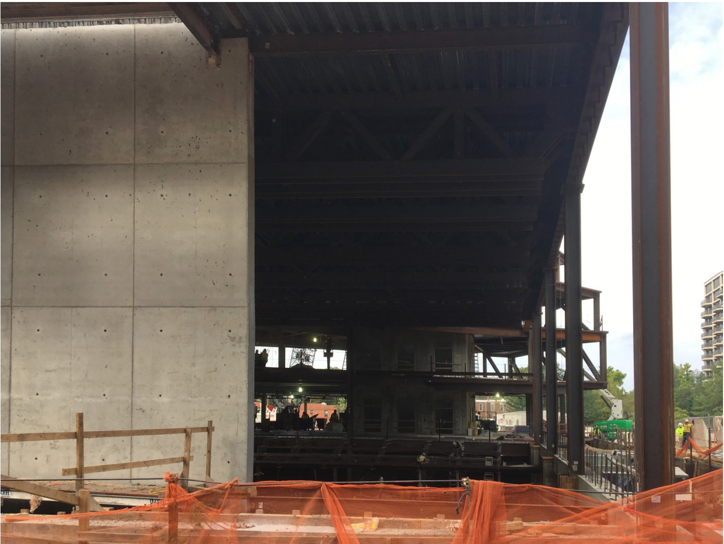
Steel trusses at theater erected
