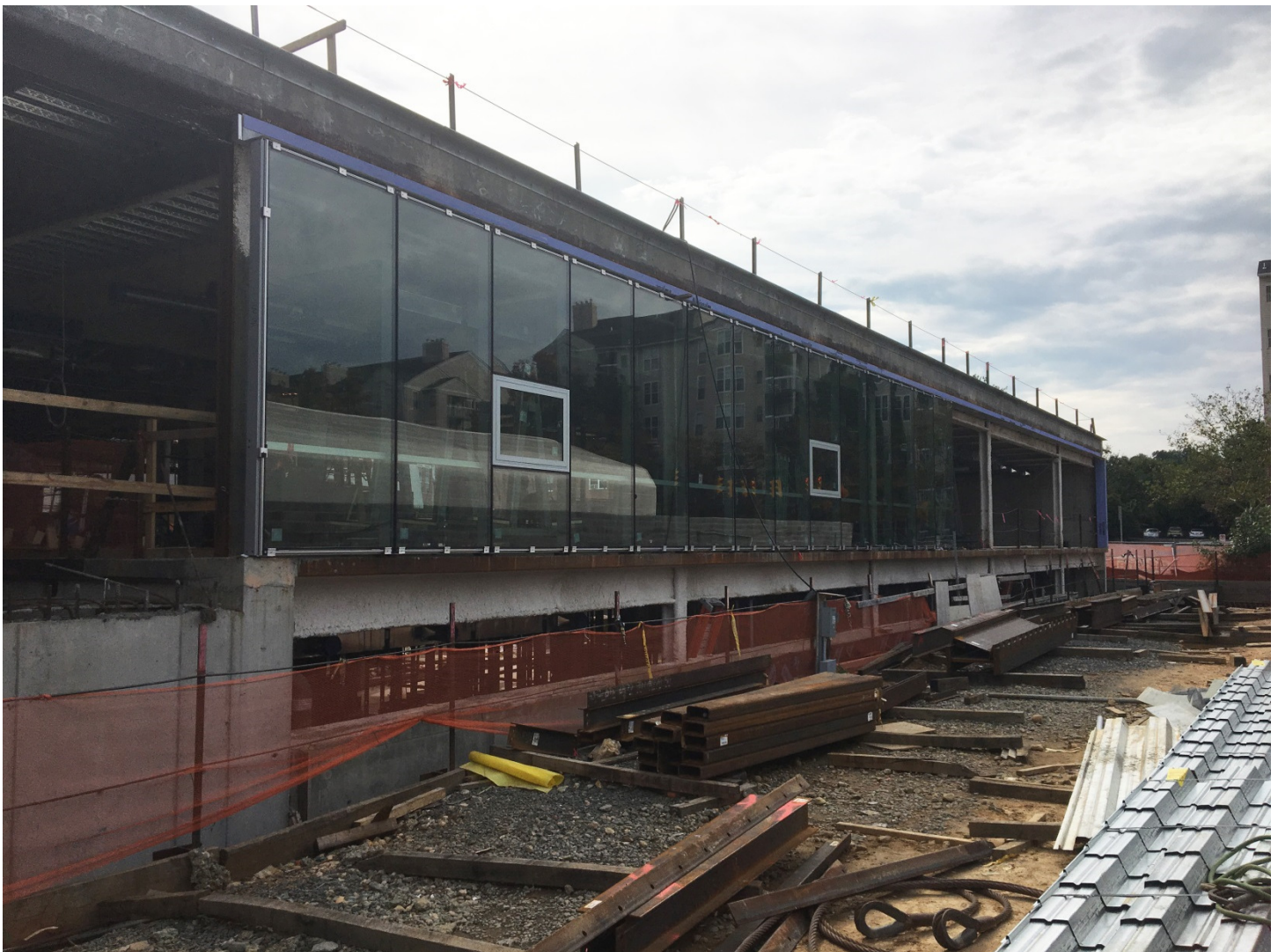
Curtainwall installation
