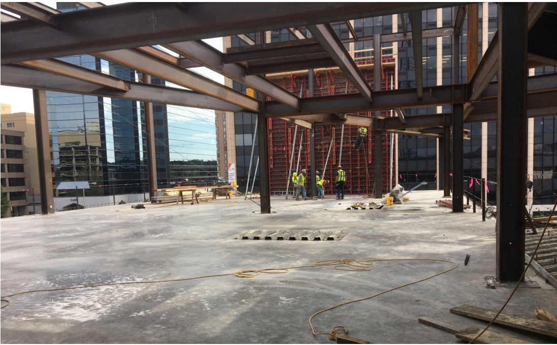
Level 3 music room slab
