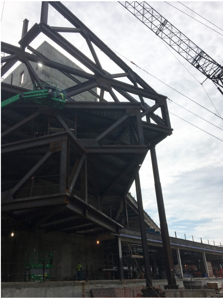
Bar 5 steel frame installation
