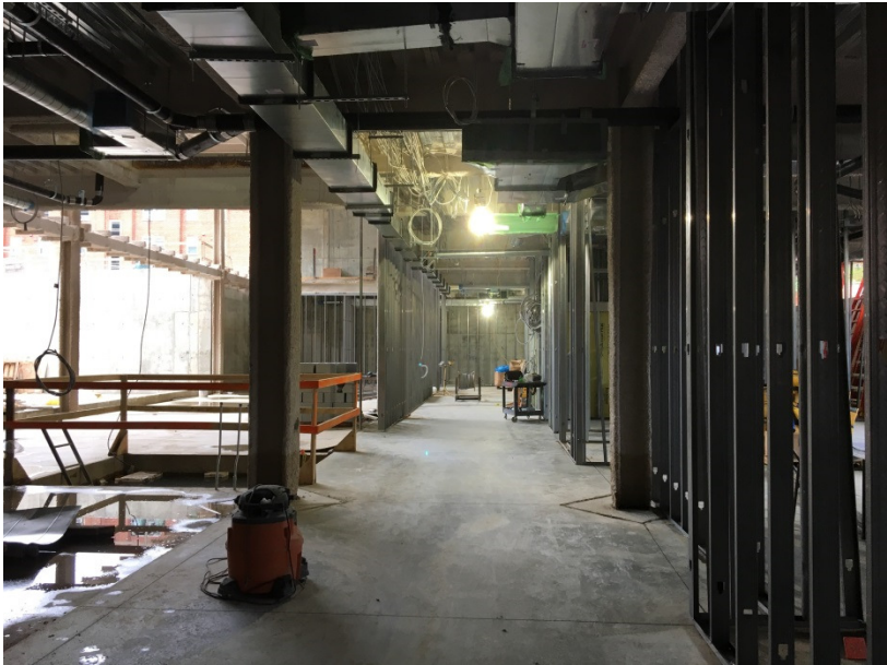
Framing and duct/pipe work at G1 level
