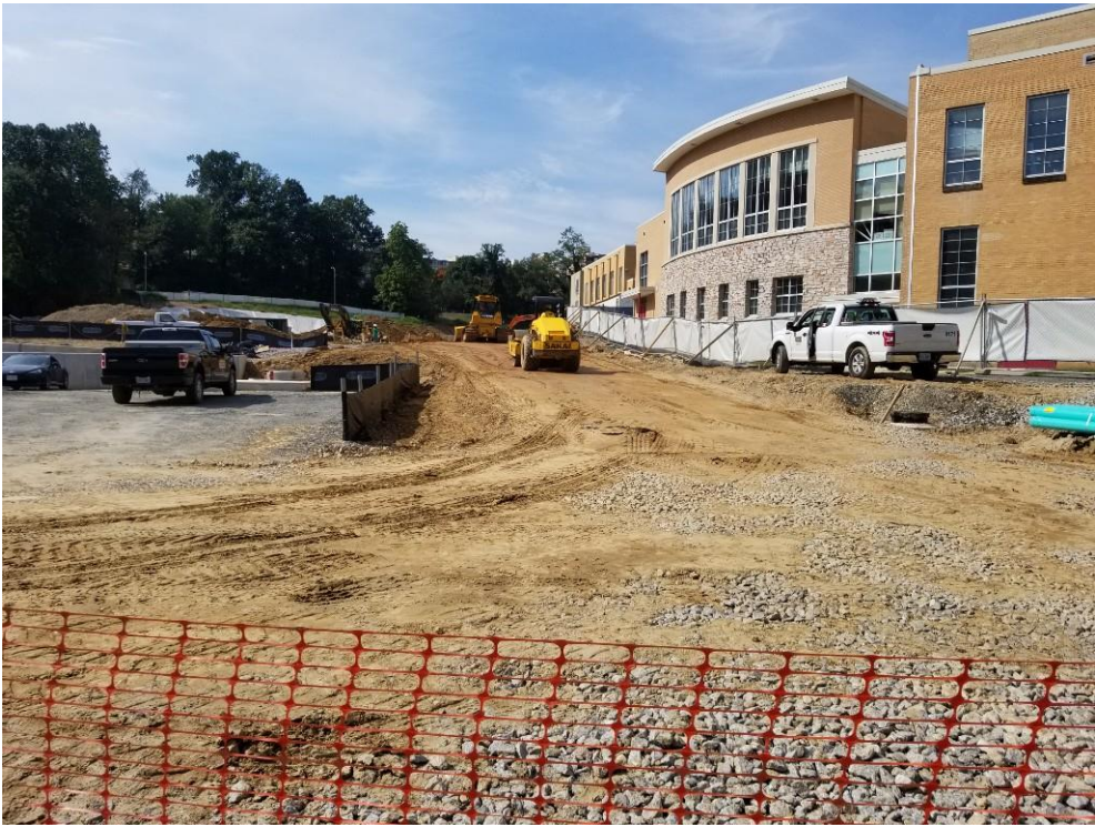
Backfill & Grading Operation for New Drop-Off Lane
