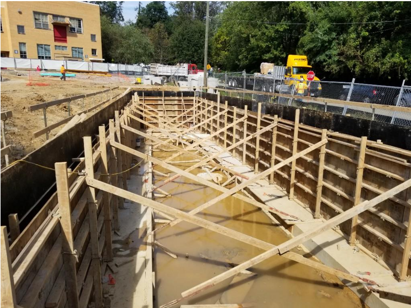
Bio Retention No. 9
