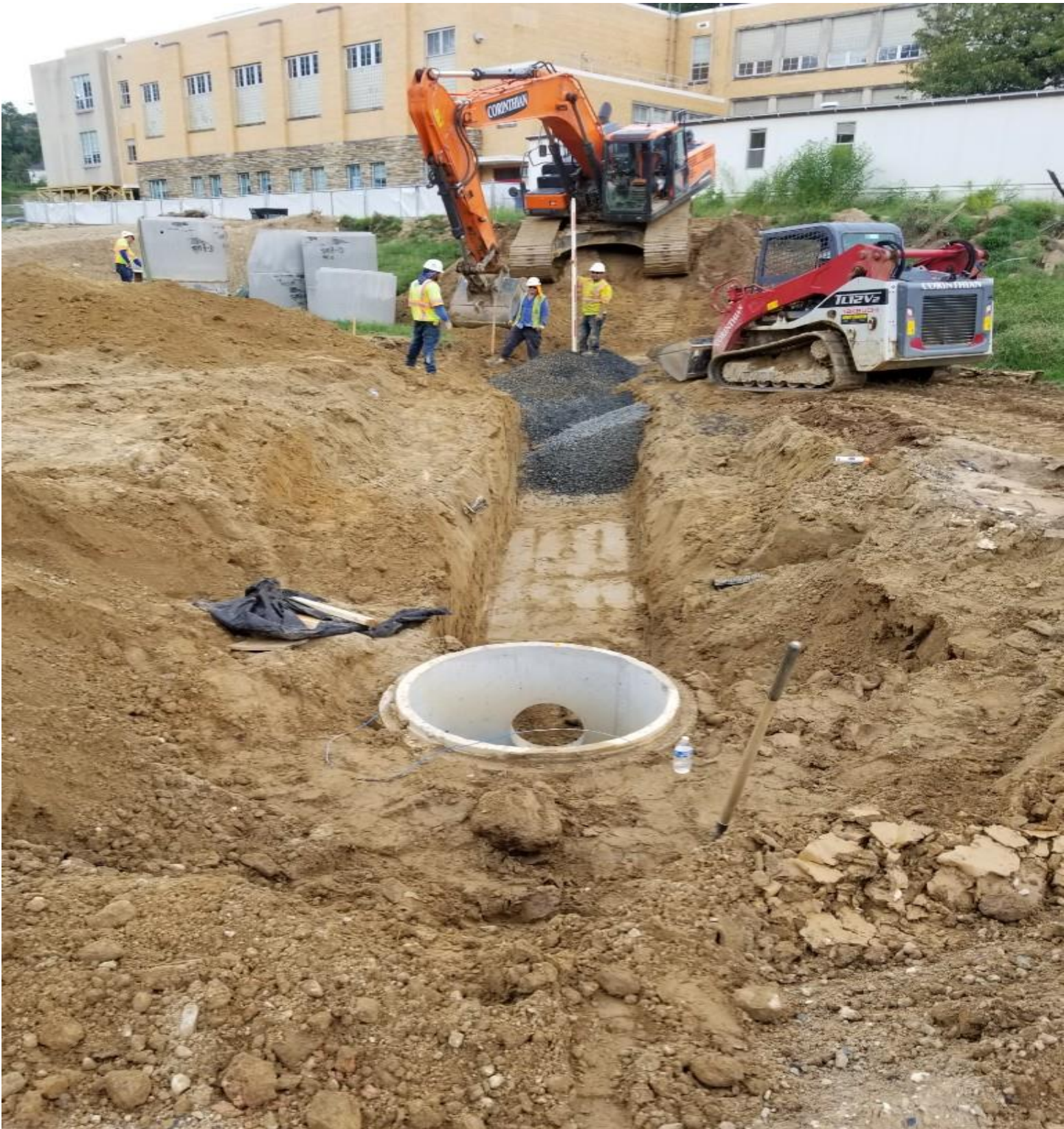
New underground Storm water piping in the field
