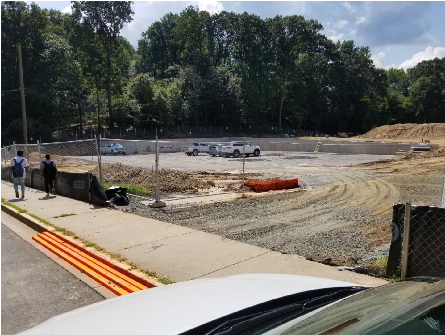
Partially complete New Employee Parking Lot
