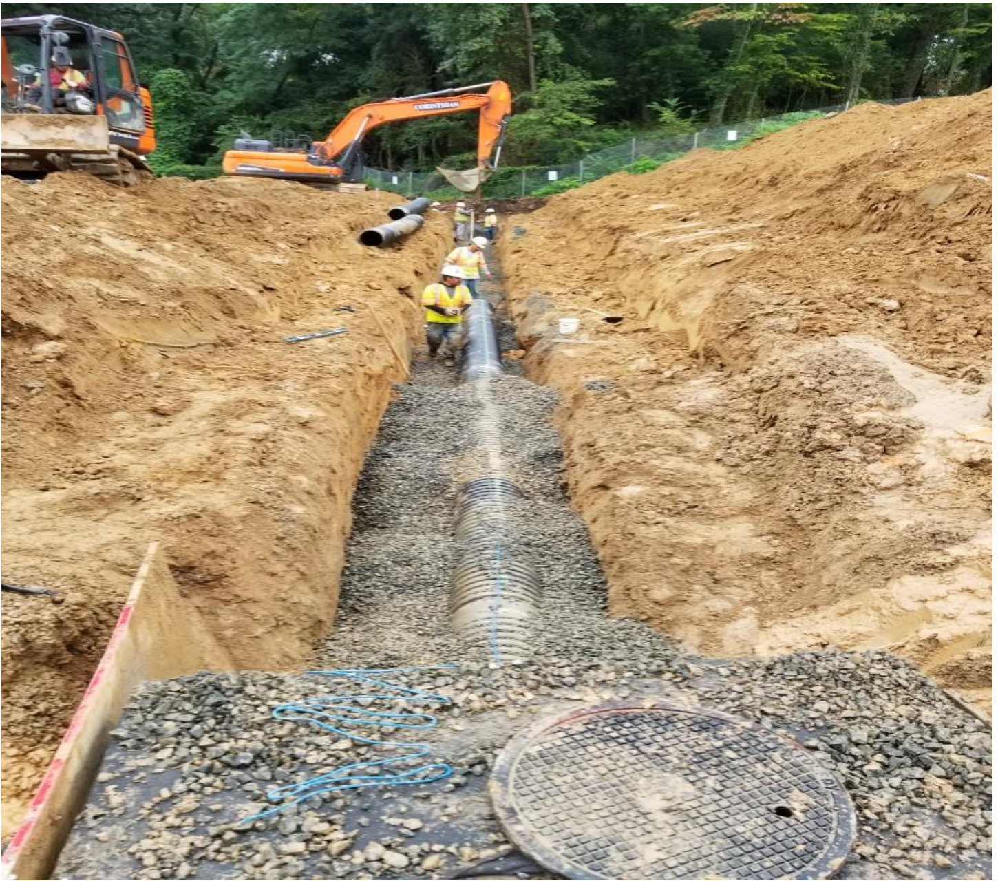
New underground Storm water piping in the field
