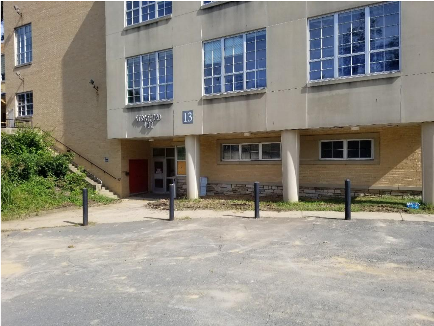
Partial Demolition of Stratford Entrance
