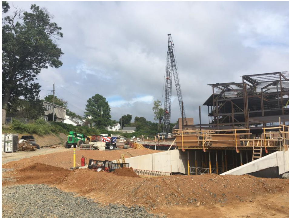
INSTALLED GARAGE ENTRY RAMP CONCRETE RETAINING WALLS
