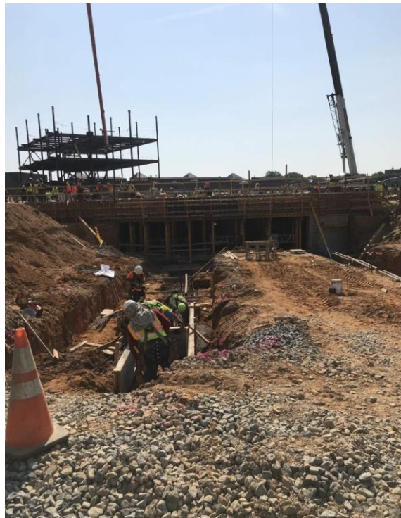
FOOTING INSTALLATION FOR GARAGE ENTRY RAMP RETAINING WALLS
