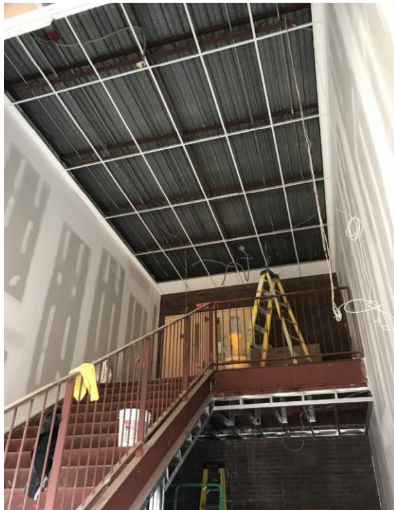
INTERIOR OF RECONFIGURED TJMS STAIRWELL
