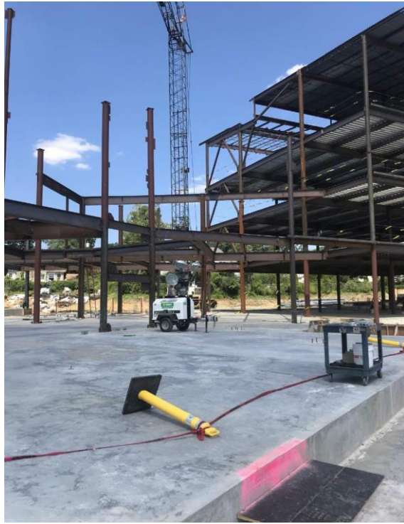
STEEL ERECTION STARTING ON 2 ND 4-STORY SEQUENCE
