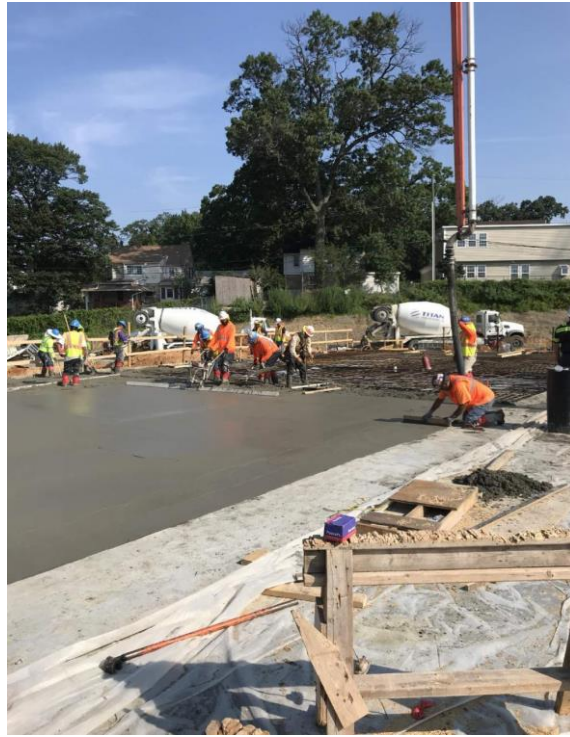
LAST CONCRETE SLAB POUR AT GROUND FLOOR LEVEL DECK
