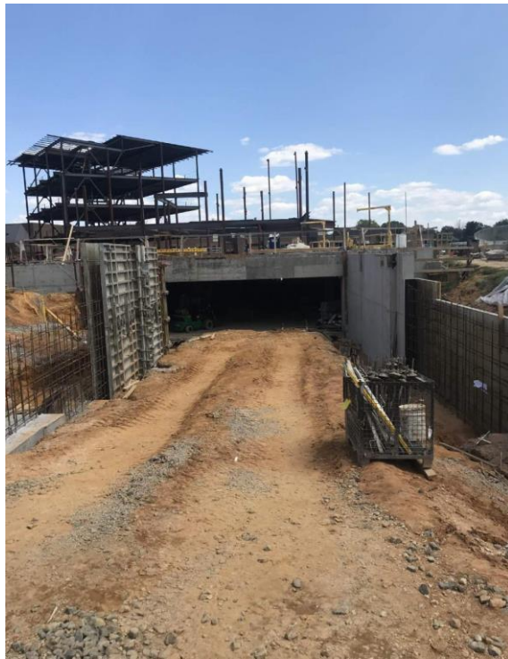
INSTALLATION OF FORMWORK FOR GARAGE ENTRY RAMP RETAINING WALLS
