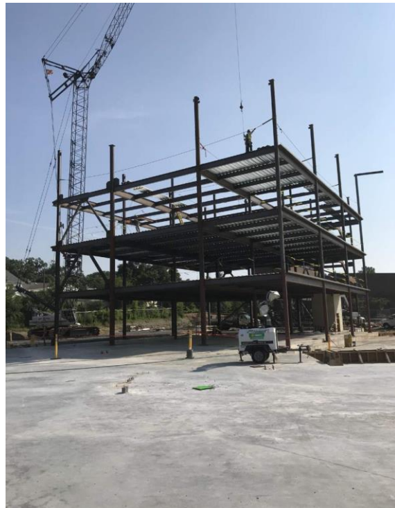
FRAMING OF 4TH FLOOR STEEL DECK
