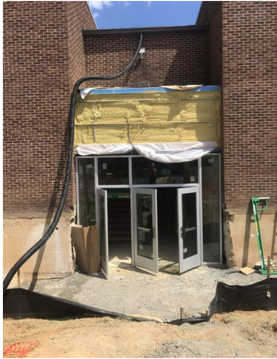
EXTERIOR OF STAIRWELL WITH NEW ENTRY DOORS IN PLACE
