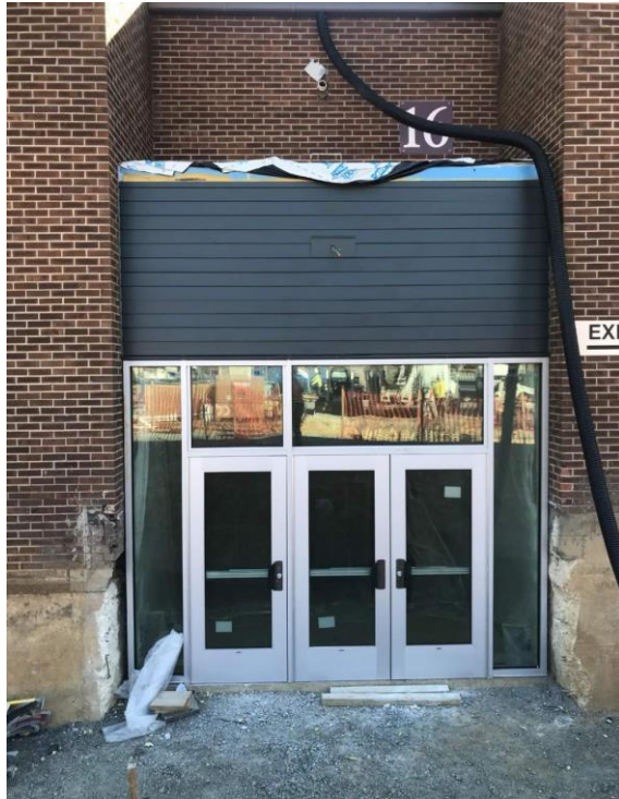
EXTERIOR OF STAIRWELL WITH SIDING IN PLACE, READY FOR ROOFING
