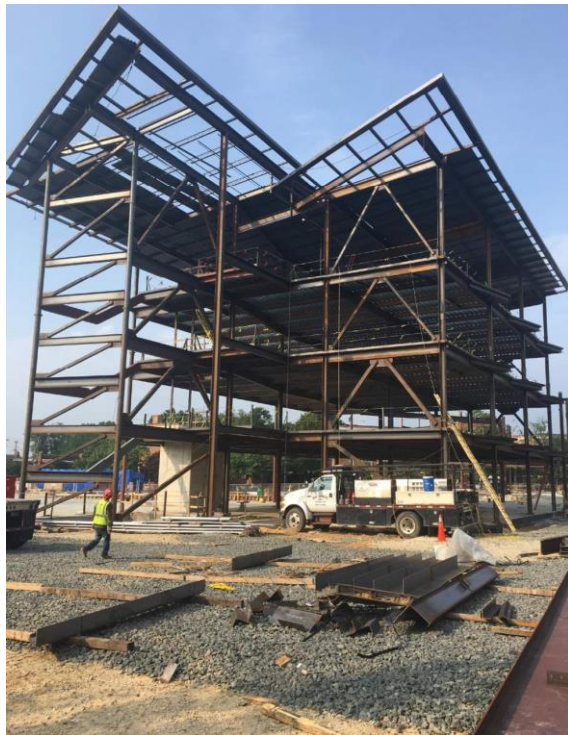
PROGRESSION OF STEEL FRAMING AND LATERAL BRACING FOR 1 ST ERECTION SEQUENCE
