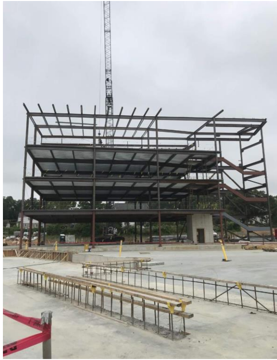
FRAMING OF ROOF STEEL
