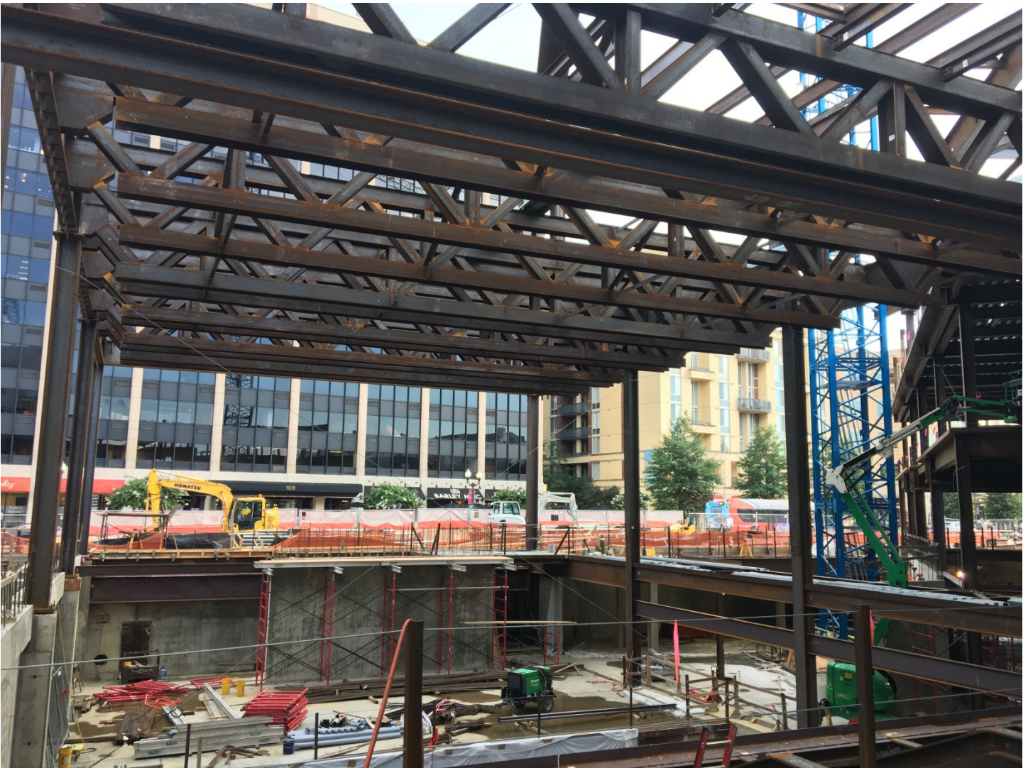
Steel trusses at theater erected
