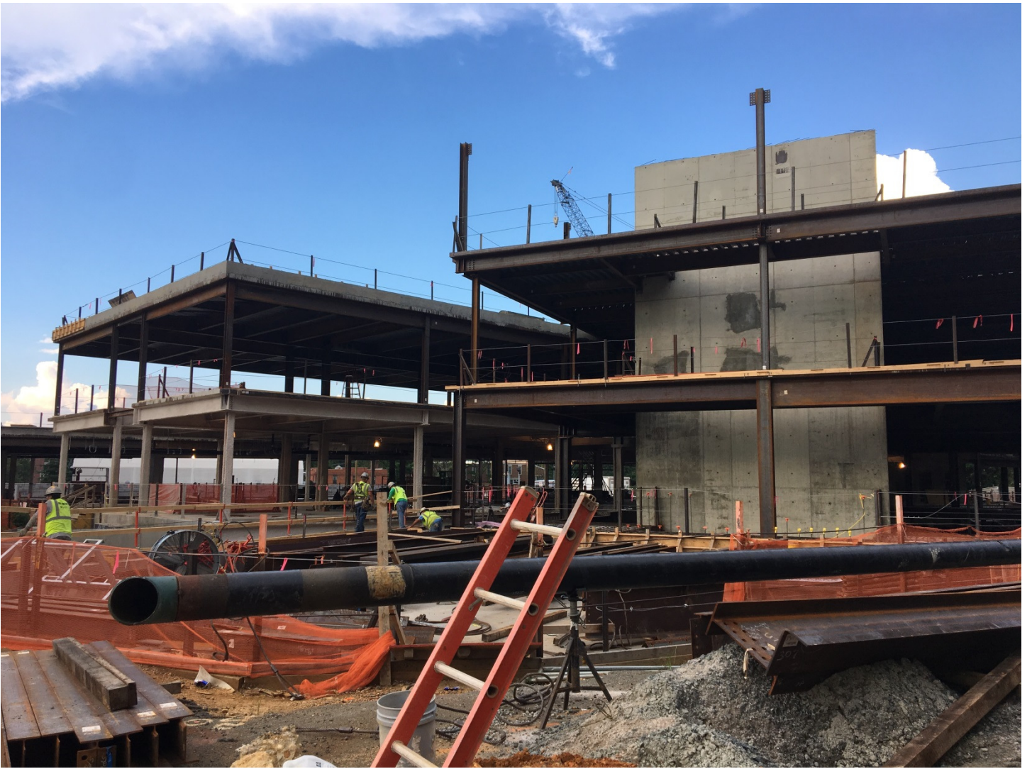
Exterior view from Wilson Blvd
