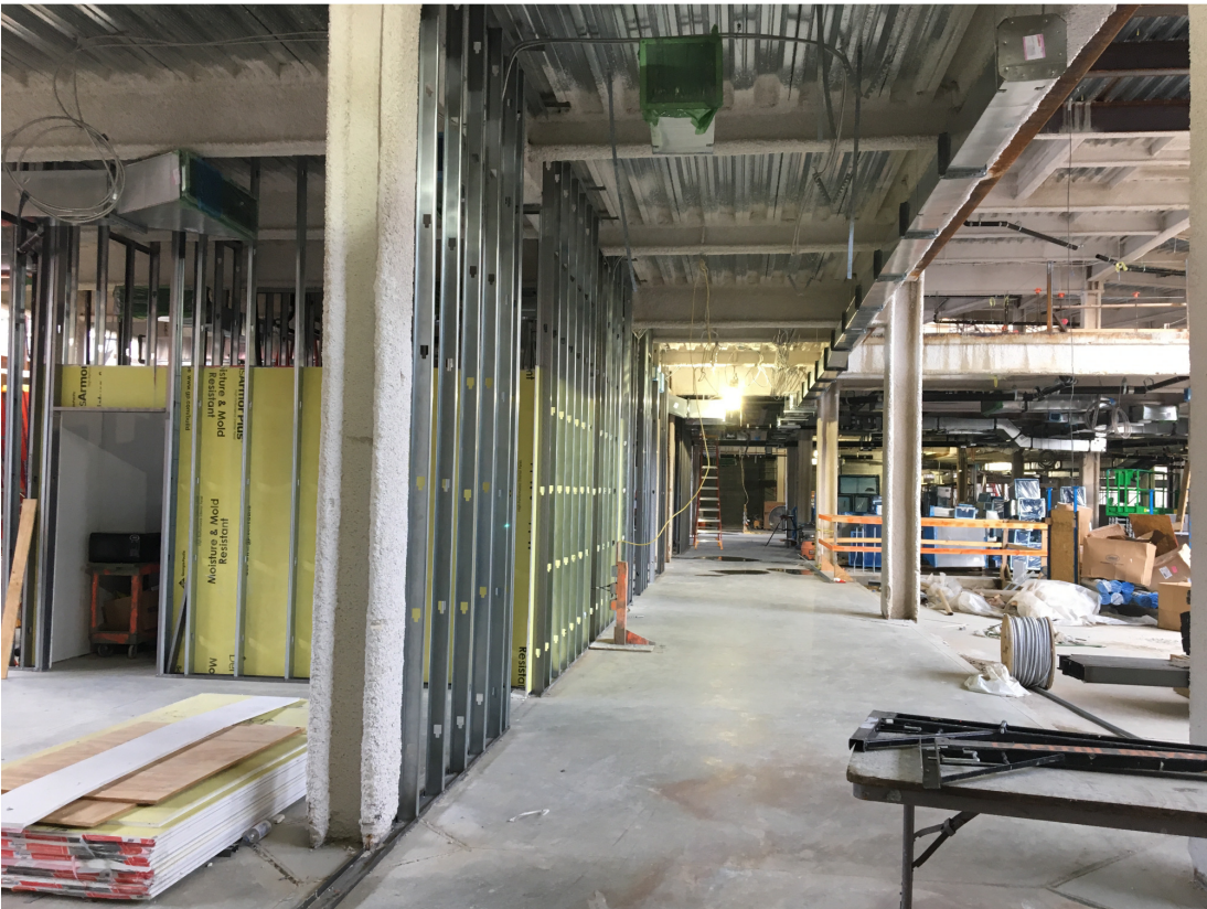
Interior wall framing at G1
