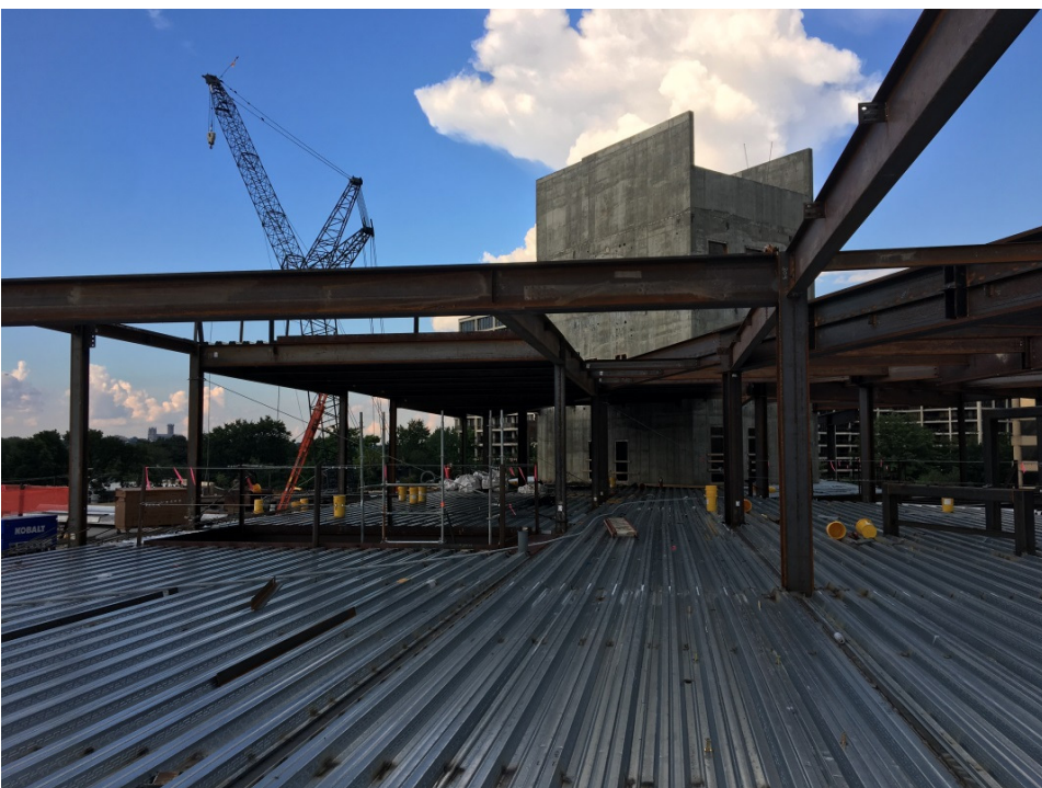
Bar 3 steel deck preparation
