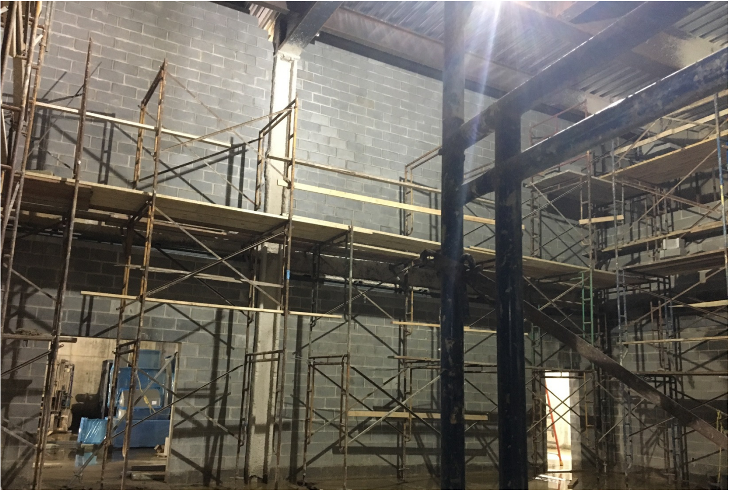
CMU walls at black box
