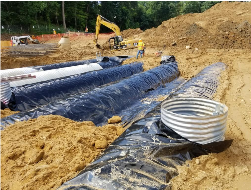
Future underground 72" Storm water detention system
