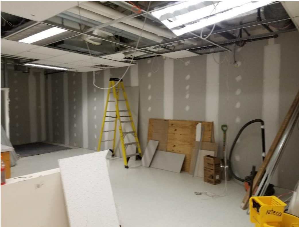
Temporary construction partition walls in Room 117
