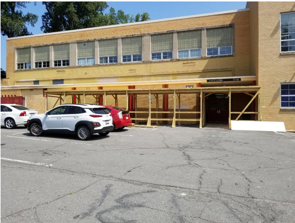
Temporary overhead walkway protection from Door 14
