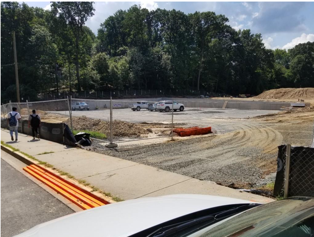
New Employee Parking Lot (temporary pavement)
