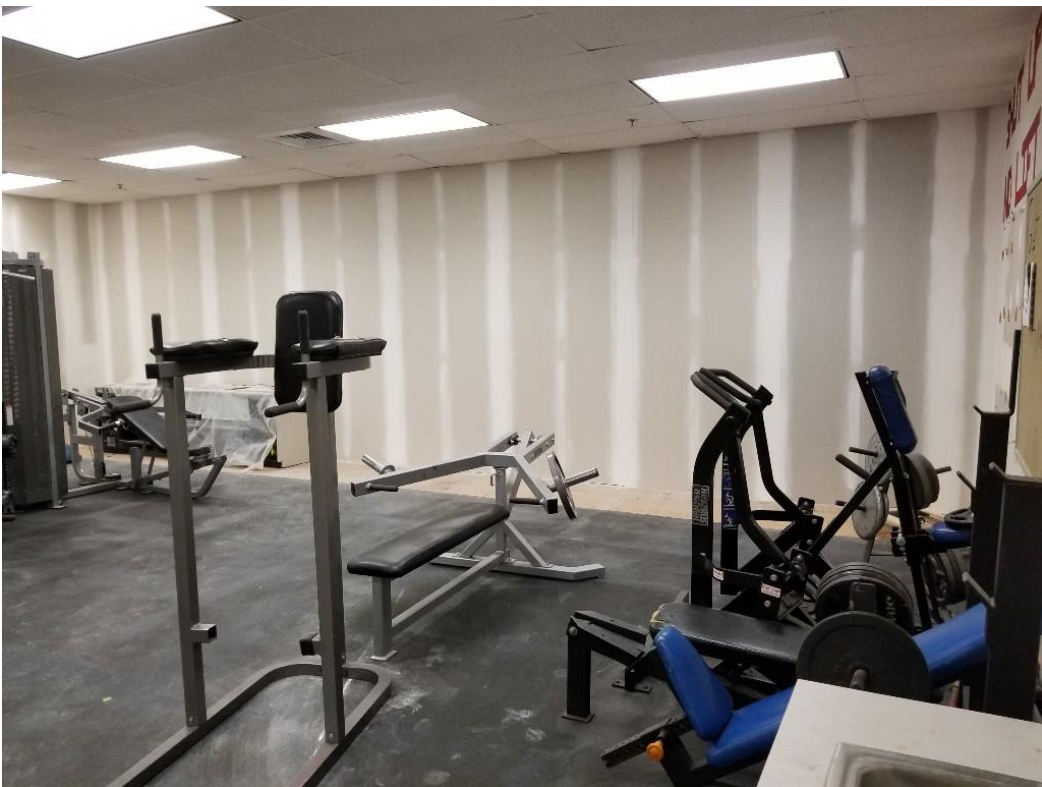
Temporary construction partition walls in Weight Room
