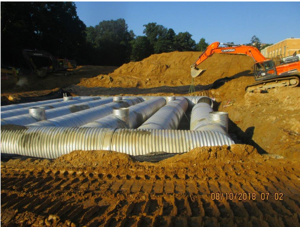
Future underground 72" Storm water detention system
