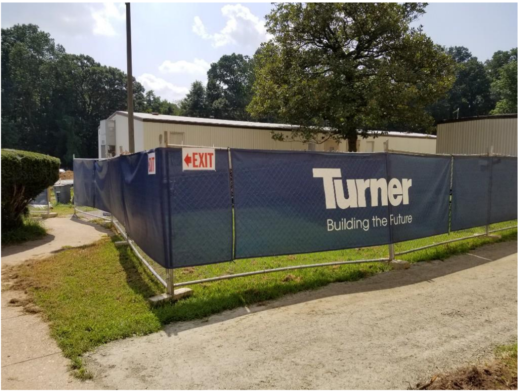
Temporary emergency egress walkway screening
