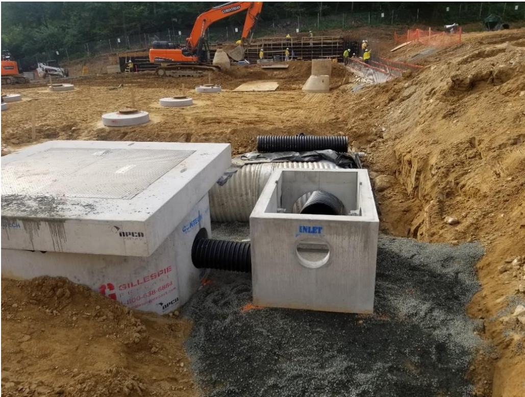
Future underground Storm water filtration system
