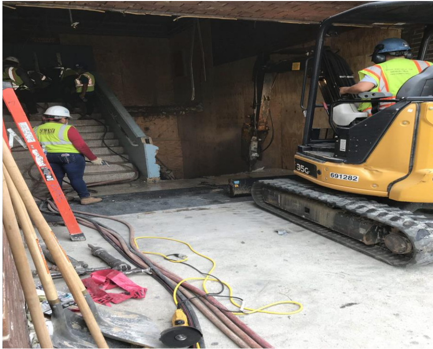
DEMOLITION OF JEFFERSON MIDDLE SCHOOL STAIRWELLS
