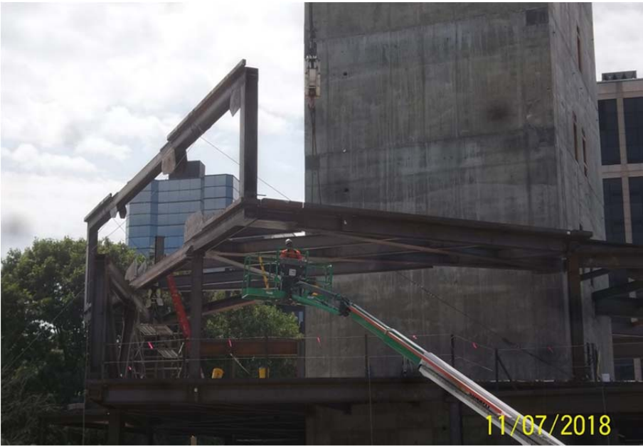
Erection of level 3 cantilevered truss
