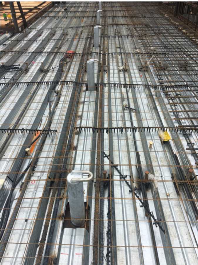
Concrete rebar and window washing davit bases
