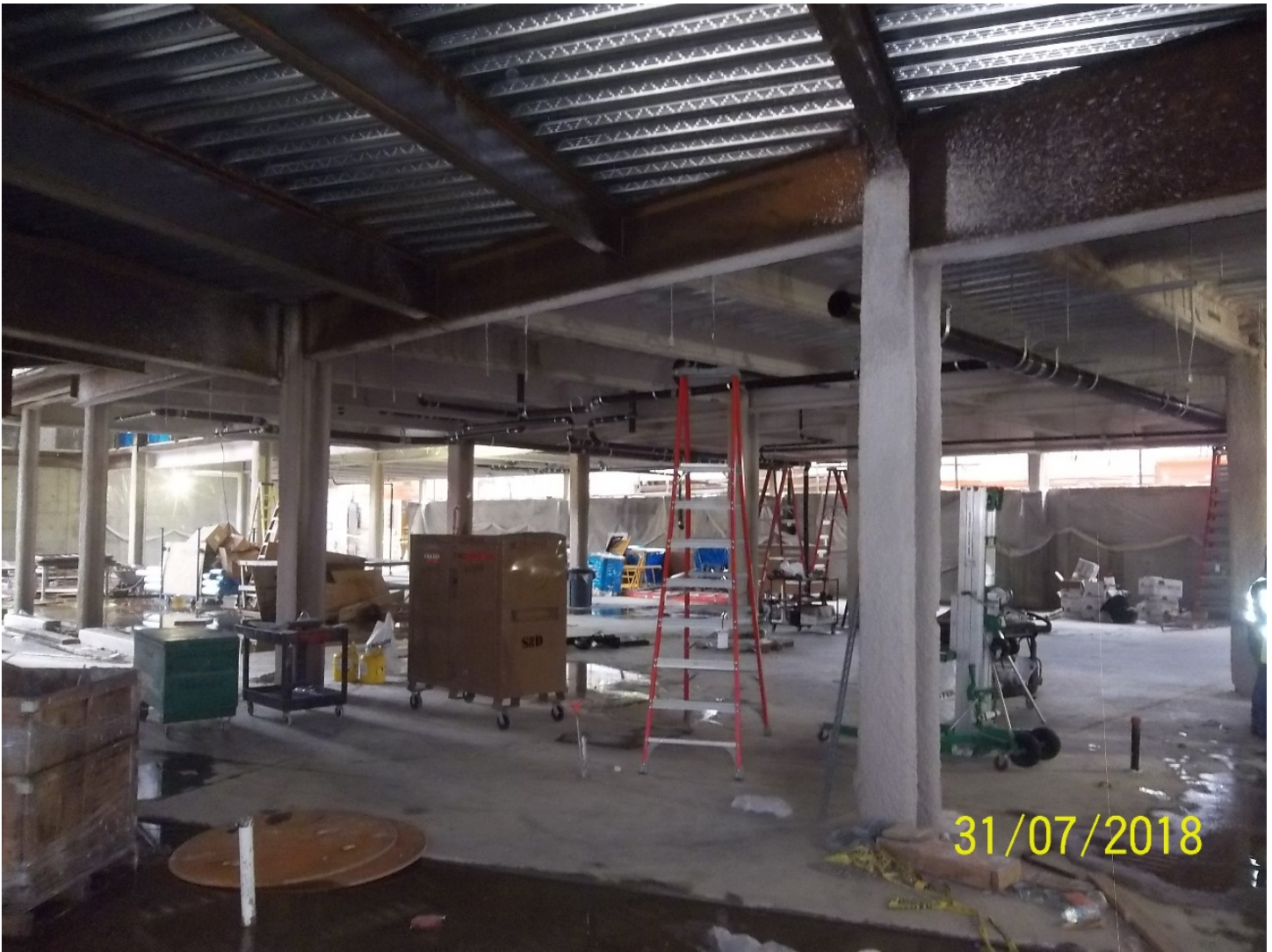
Plumbing rough-in at level G1 ceiling
