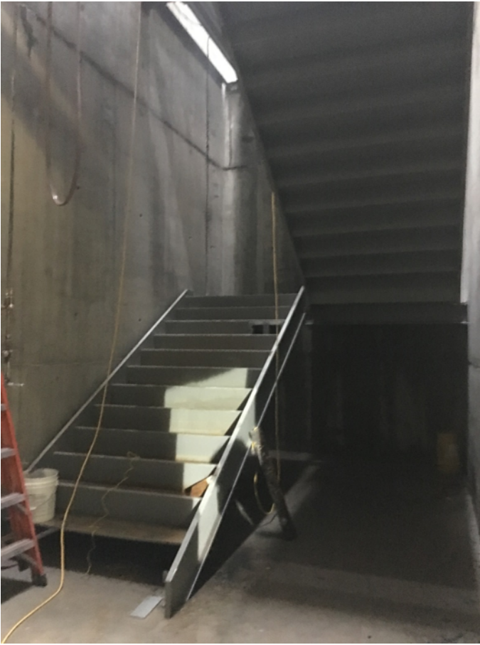
Stair #1 installed next to elevator shaft
