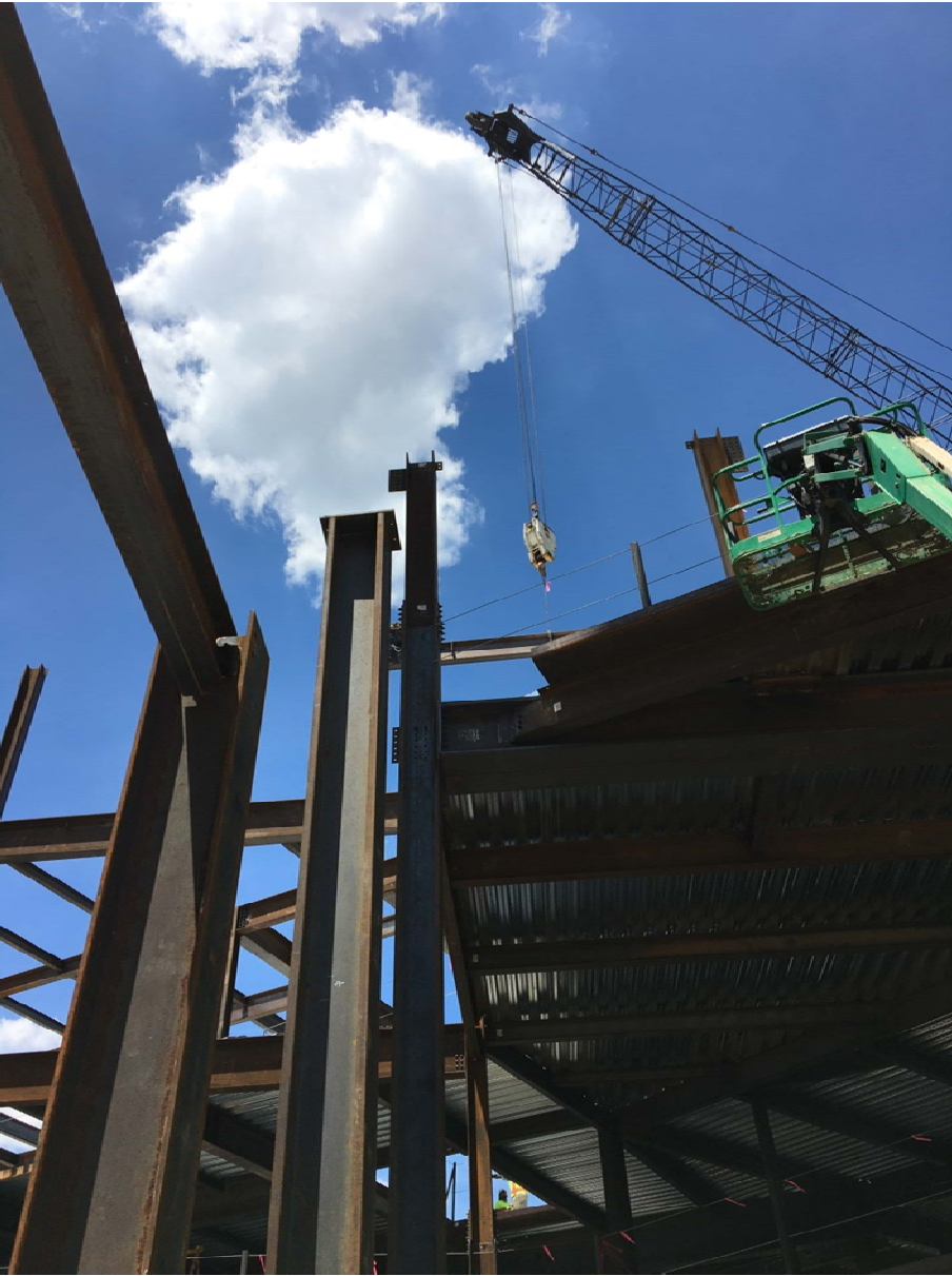
Erection of level 3 steel
