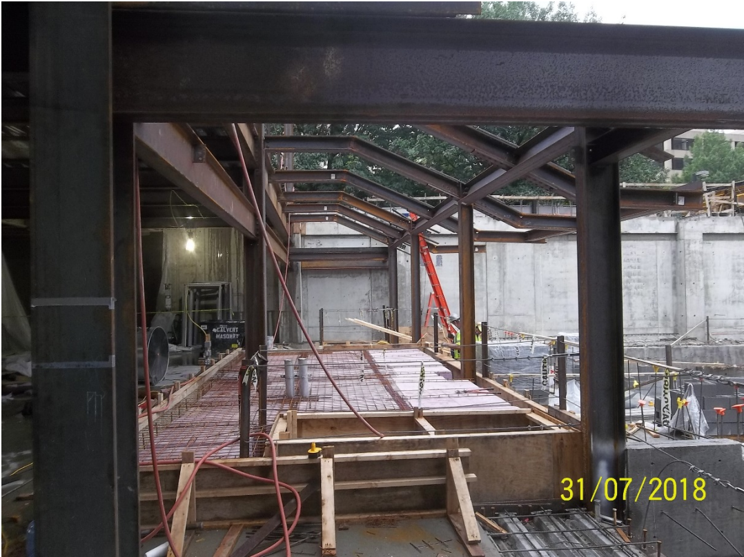
Steel framing at auditorium balcony
