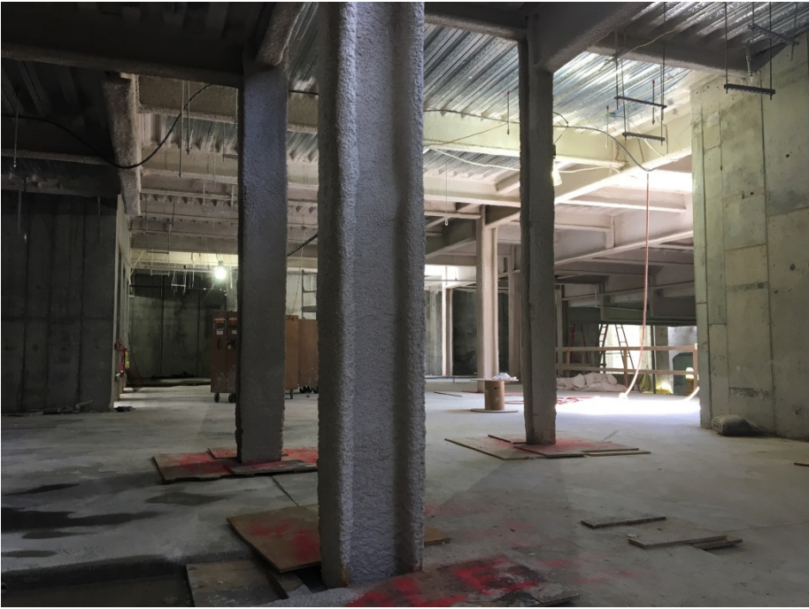
Spray fireproofing @ B2
