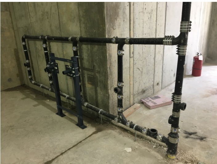
Plumbing installed at B2 level
