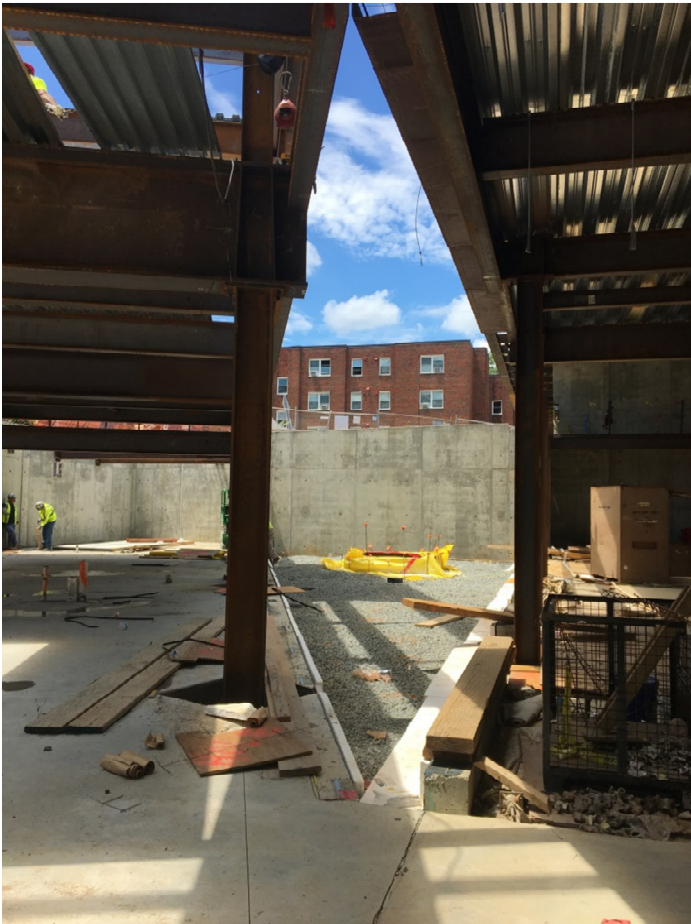
Courtyard next to auxiliary gym
