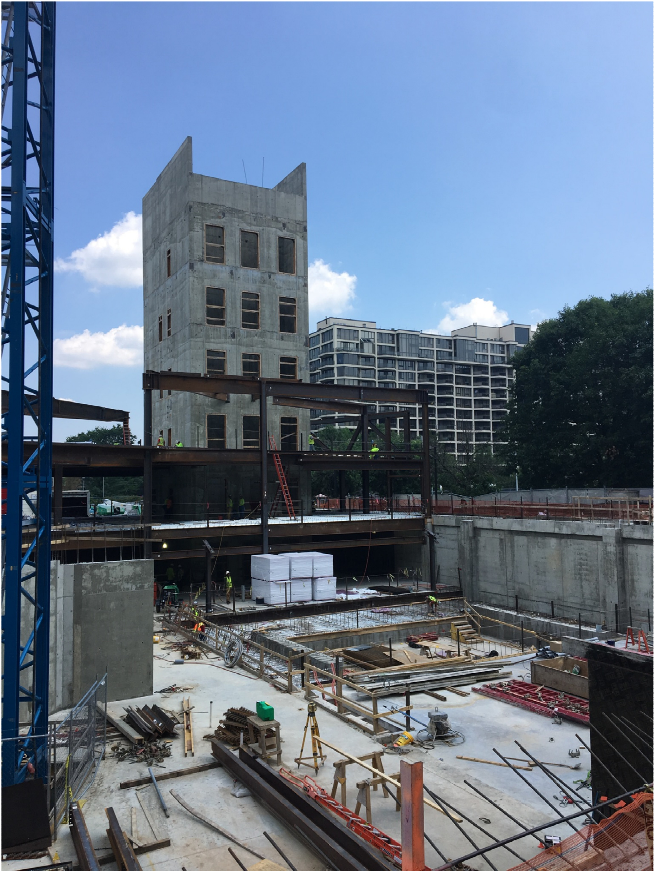
View from Wilson Blvd to future auditorium
