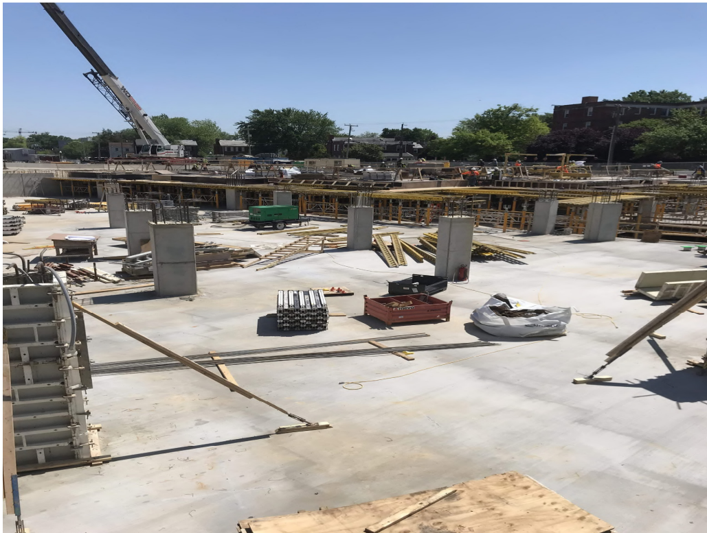
PROGRESSING FORMWORK FOR GROUND FLOOR DECK
