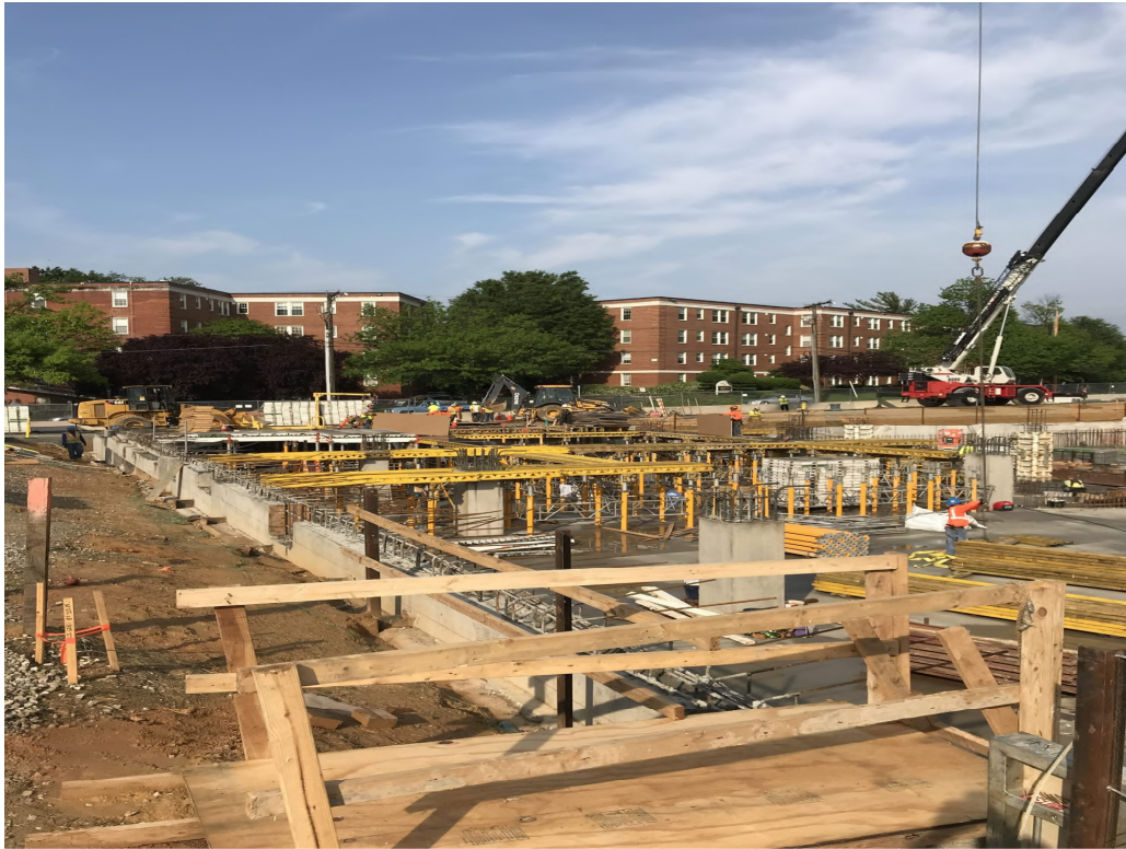
START OF PLACEMENT OF FORMWORK FOR GROUND FLOOR DECK
