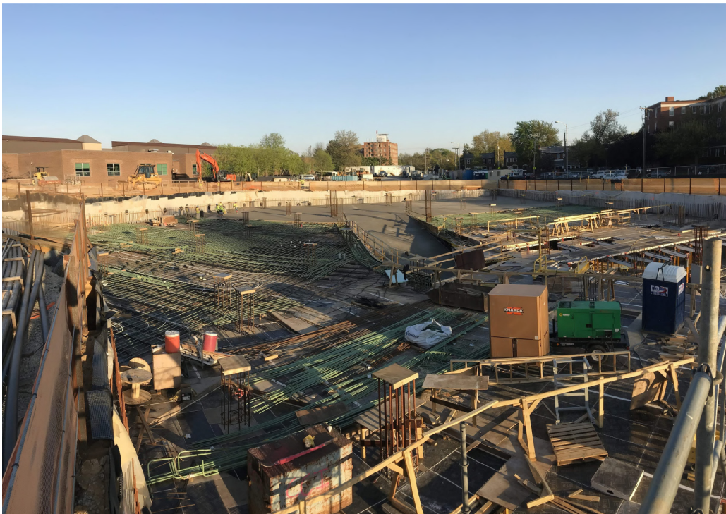
PARTIAL GARAGE UPPER LEVEL CONCRETE DECK AND INTERNAL GARAGE RAMP
