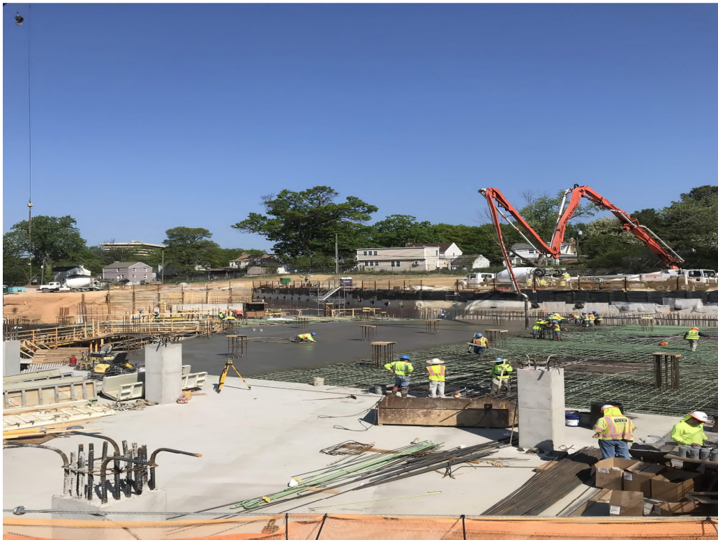
INSTALLATION OF CONCRETE AT GARAGE UPPER LEVEL DECK
