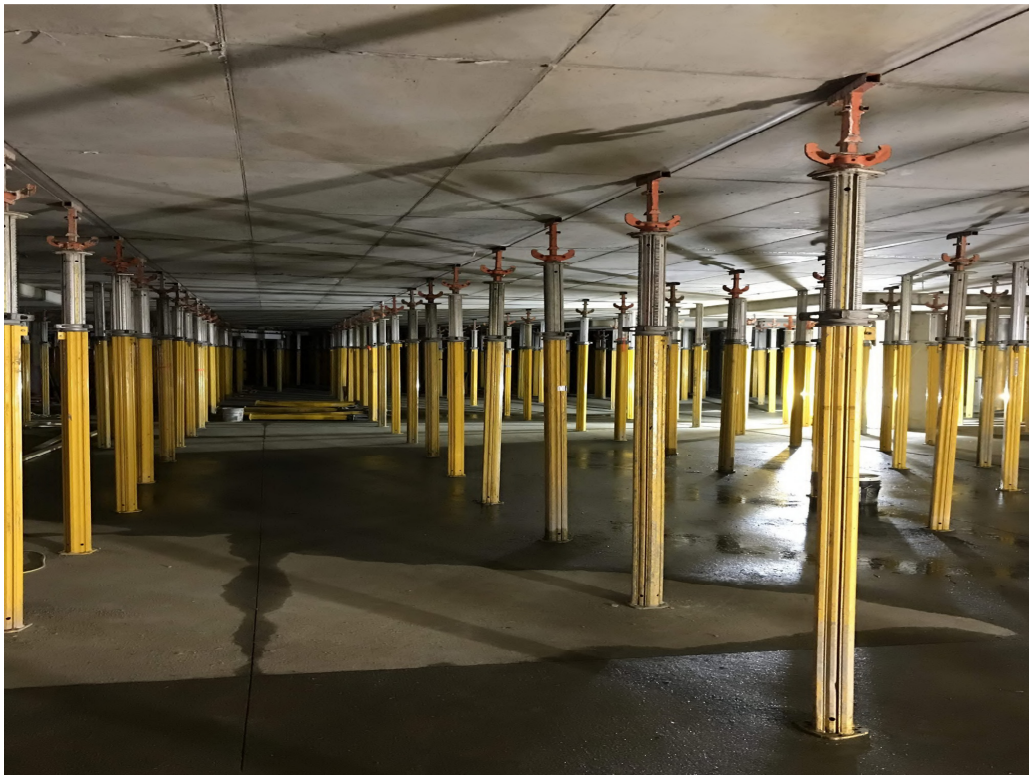
SHORING COLUMNS SUPPORTING GARAGE UPPER LEVEL DECK DURING CURE OF CONCRETE
