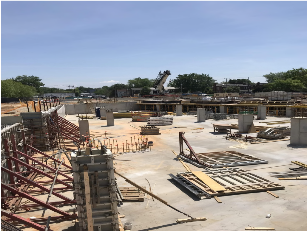
FORMWORK BEING SET FOR GARAGE UPPER LEVEL WALLS
