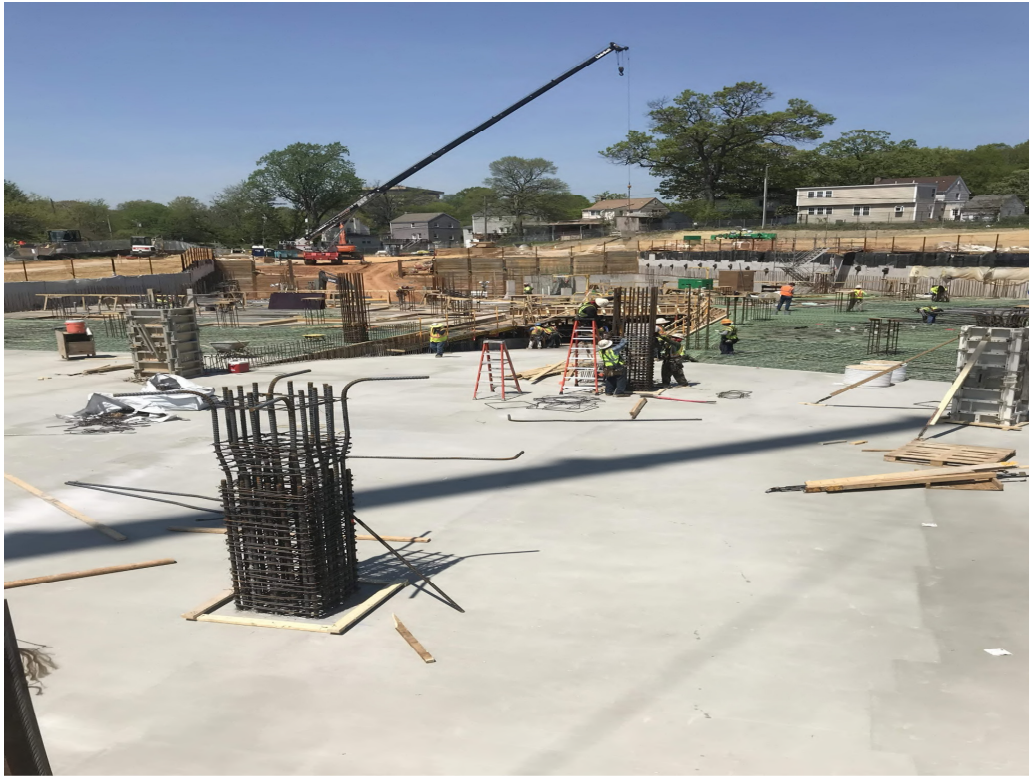
PLACEMENT OF REINFORCING STEEL FOR COLUMNS AT GARAGE UPPER LEVEL
