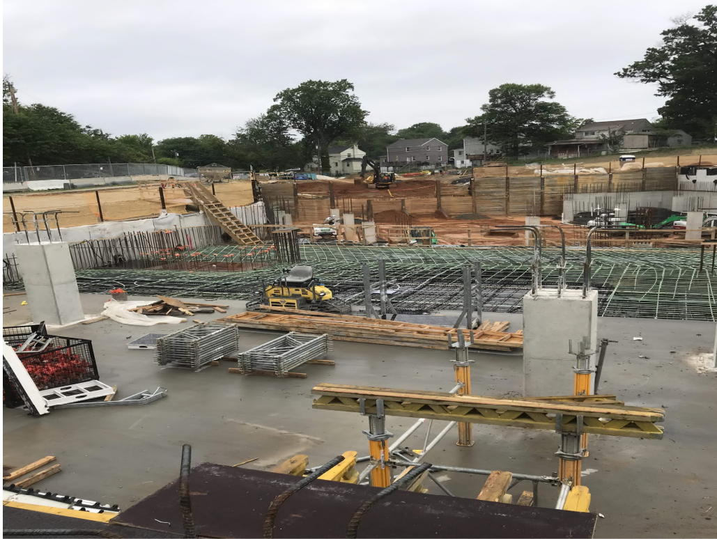
INSTALLATION OF REINFORCING STEEL AT GARAGE UPPER LEVEL DECK
