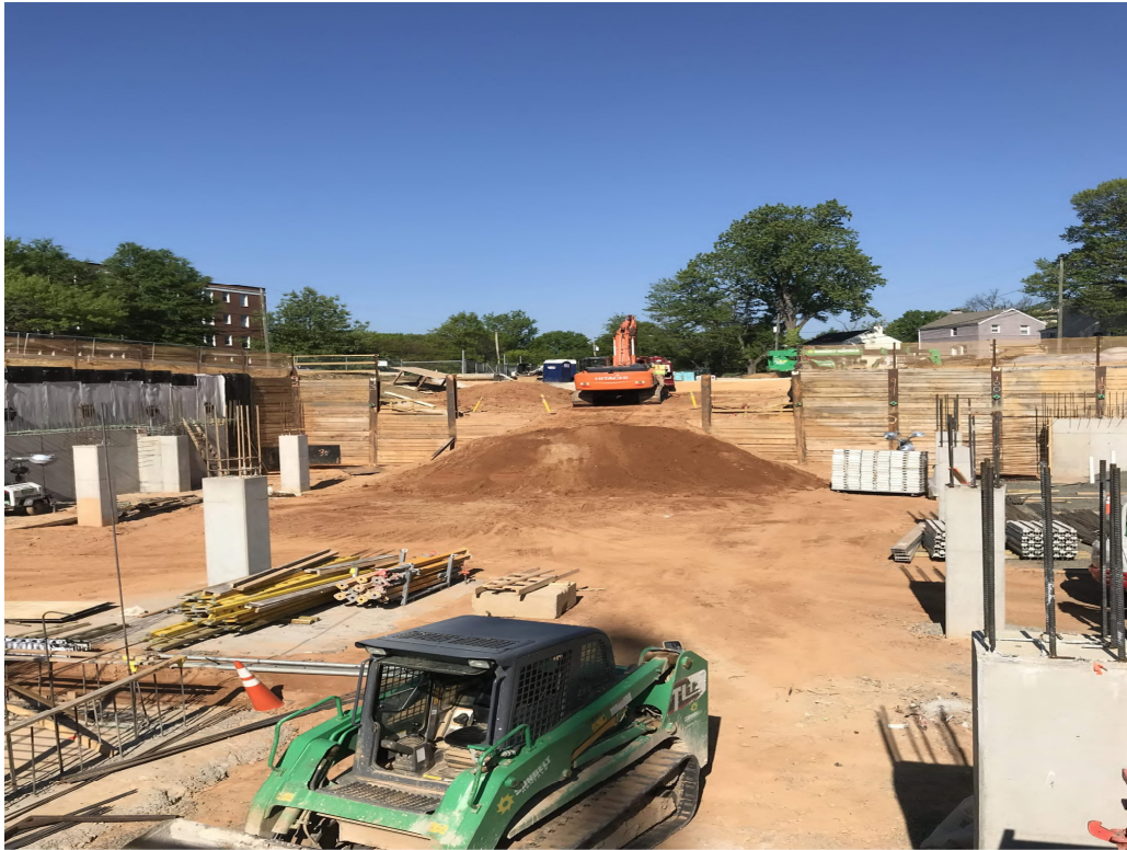
EXCAVATION FOR GARAGE ENTRY RAMP FROM BUS LOOP
