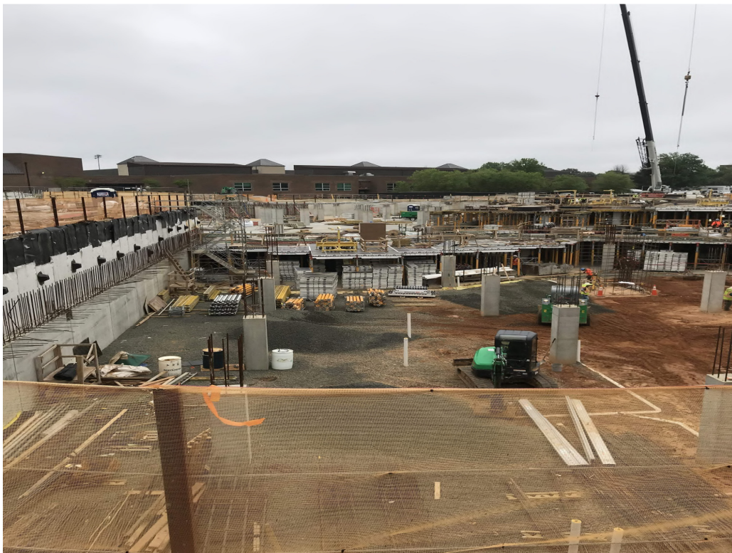
WORKING 2 GARAGE LEVELS AND GROUND FLOOR LEVEL SIMULTANEOUSLY
