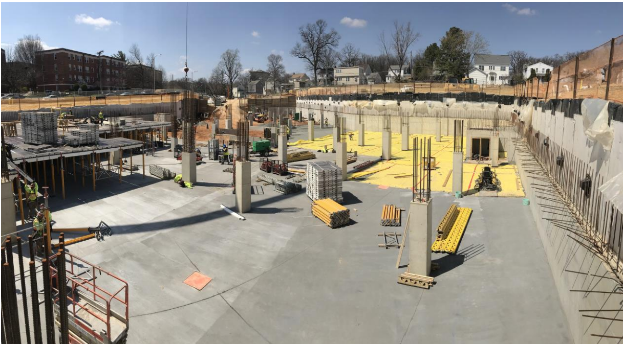
START OF PLACEMENT OF FORMWORK FOR GARAGE 2 ND LEVEL DECK
