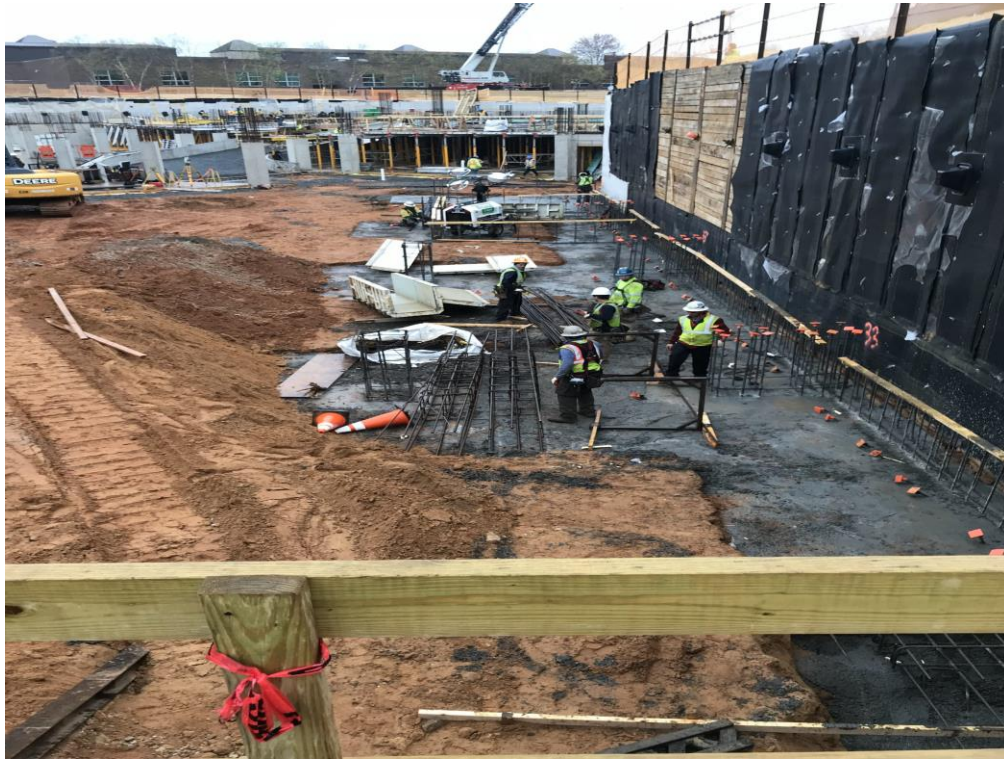
INSTALLATION OF CONCRETE AT GARAGE LOWER LEVEL FOOTINGS
