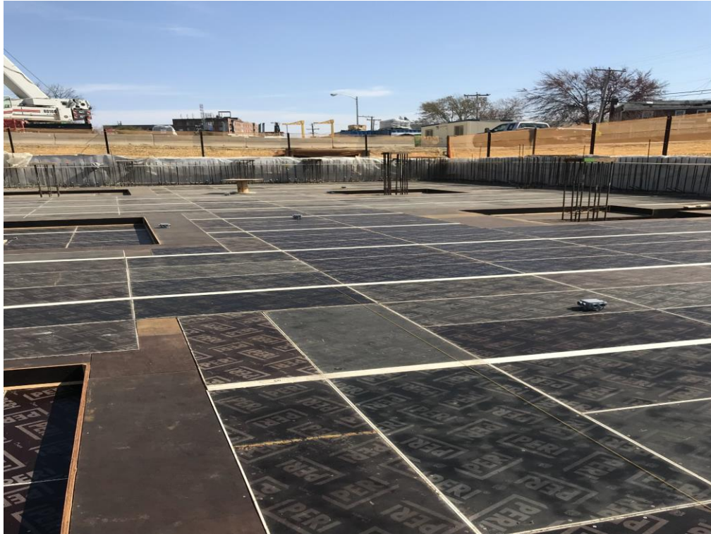
FORMWORK IN PLACE FOR GARAGE 2 ND LEVEL DECK
