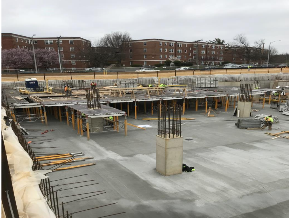
START OF PLACEMENT OF FORMWORK FOR GARAGE 2 ND LEVEL DECK
