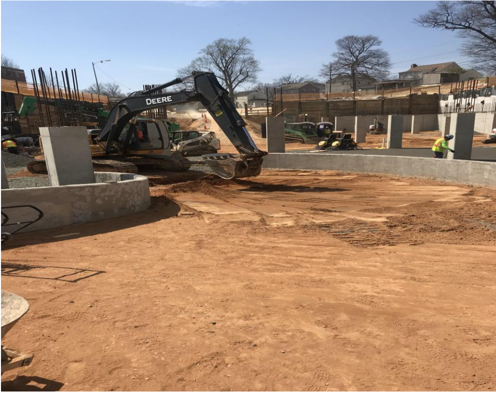
FINAL GRADING FOR GARAGE INTERNAL RAMP
