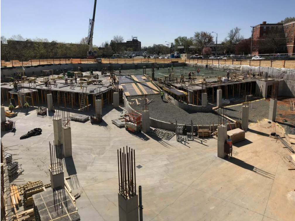
FINAL PREPARATION OF GARAGE INTERNAL RAMP PRIOR TO CONCRETE POUR
