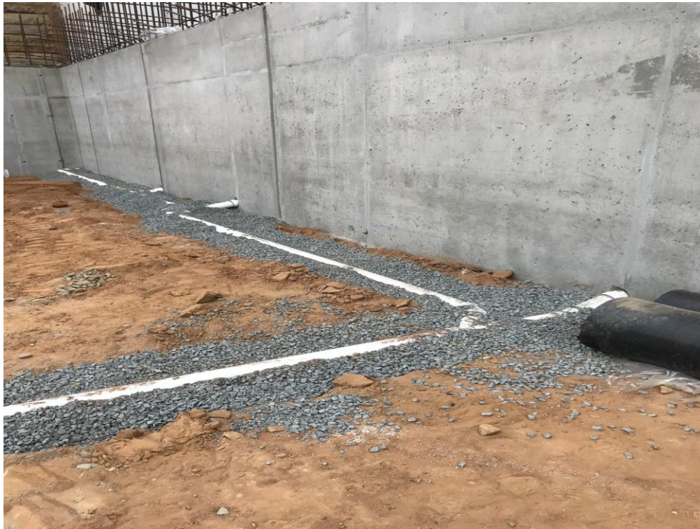
DRAINAGE PIPING UNDER GARAGE LOWER LEVEL SLAB
