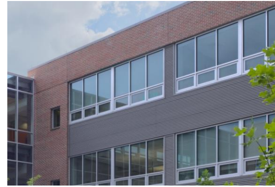
Used as in-fill with brick
