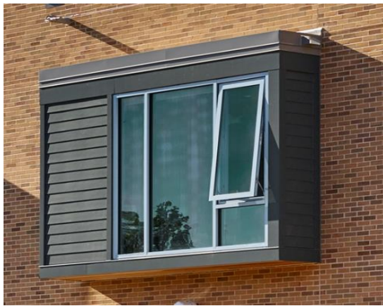
lap siding & trim used together
