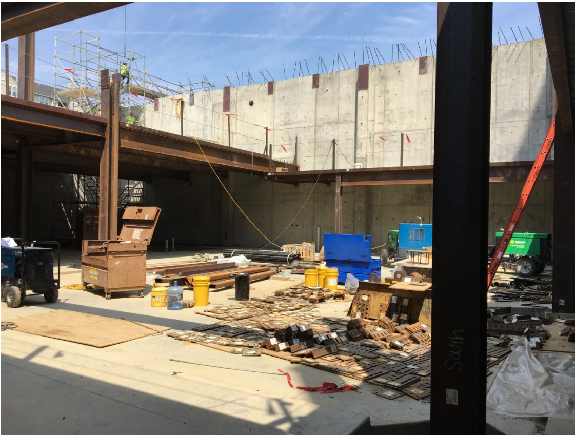
Steel beams around black box theater
