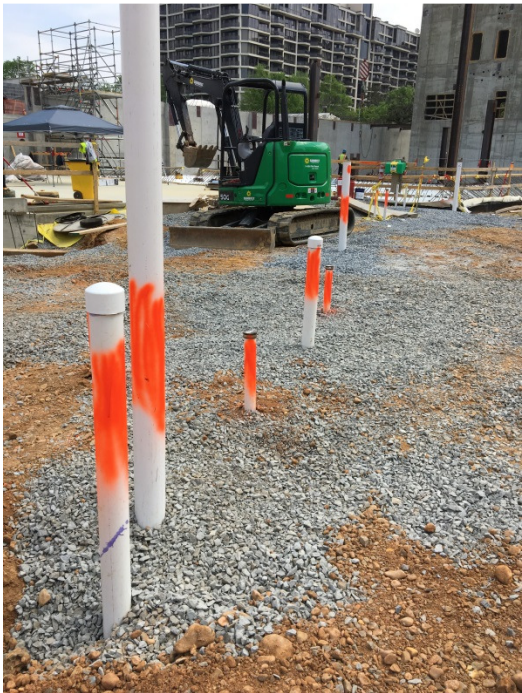
Underground sanitary installed
