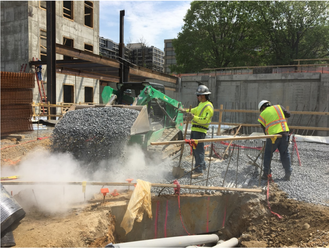
Prepare for concrete slab
