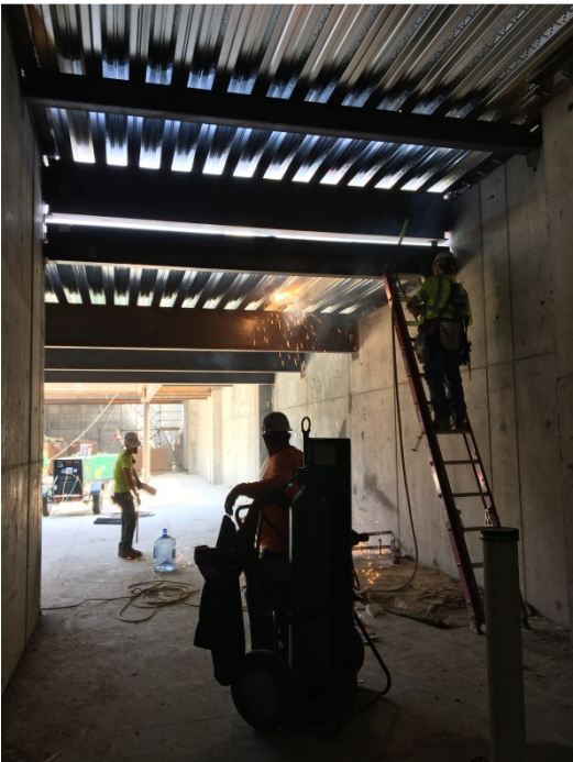
Metal decking around elevator core
