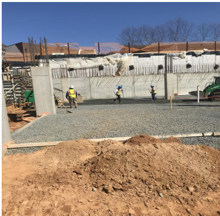
INSTALL OF GRAVEL BASE FOR GARAGE SLAB CONCRETE
