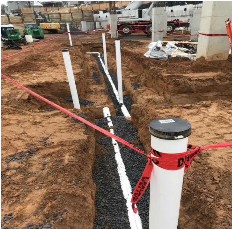
INSTALL OF BELOW SLAB PIPING FOR GARAGE IN-SLAB DRAINS
