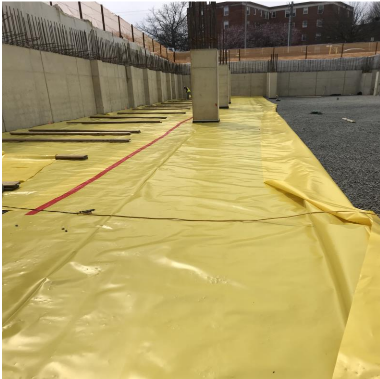
INSTALL OF VAPOR BARRIER OVER GRAVEL BASE FOR GARAGE SLAB
