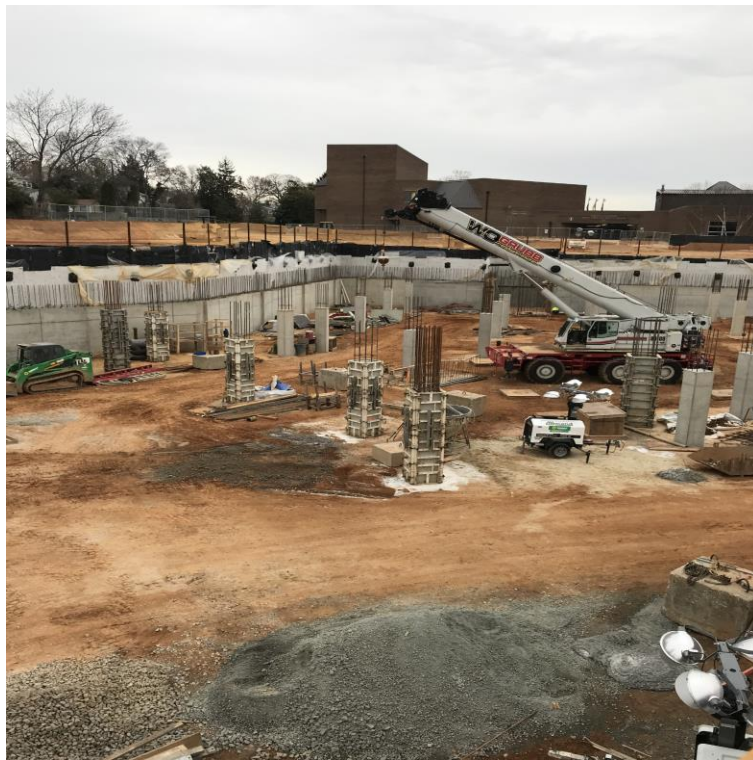
PLACEMENT OF FORMWORK FOR GARAGE COLUMNS
