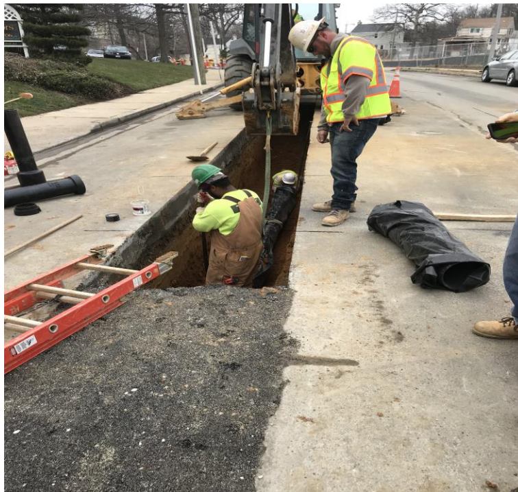
WATERLINE REPLACEMENT IN SOUTH OLD GLEBE ROAD
