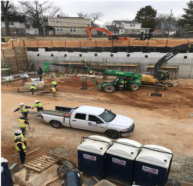
PLACEMENT OF FORMWORK FOR GARAGE WALLS
