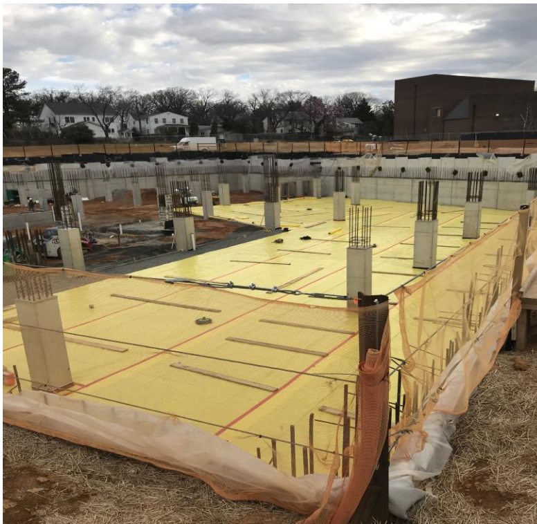
OVERVIEW OF VAPOR BARRIER INSTALL FOR GARAGE SLAB
