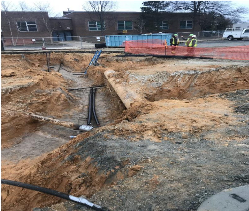
GEOHERMAL HORIZONTAL PIPING INSTALLATION
