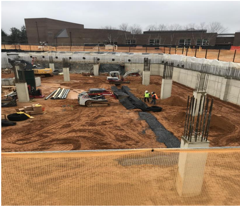
INSTALLATION OF SLAB UNDERDRAIN PIPING AT LOWEST GARAGE LEVEL
