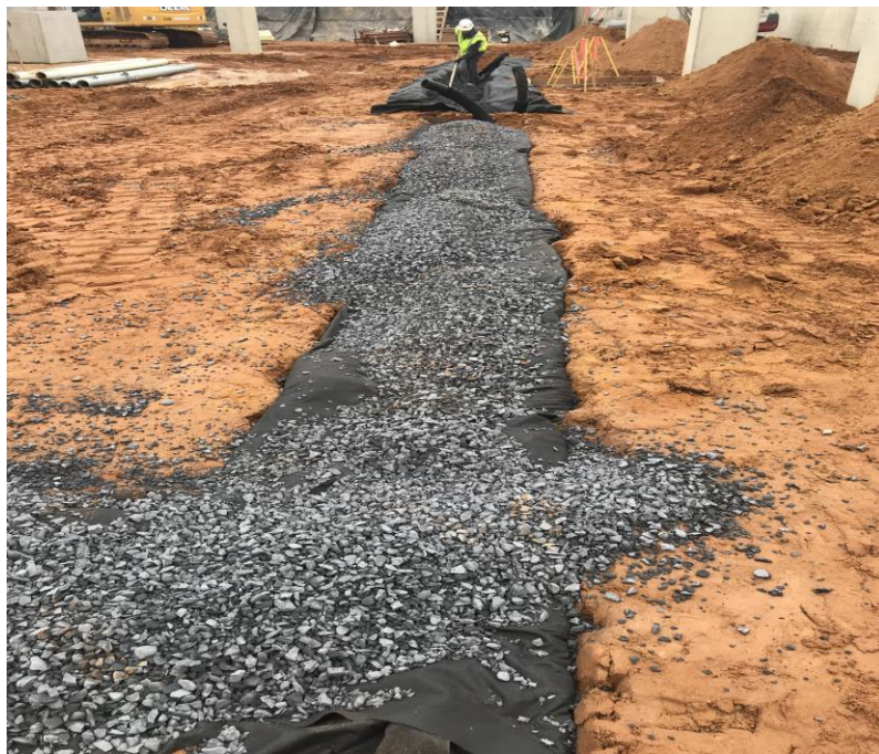
DETAIL OF SLAB UNDERDRAIN PIPING INSTALLATION
