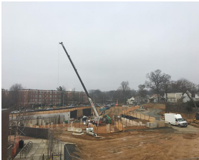
MOBILE CRANE WITHIN GARAGE EXCAVATION AND STABILIZED BUS LOOP ROAD ABOVE
