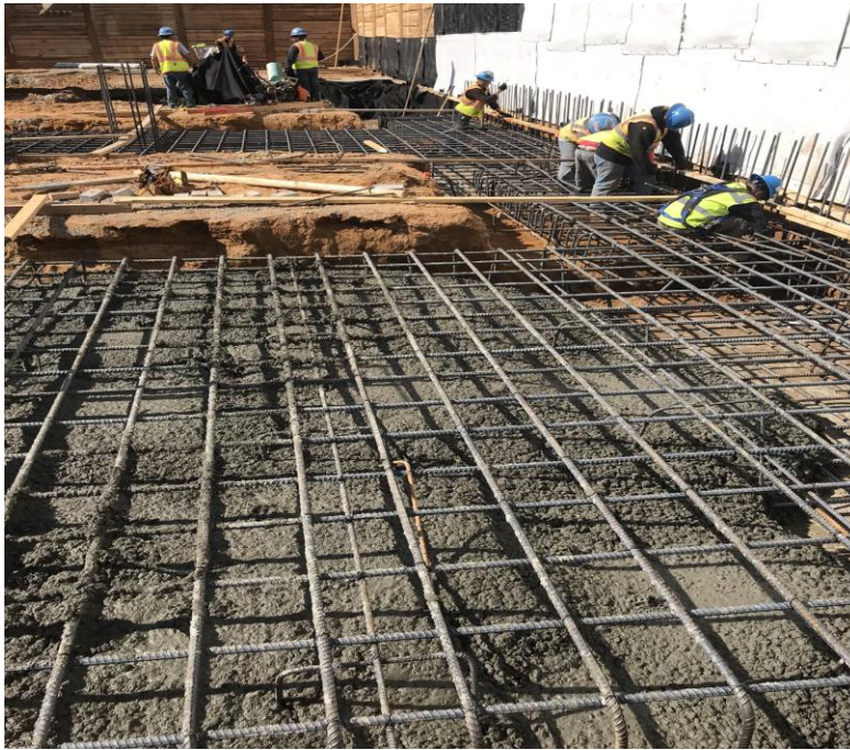
INSTALLATION OF REINFORCING STEEL BAR (REBAR) FOR GARAGE FOOTINGS
