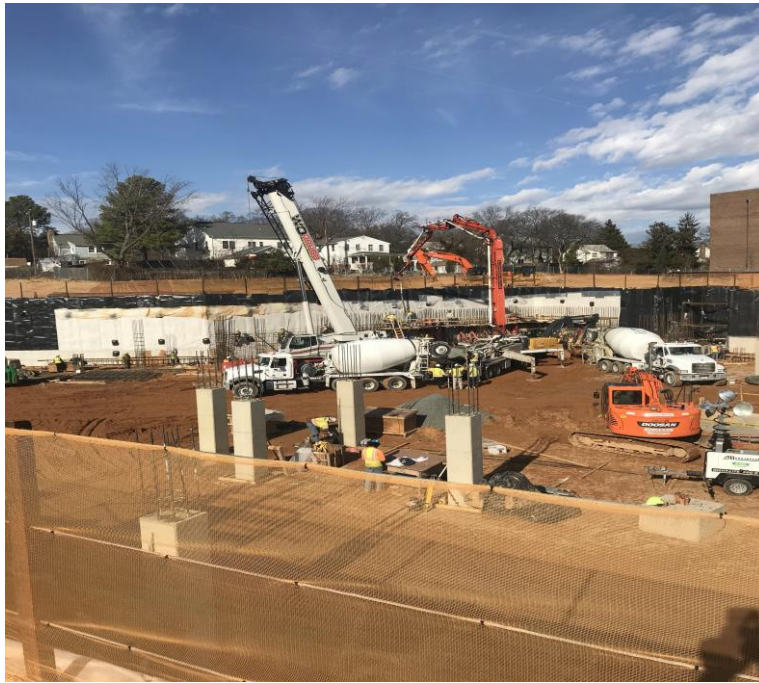
POURING OF CONCRETE FOR GARAGE LOWER LEVEL WALLS WITH CONCRETE PUMPER
