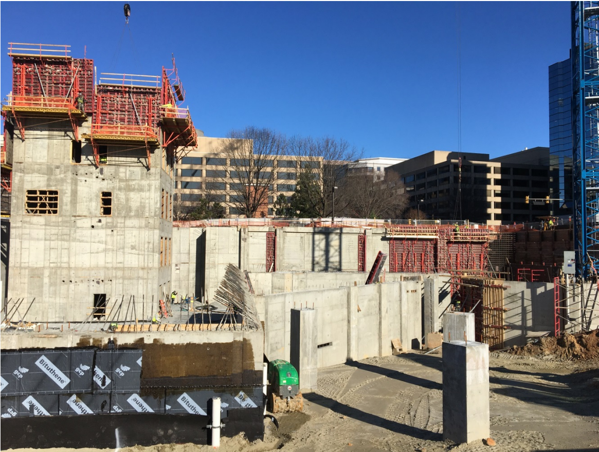
B2 foundation wall
