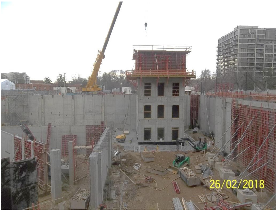
Elevator core formed @ Level 2
