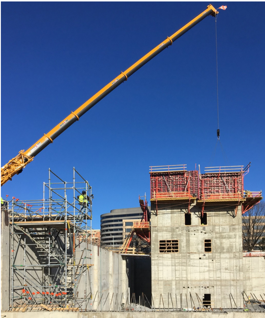
Installing forms @ elevator core
