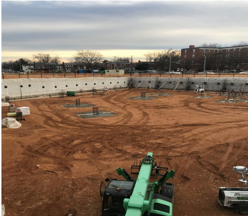
POURED GARAGE COLUMN FOOTINGS
