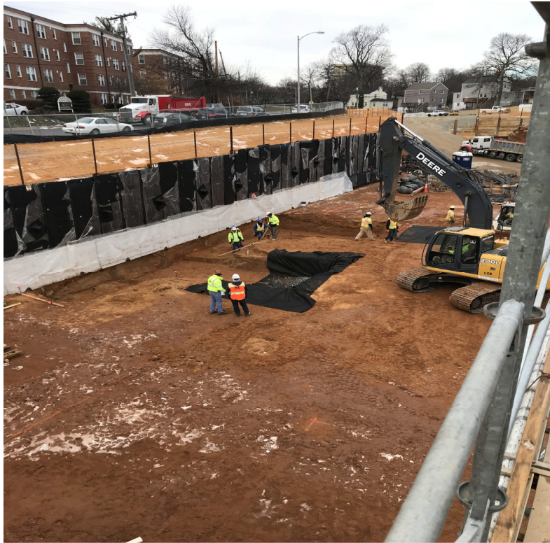
EXCAVATION FOR GARAGE FOOTINGS
