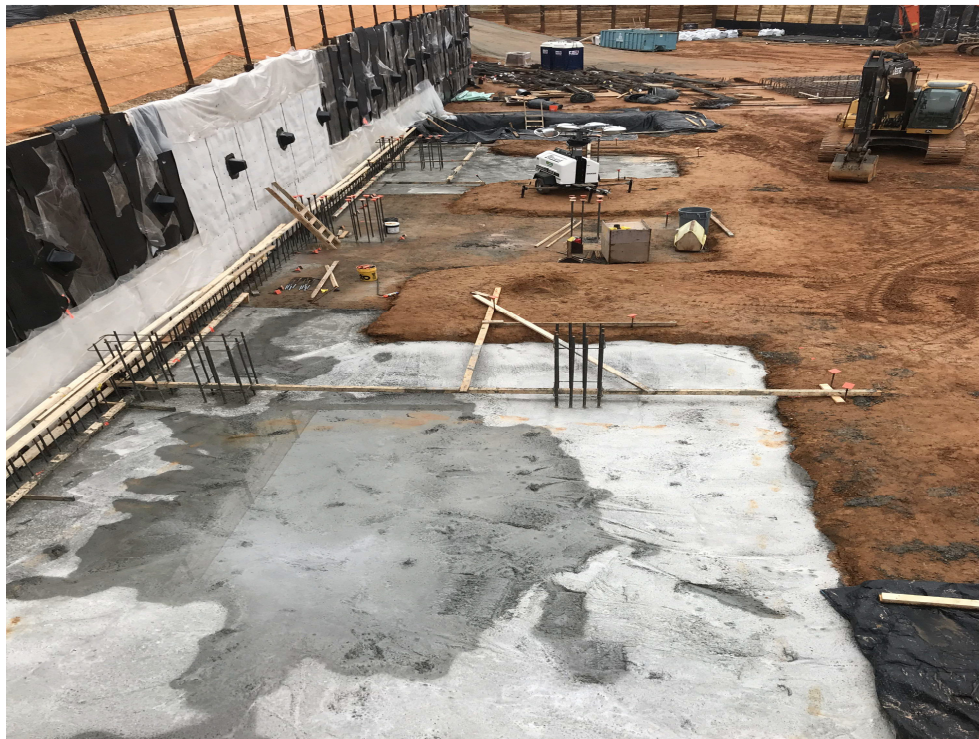
POURED FOOTINGS AT LOWEST GARAGE LEVEL
