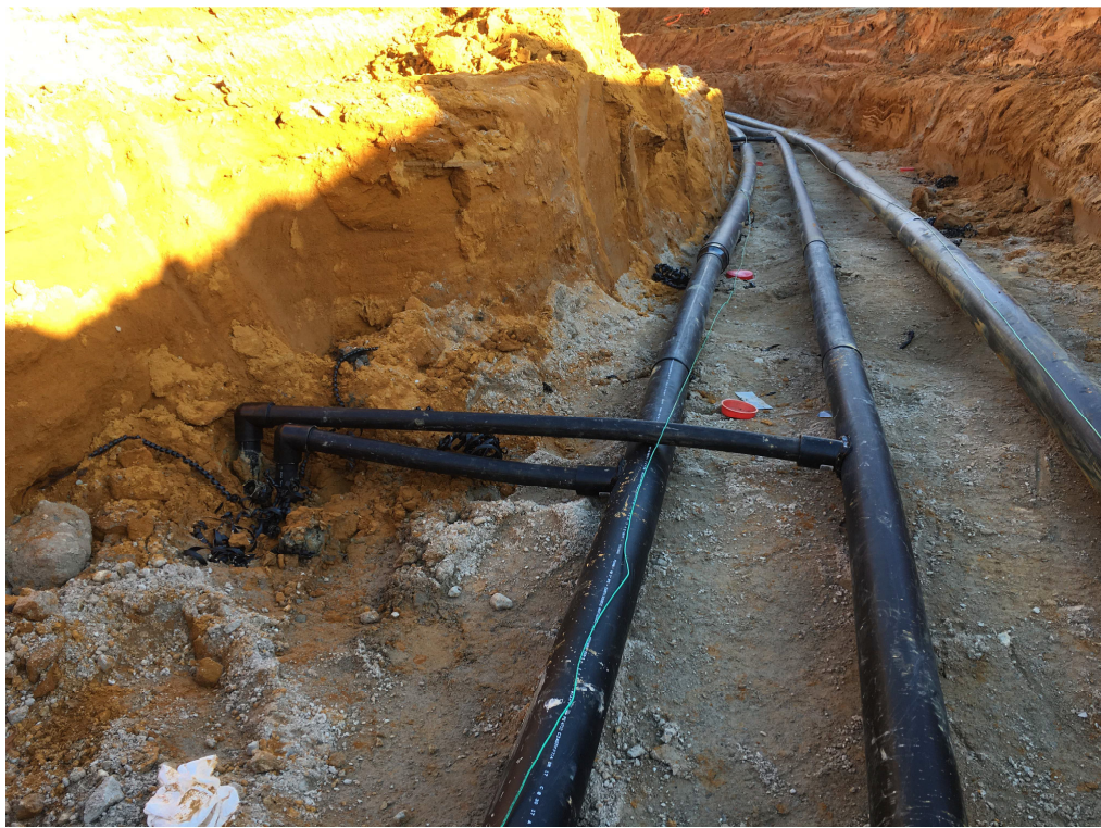
GEOHERMAL HORIZONTAL PIPING INSTALLATION
