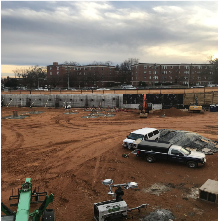
INSTALLED REBAR AT FOUNDATION WALLS PRIOR TO PLACEMENT OF FORMWORK
