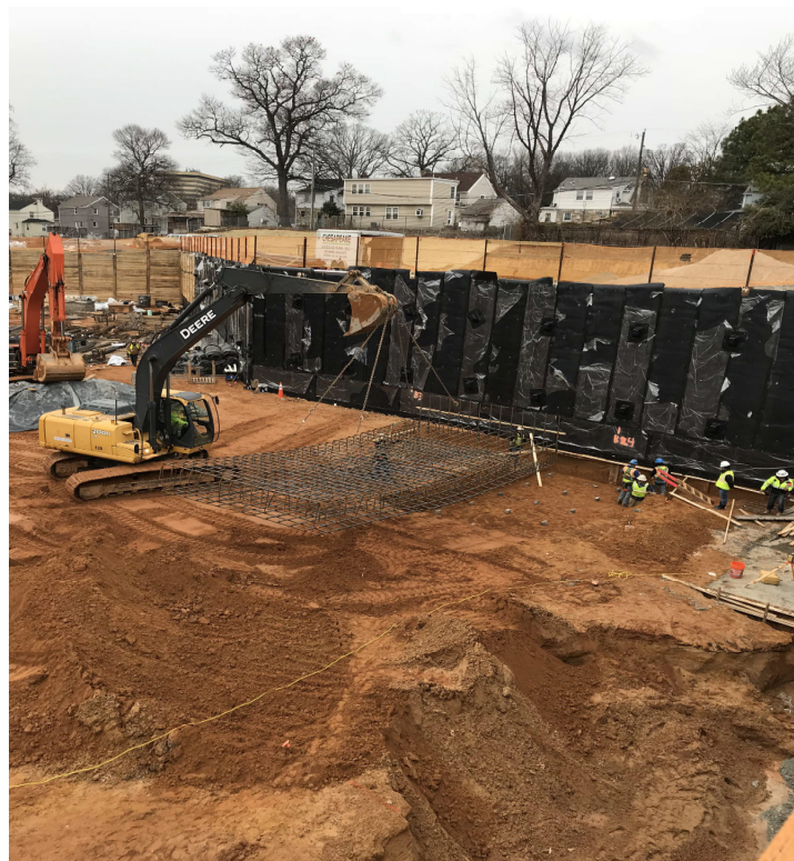
INSTALLATION OF REINFORCING STEEL BAR (REBAR) FOR GARAGE FOOTINGS
