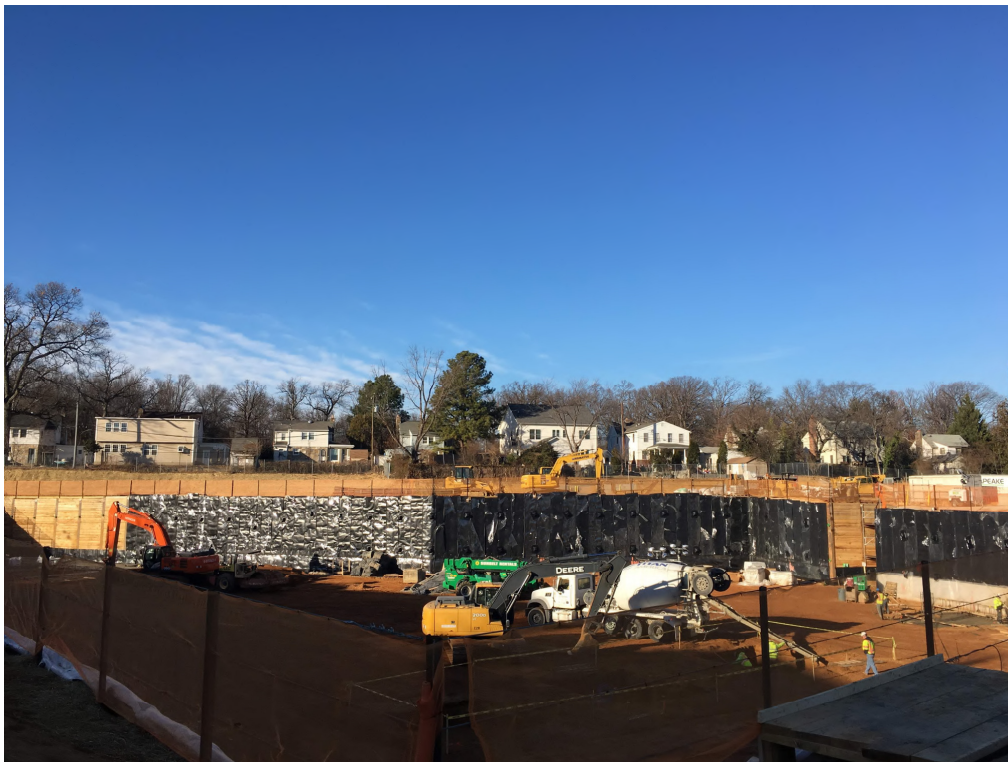
POURING FOOTINGS AT LOWEST GARAGE LEVEL
