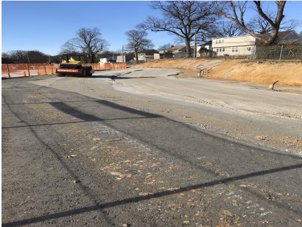
BUS LOOP STABILIZATION WITH STONE BASE
