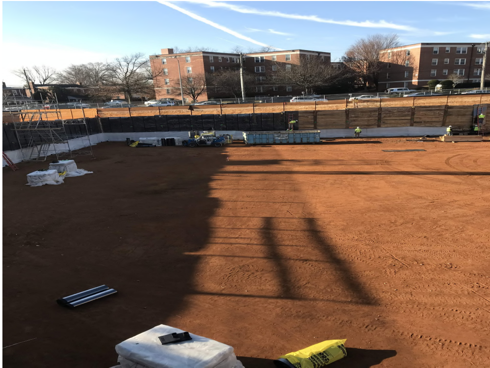
WATERPROOFING OF GARAGE FOUNDATION WALLS
