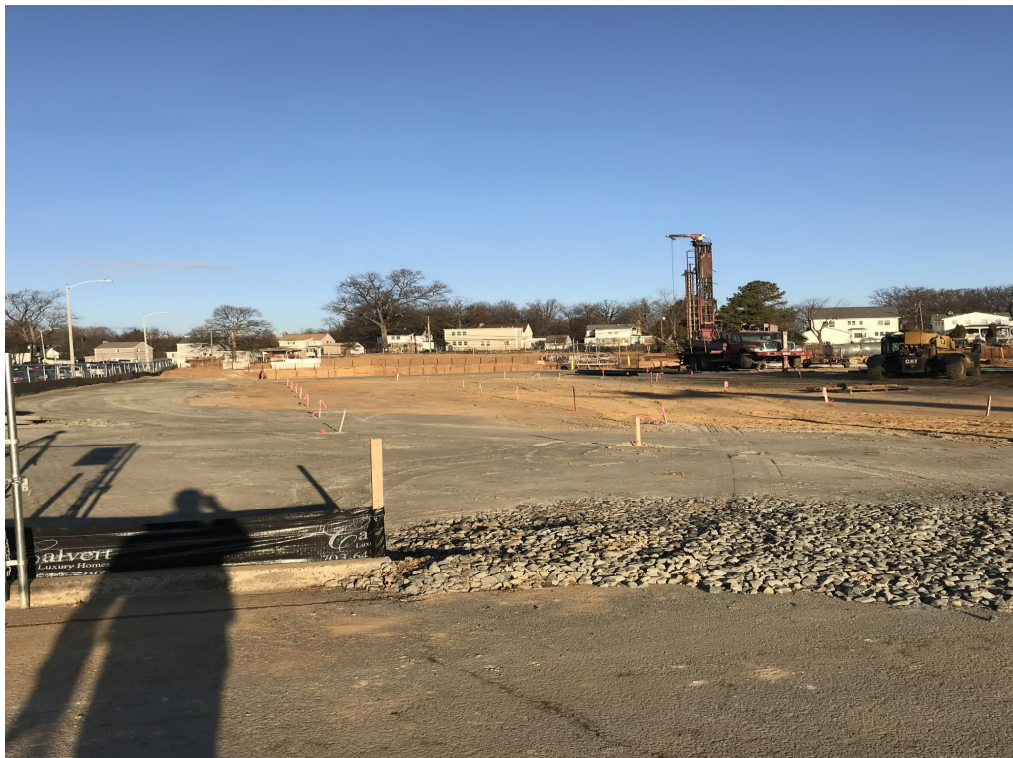
GEOTHERMAL WELL DRILLING AT WELL FIELD SOUTH OF GARAGE
