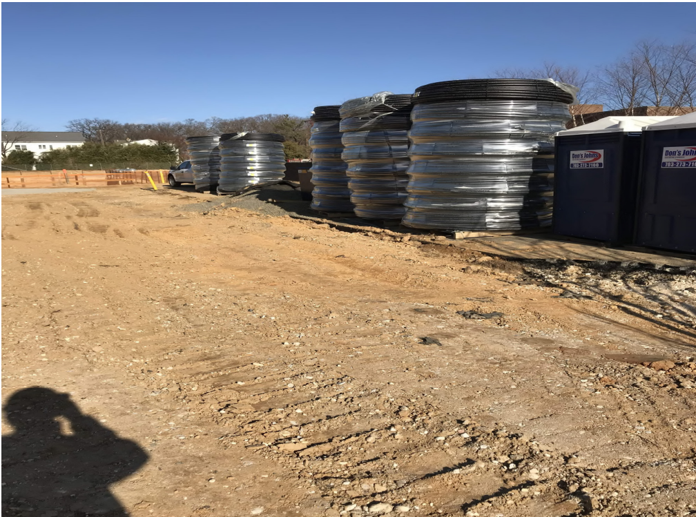
STAGING OF GEOTHERMAL WELL FIELD PIPING
