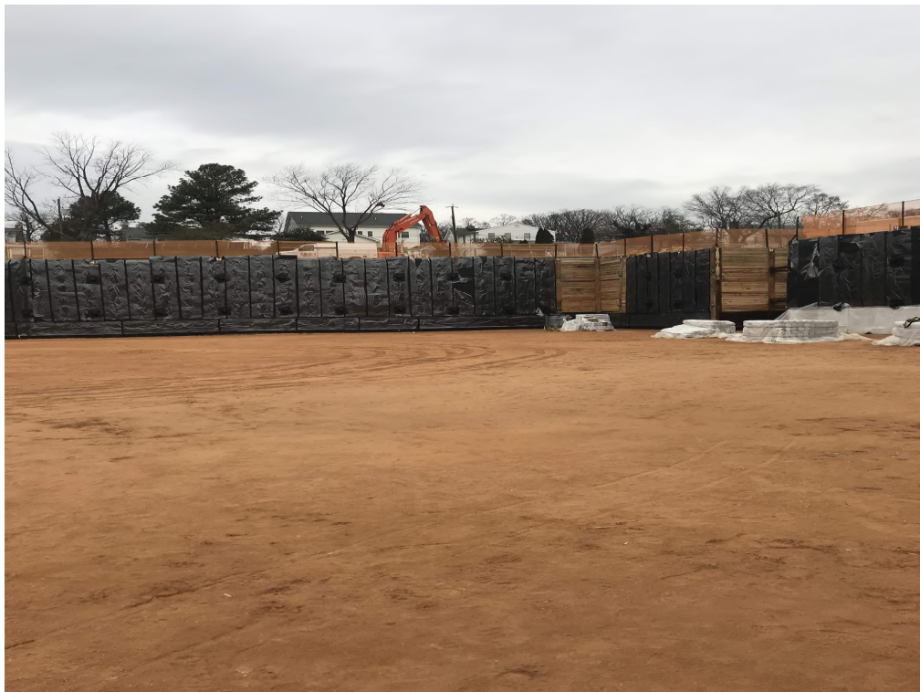
WATERPROOFING OF GARAGE FOUNDATION WALLS
