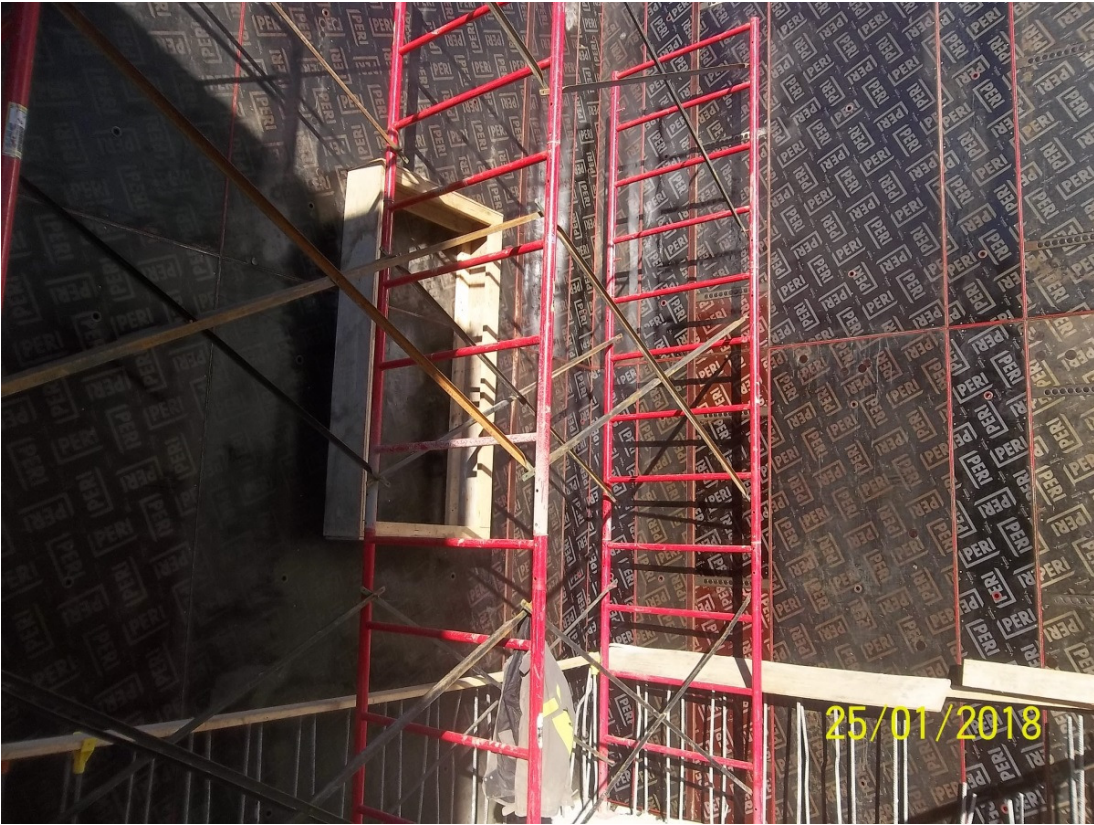
Steel formwork and rebar
