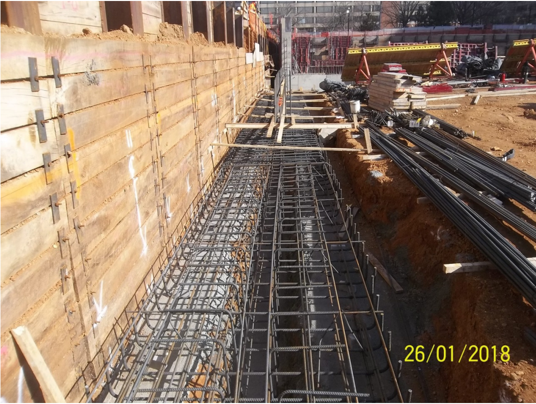
Foundation rebar
