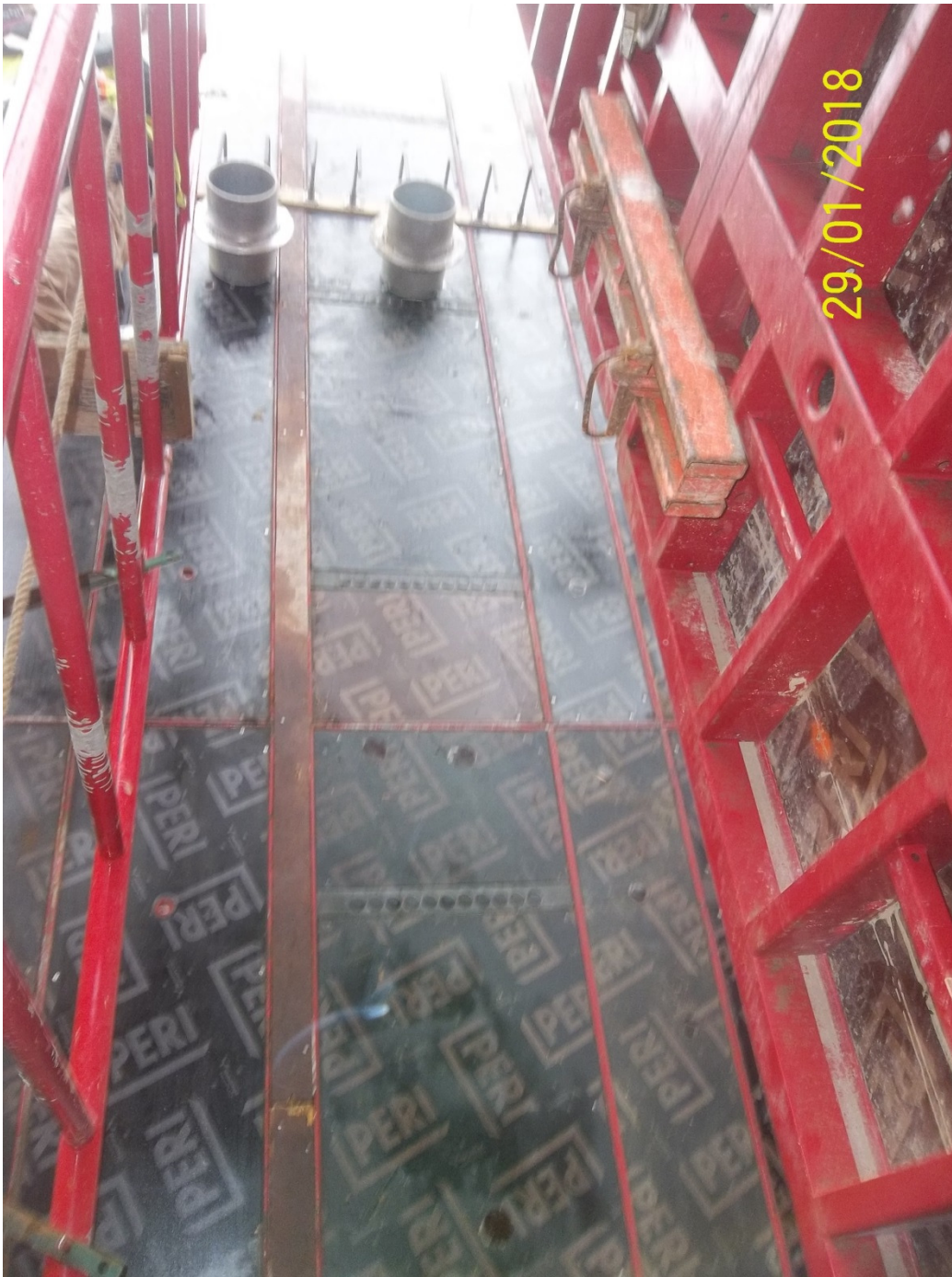
Steel formwork and wall sleeves
