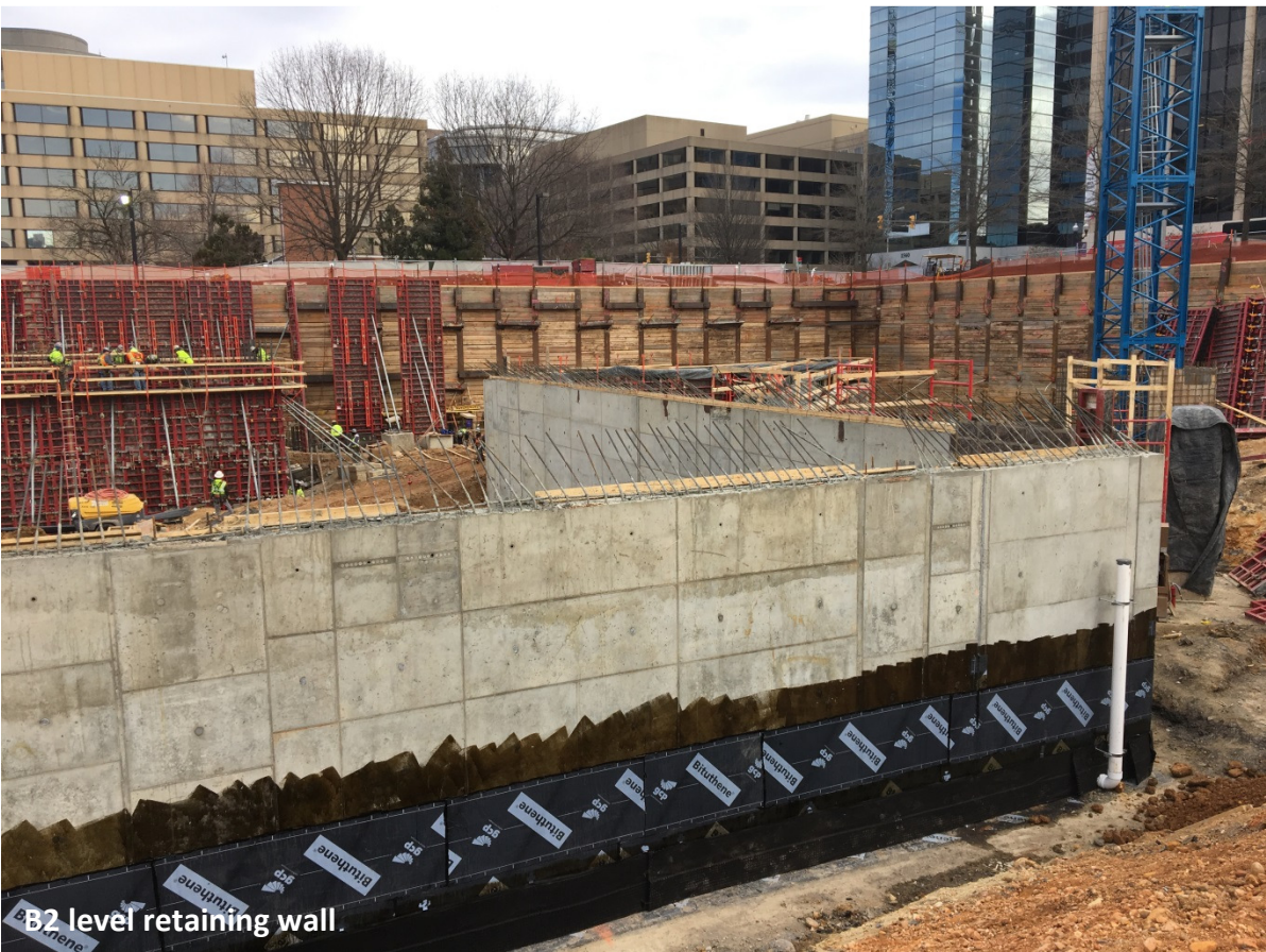
B2 level soil final grading for slab on grade
