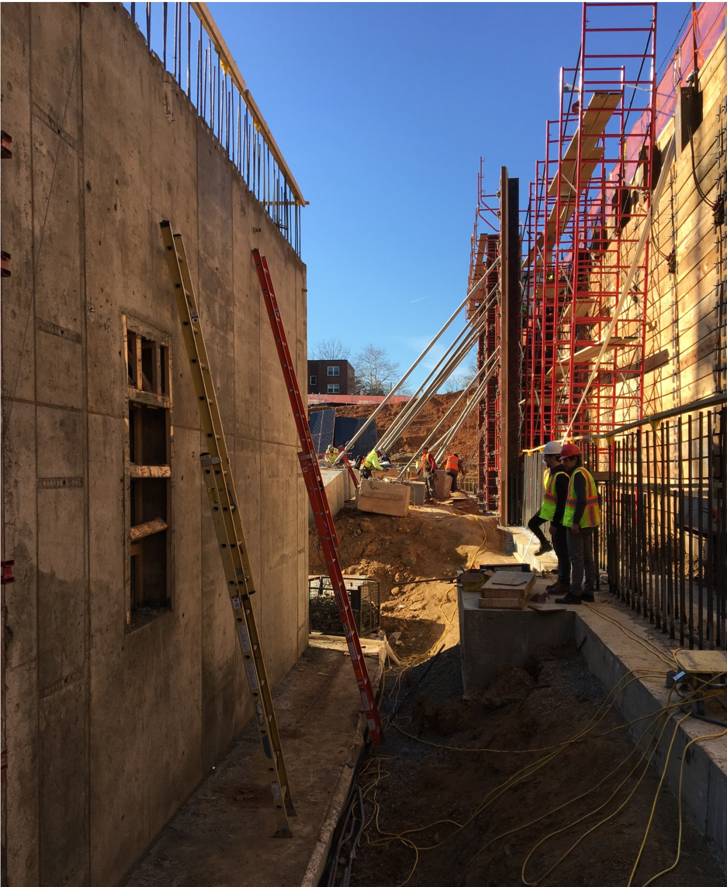
Form removed for B2 level elevator core concrete wall
