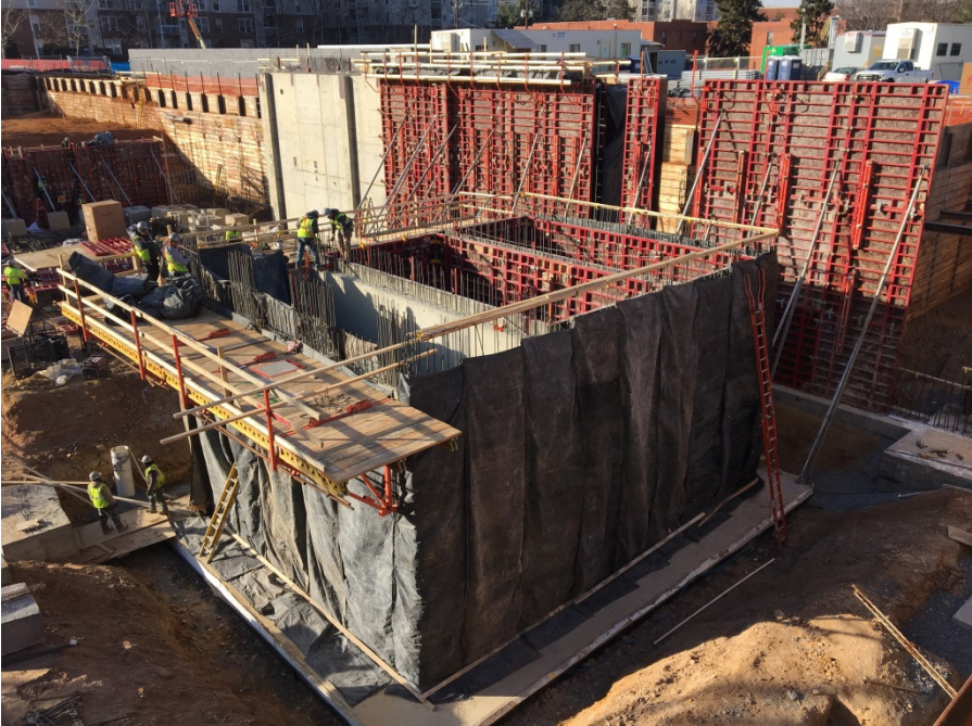
Start forming ground level elevator core
