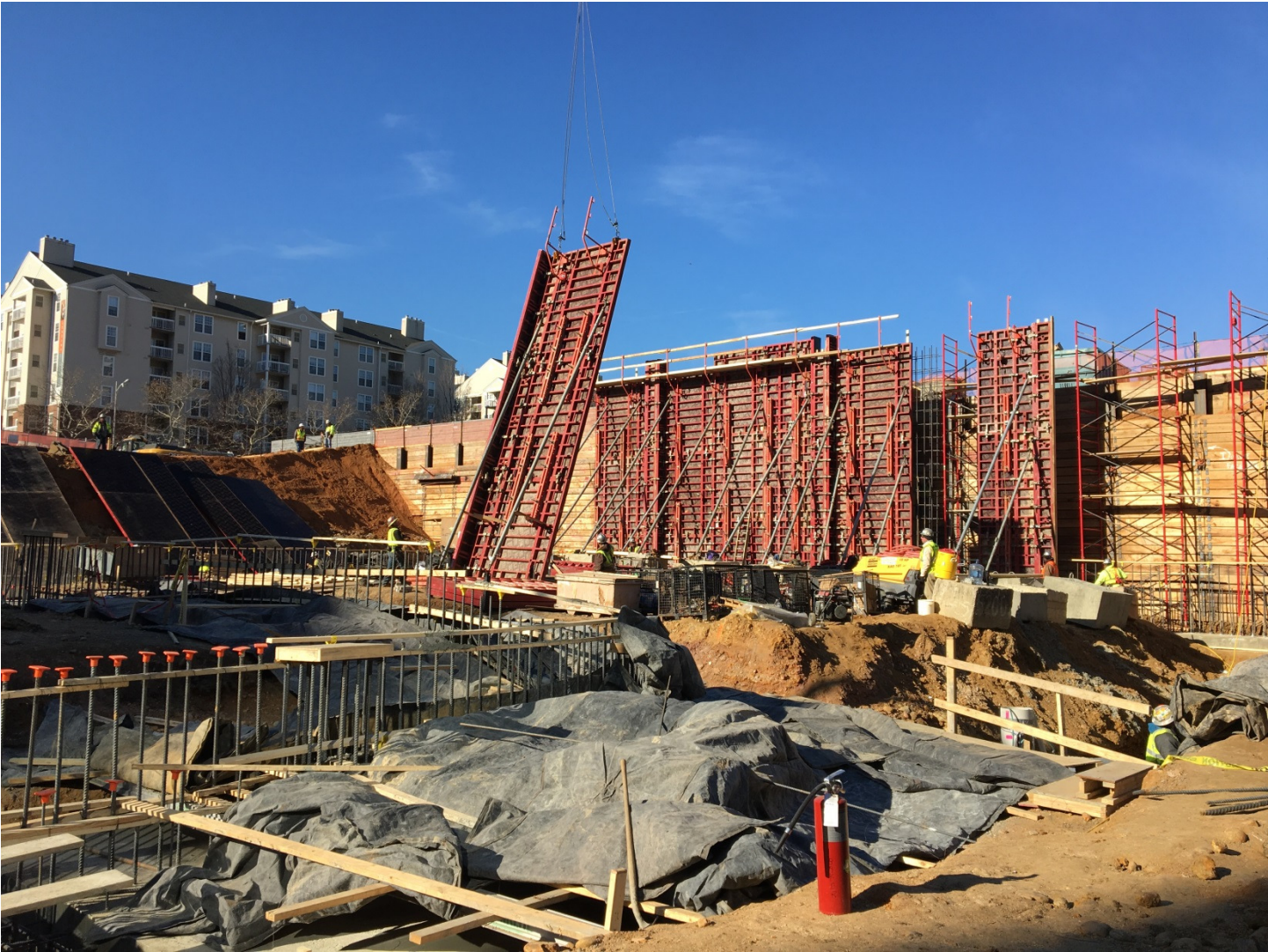
Erecting form for basement retaining wall
