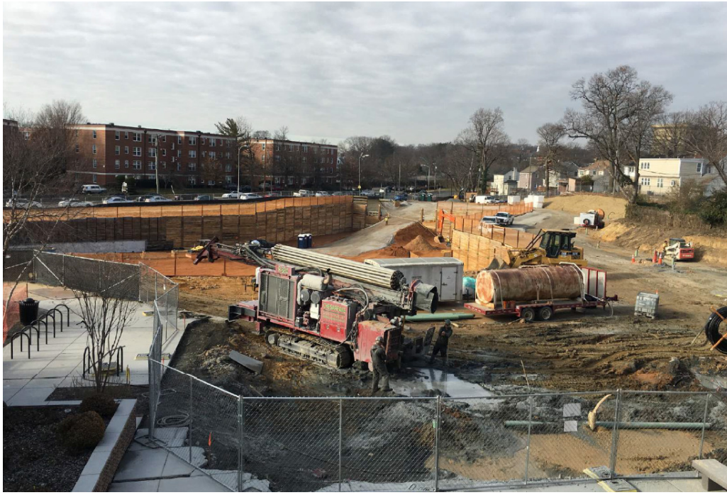
GEOHERMAL WELL DRILLING AT WELL FIELD UNDER THE BUS LOOP
