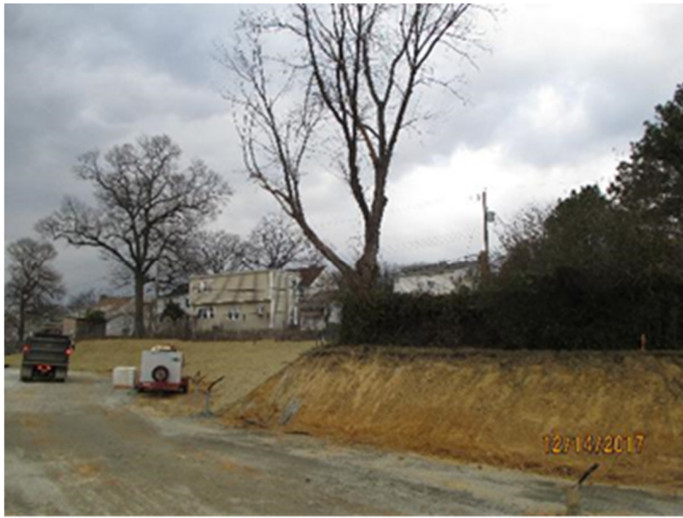
BUS LOOP GRADING AND STABILIZATION
