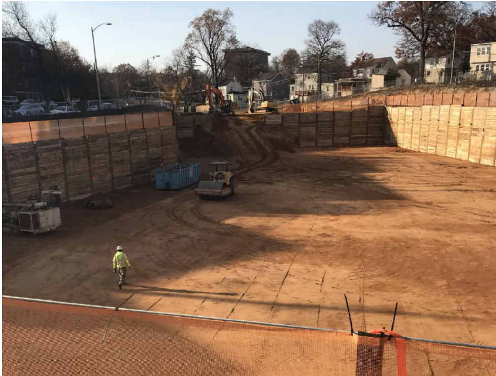
VEHICLE RAMP INTO GARAGE EXCAVATION
