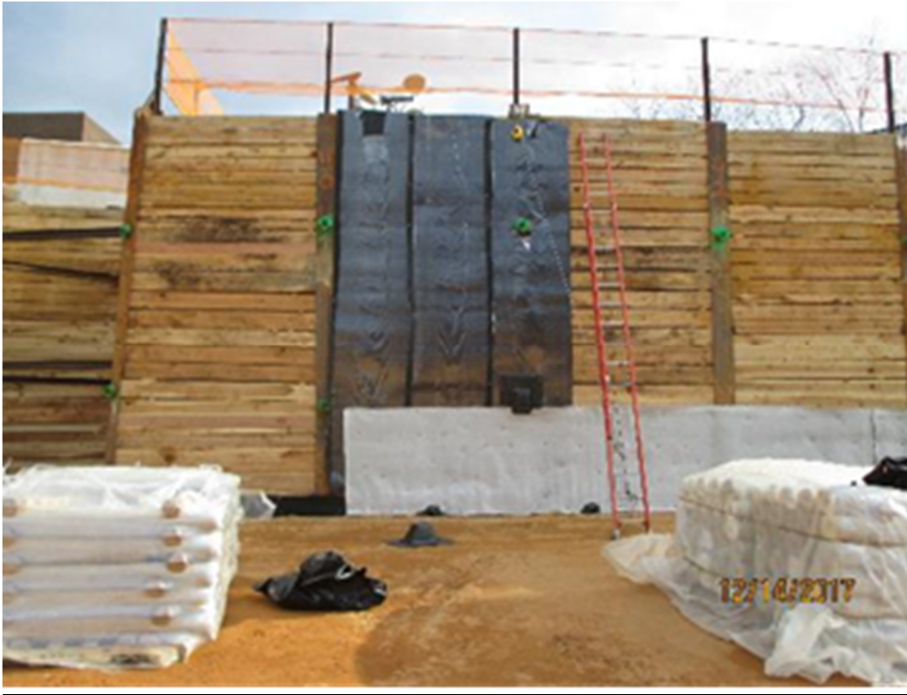
WATERPROOFING OF GARAGE FOUNDATION WALLS
