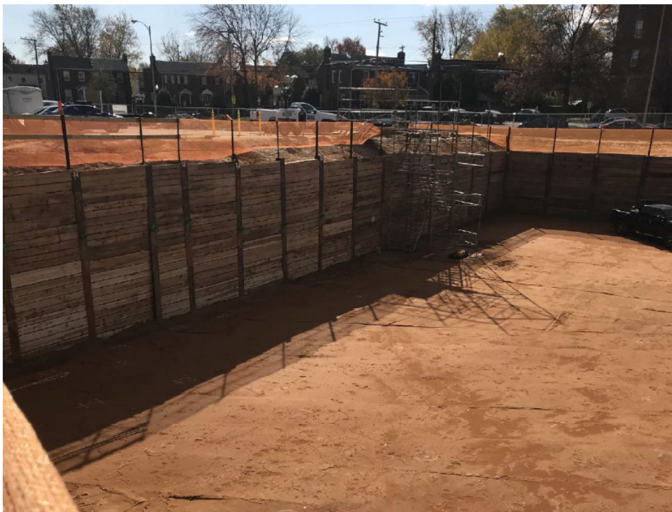
TEMPORARY STAIR FOR ACCESS TO GARAGE EXCAVATION
