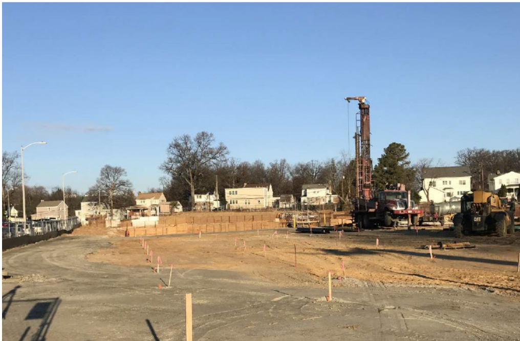
GEOHERMAL WELL DRILLING AT WELL FIELD SOUTH OF GARAGE
