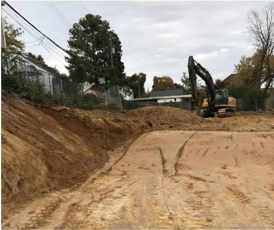
BUS LOOP EXCAVATION
