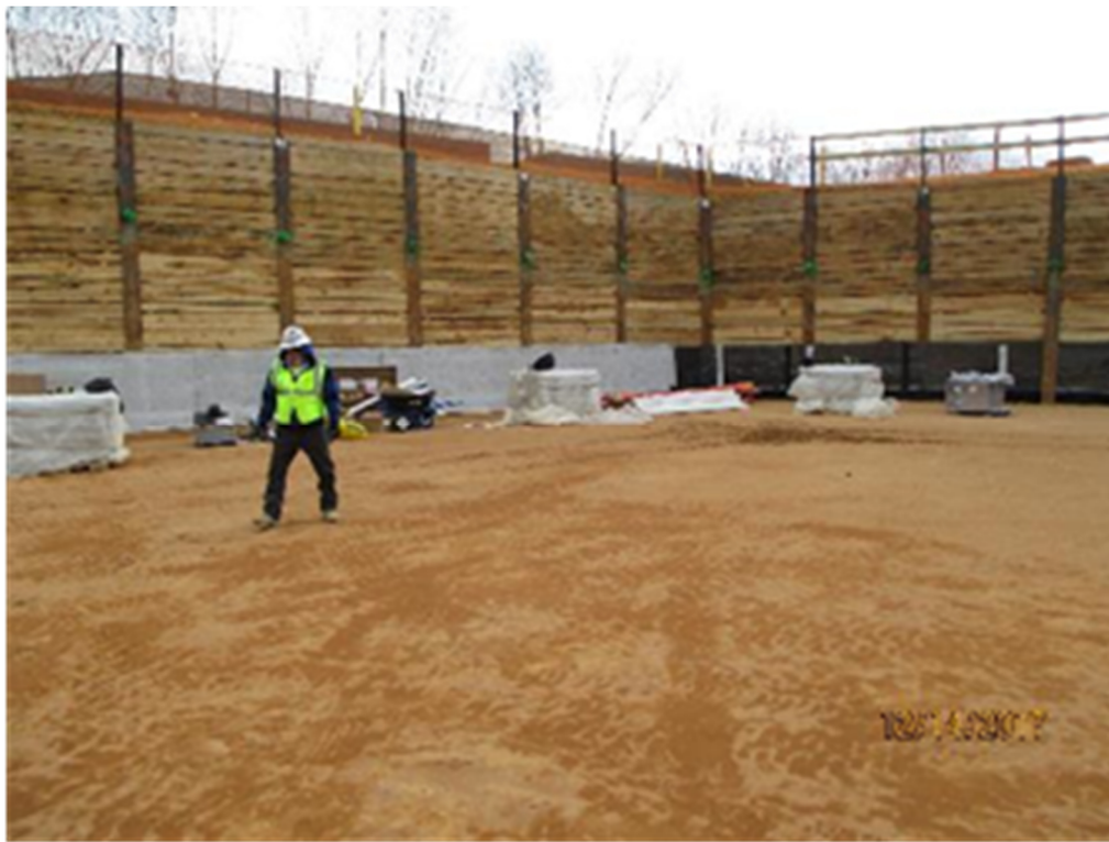
WATERPROOFING OF GARAGE FOUNDATION WALLS
