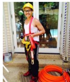
Career Center Student Solar Installation
