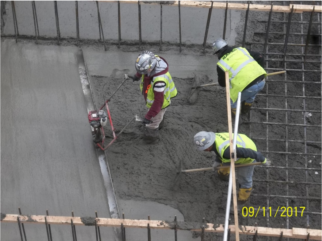
Pouring elevator core footing
