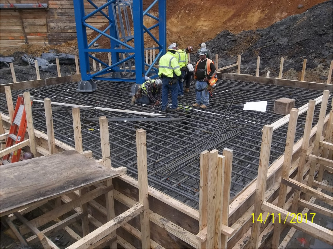
Rebar for crane pad
