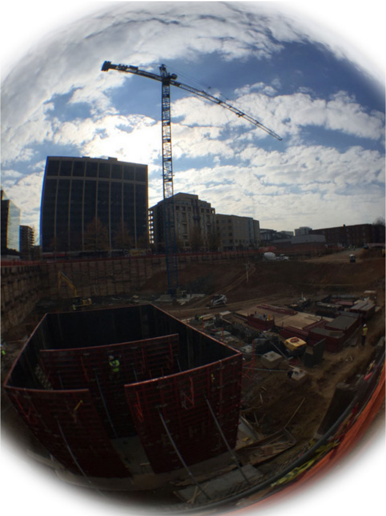
Erected tower crane and elevator shaft framing
