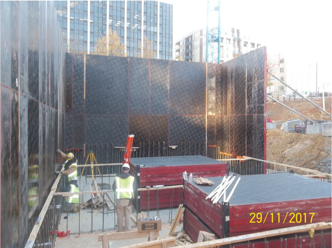
Elevator core concrete wall formwork
