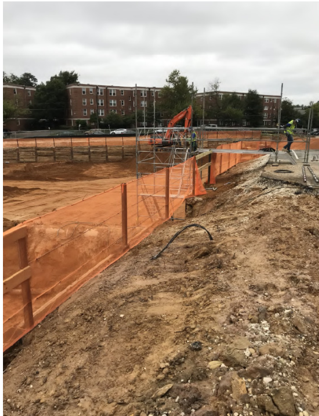
TEMPORARY STAIR FOR ACCESS TO GARAGE EXCAVATION
