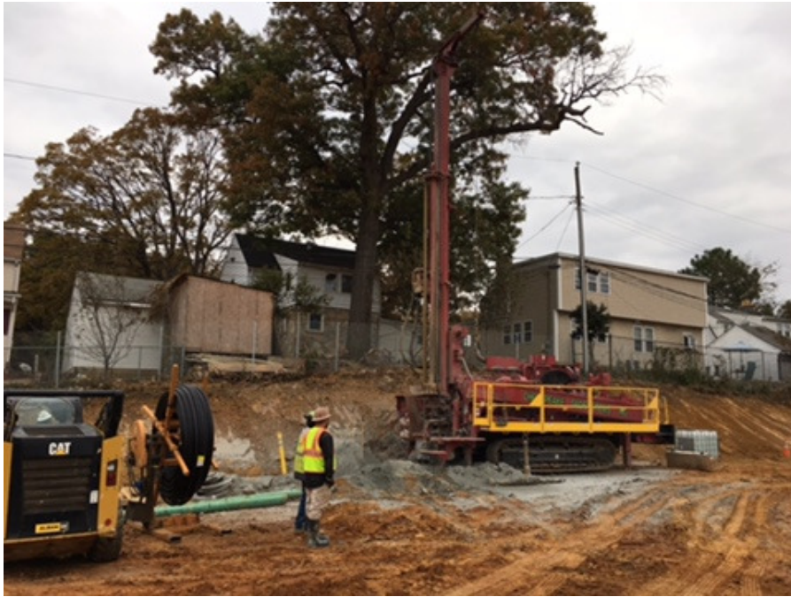
GEOTHERMAL WELL DRILLING
