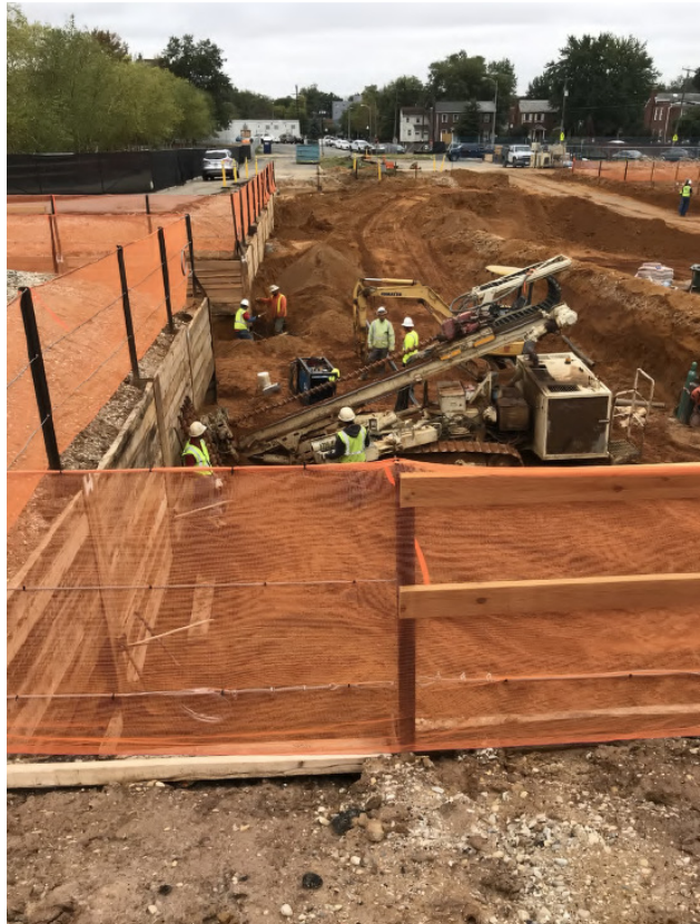
DRILLING OF TIE-BACKS FOR SUPPORT OF EXCAVATION PILES
