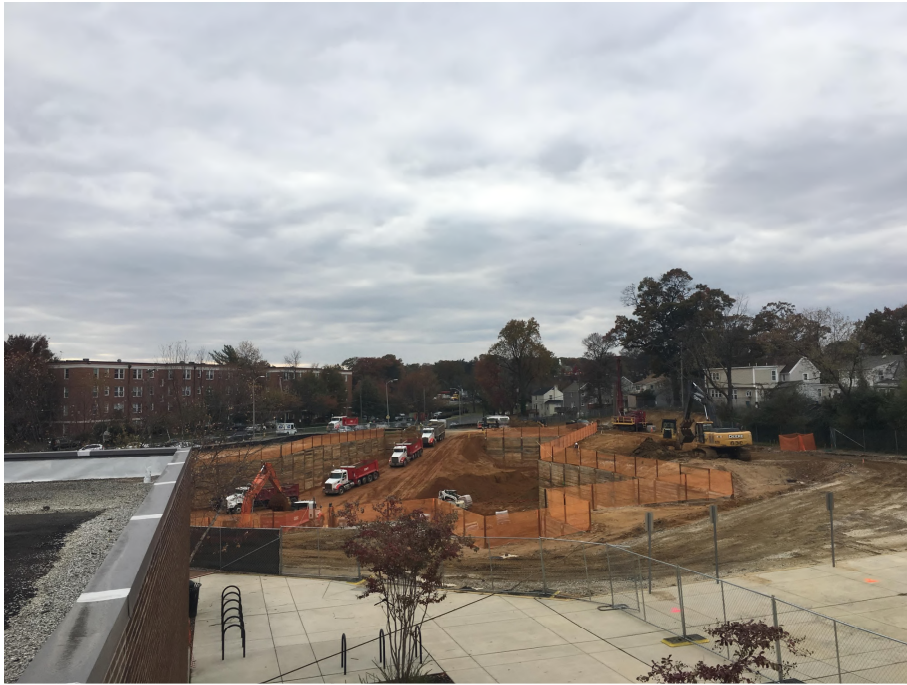
GARAGE AND BUS LOOP EXCAVATION
