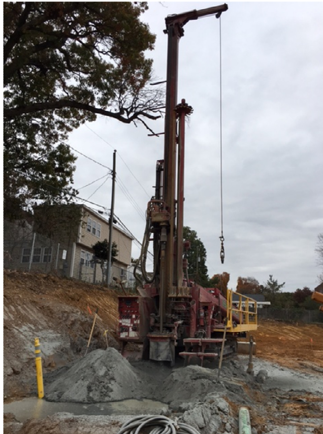
GEOTHERMAL WELL DRILLING
