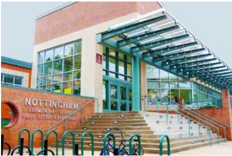
Nottingham Elementary School
