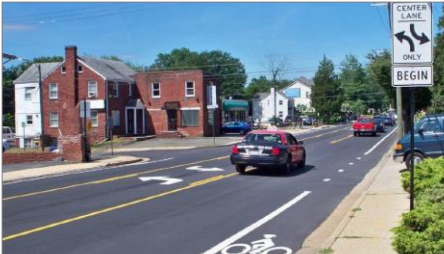
Wilson Boulevard restriping (between Frederick and Manchester Streets)
