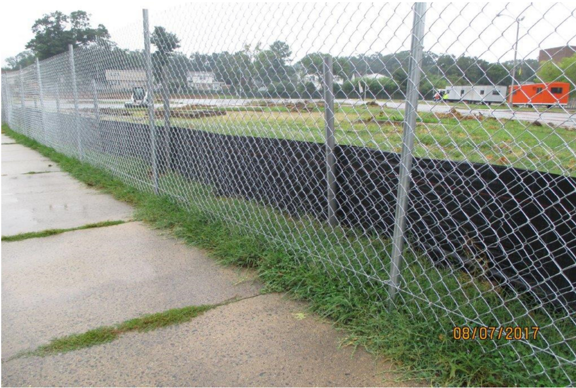
EROSION AND SEDIMENT CONTROLS SILT FENCE
