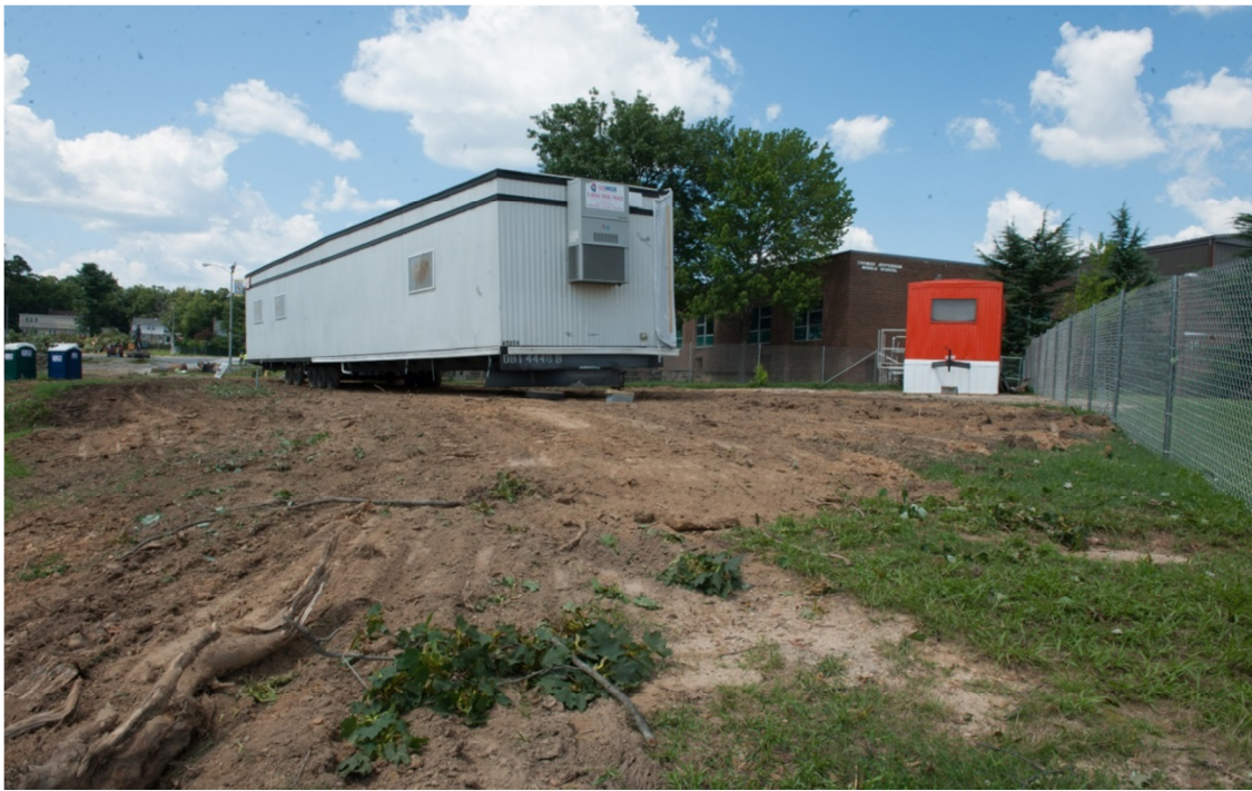
FIELD OFFICES SET UP
