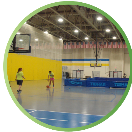
New LED Gymnasium Lighting at Jefferson Middle School and Community Center
