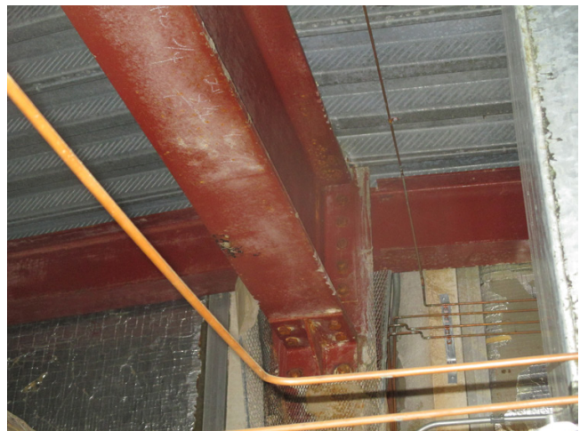
Photo #2: Typical bolted seat angle moment connection
