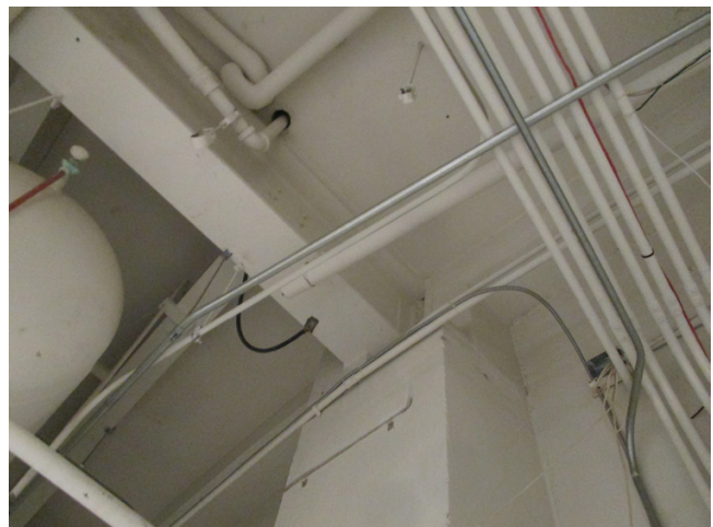
Photo #3: Steel girder to concrete pilaster connection at 1st floor
