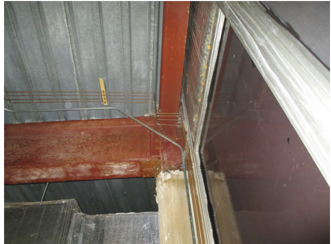
Photo #1: Typical beam-column connection detail
