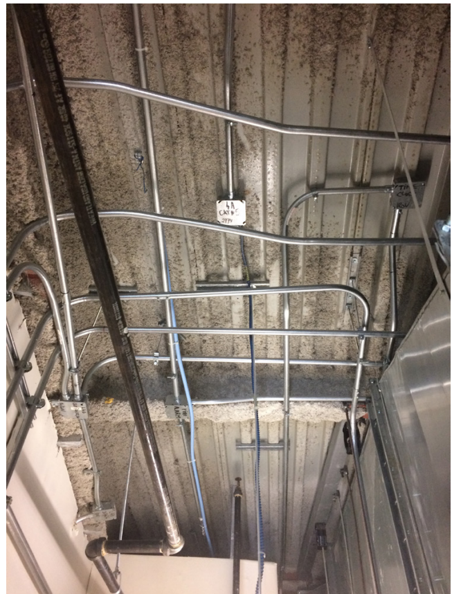
Existing steel structure, floor and roof deck will require spray applied fireproofing
