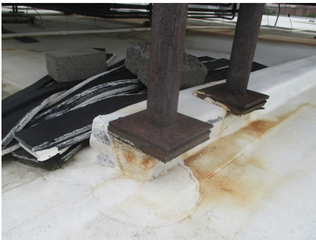
Photo #5: Cantilevered dunnage base plates
