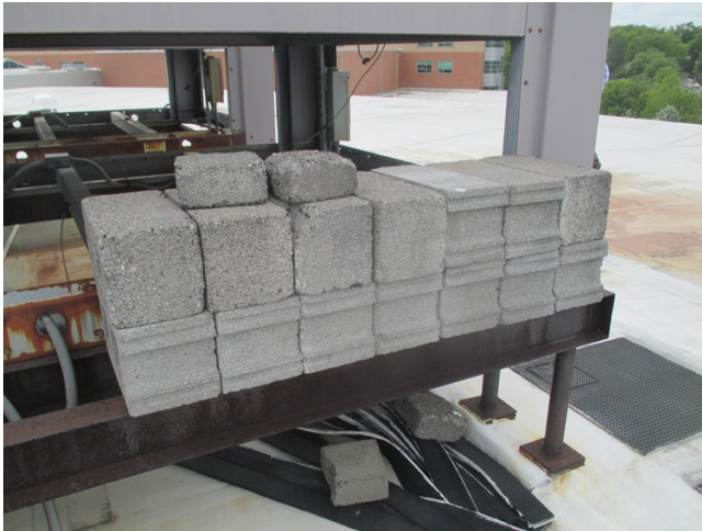
Photo #4: Stacked CMU at top of dunnage beams
