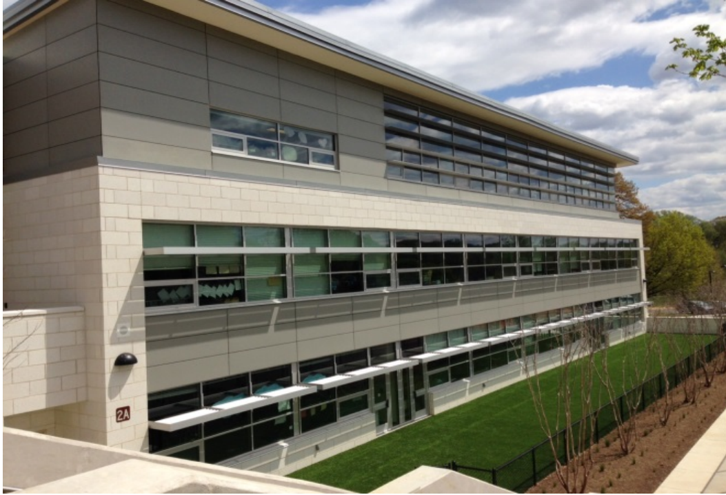
New Wing of the Expanded Ashlawn Elementary School
