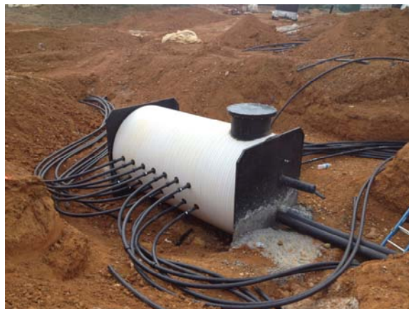
Geothermal Element Being Installed at Wakefield High School Well Field
