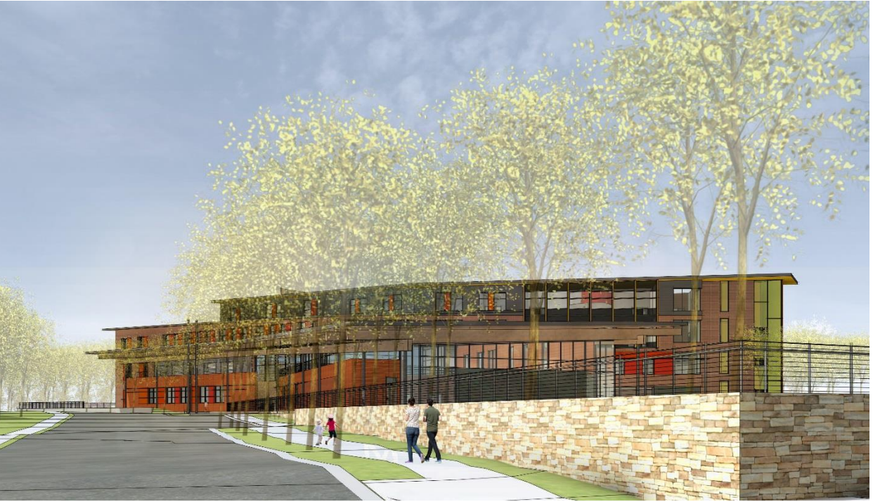
One level parking, partially below grade
