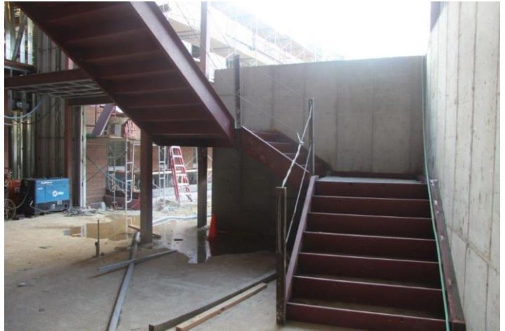
3-Story Interior Stairwell
