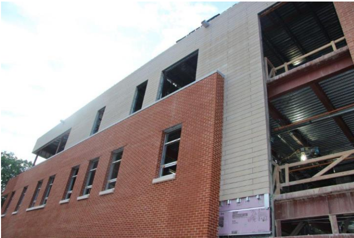
3-Story Addition North View
