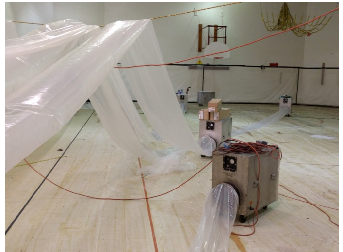
Abatement in gymnasium
