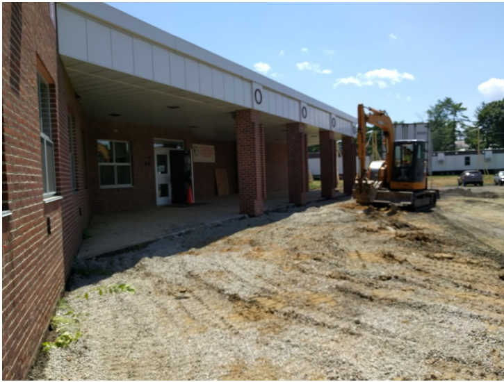
Site demolition at old school entrance
