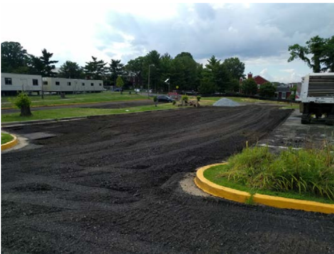
Milling of existing parking lot
