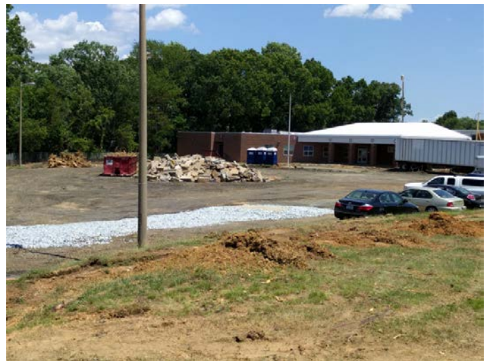
Exiting site demolition complete
