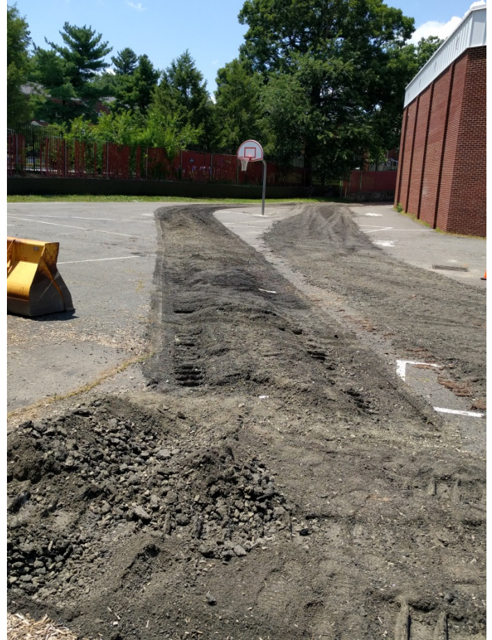
Milling for installation of new electrical service
