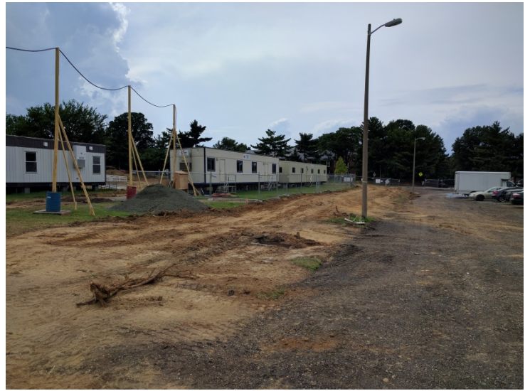
Site demolition at new bus loop
