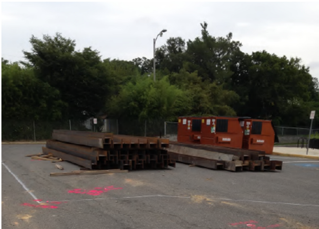
SHORING PILES STACKED AND READY TO BE SET
