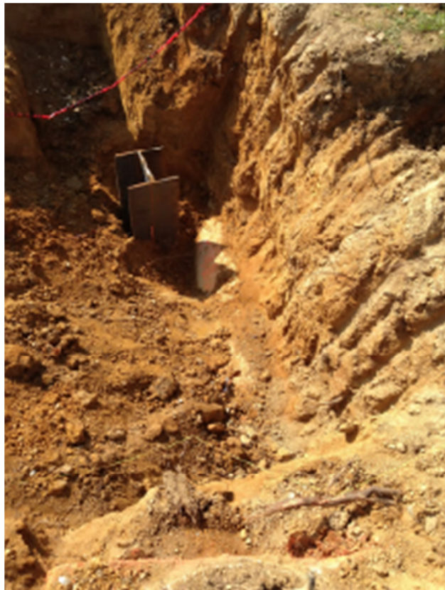
TOP OF A DRIVEN PILE PRIOR TO EXCAVATION
