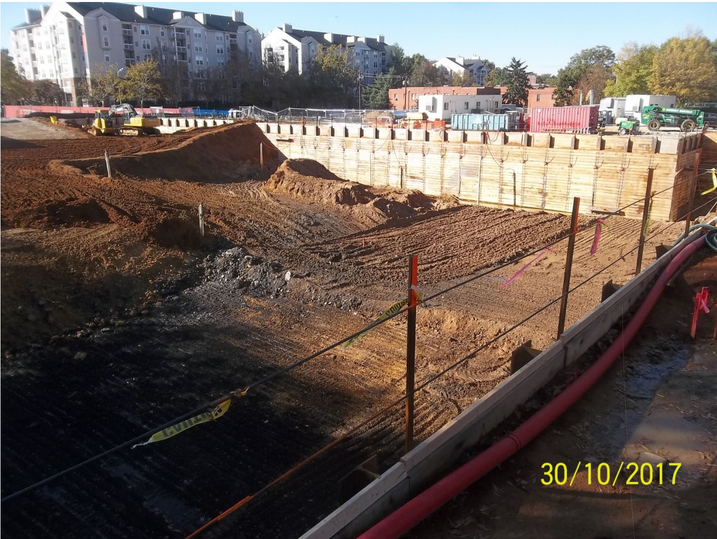
Excavation for concrete pad at elevator tower
