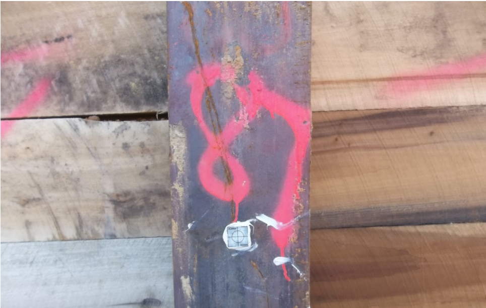
Pile 3D monitoring station
