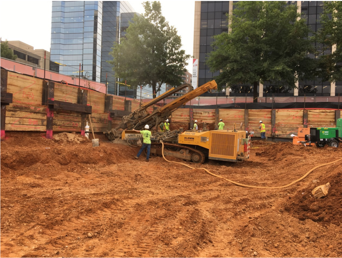
Drilling of tie backs
