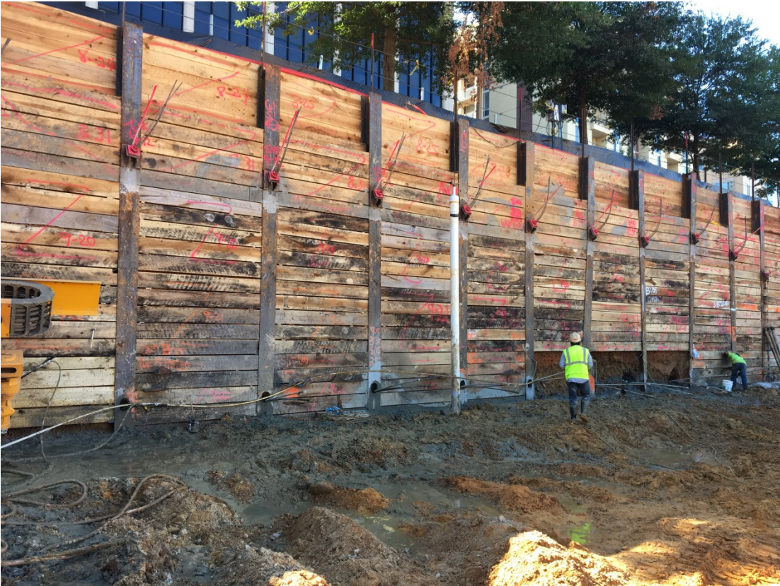
Sheeting and shoring along south side of foundation (Wilson Blvd)
