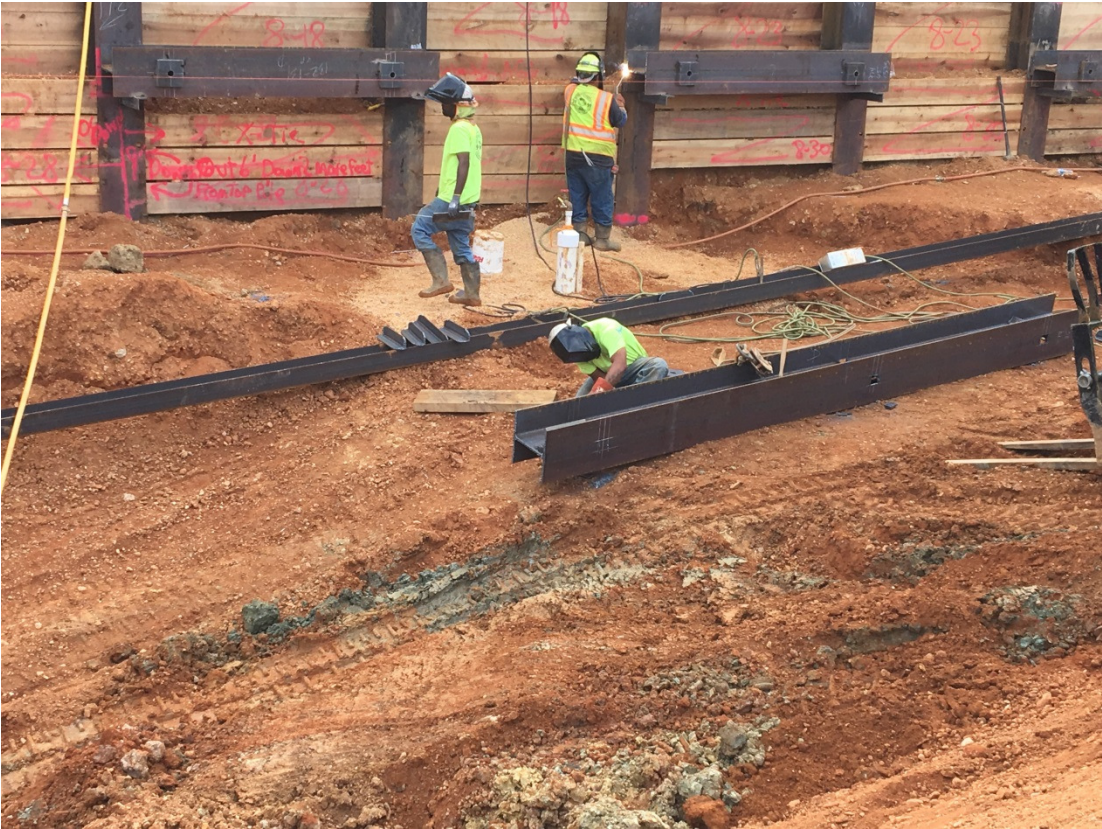
Installation of walers
