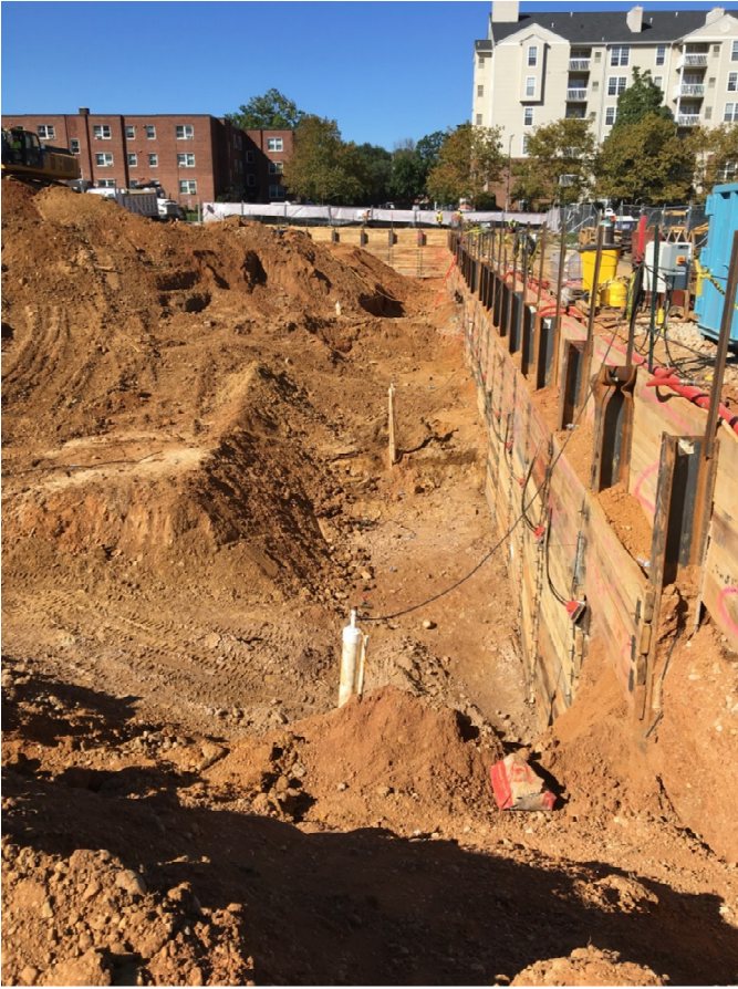
Sheeting and shoring along north side of foundation
