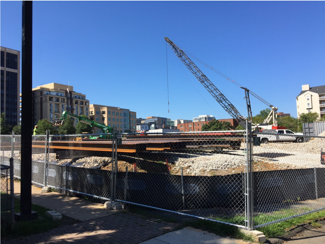
Laydown area for piles
