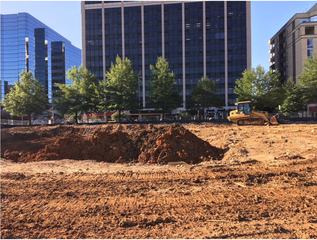
Ongoing site clearing
