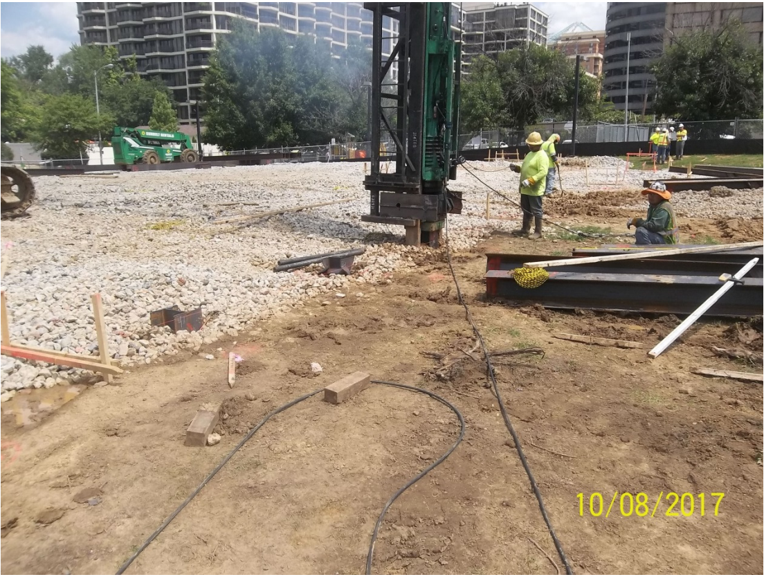
Sheeting and shoring piles to support excavation
