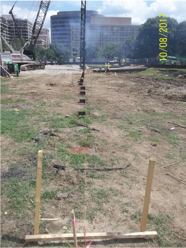
Line of piles
