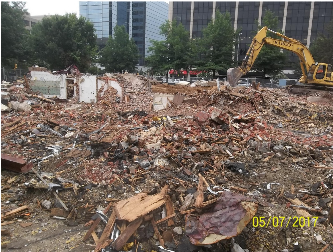
Demo in progress
