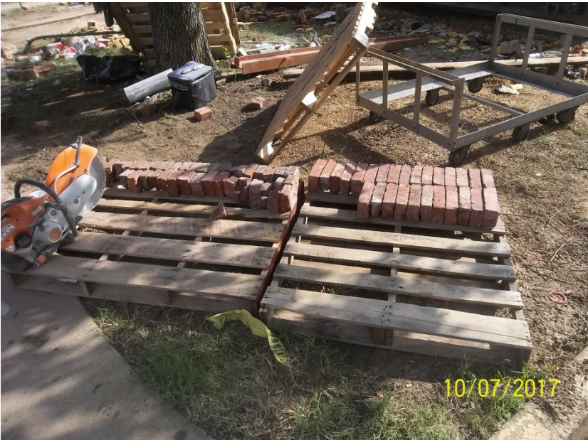
Cleaning salvaged brick
