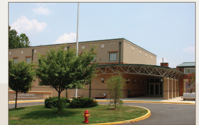
Claremont Elementary School
